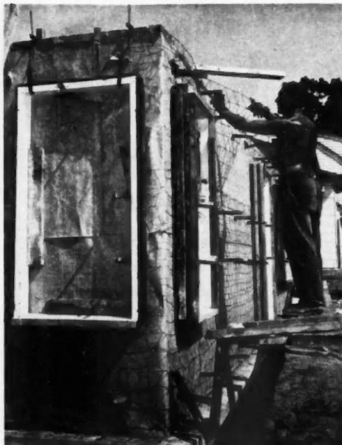
BUILDING paper forms vapor barrier between concrete and furring strips in Pollman system. Window frames held in place with hangers
