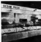
**Wall Covering**—Baltimore Porcelain Steel Corp., Box 928, Baltimore 3, Md. Mirawal is a porcelain-on-steel facing for interior and exterior applications. Has 1/8-inch Masonite backing. Surface is stainproof, fireproof. Application is simple.
