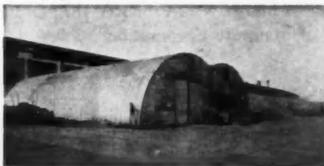
Quonset Multiple and Quonset 40 were chosen by Twin Coach Co., Buffalo, N.Y., to provide additional storage space and experimental manufacturing facilities. Flexibility of design and speedy construction make Quonsets ideal for factory additions.
