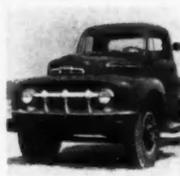
**New Ford Trucks**—Ford Motor Co., Dearborn, Mich., feature automatic Power Pilot carburetion-ignition control, providing economical power by metering and firing correct amount of fuel at right instant. Offers many other improvements.
