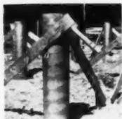
**Column Forms** — Sonoco Products Co., Hartsville, S.C. Sonotubes for forming concrete piers, columns and posts are made in diameters from 3 to 24 inches. Also used for forming ducts in concrete floors, lamp posts. Lightweight, cut by hand saw.
