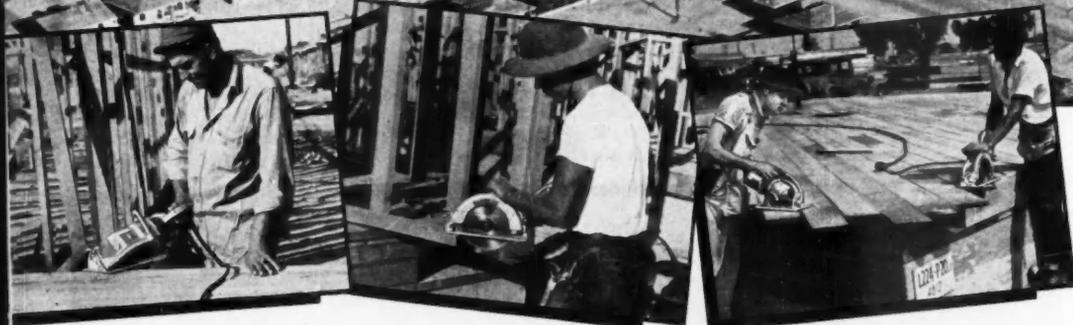
**OVER 171 MILLION FEET OF ROOF LUMBER** will go into Lakewood Park—and SKIL Saws cut all of it. Model 825 SKIL Saw is used in sawing all 2-inch rough lumber for framing members . . . bevel-cutting lumber for jack rafters up to 2½ inches at 45 degrees.
