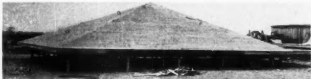
**ROOF OF HOUSE** built complete on jig in assembly yard. Before removal to site roof is cut in four equal panels for easy handling by crane. Note metal rings for hooks
