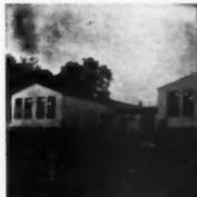
**School Buildings** — Steel-ox buildings are prefabricated by Armco Drainage, Inc., Middletown, Ohio, of patented 18- and 20-gage steel, two to three times heavier than ordinary galvanized roofing. Painting is only maintenance.
