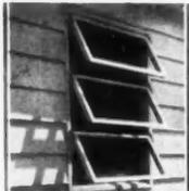
**Awning Window** — Gate City Sash and Door Co., Ft. Lauderdale, Fla. New operating gear enclosure on wood awning window assures smoother lifting and lowering of horizontally opening sash. Available with Thermapane or Twindow.
