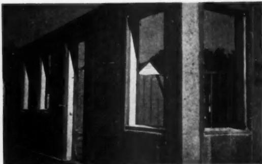
**MORTAR-CEMENT** mix is used to fill small holes where ties are removed
