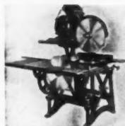
**Portable Woodworking Mill**—The Master Woodworker Mfg. Co., Detroit 26, Mich. Several machines in one, this unit is equipped with overhead cross cut radial saw, knife round head jointer and underslung rip saw. Gas or electric motor.
