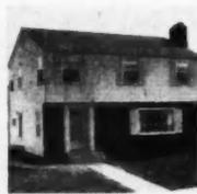
**Building Panel**—Masonite Corp., 111 W. Washington St., Chicago 2, Ill. Tempered Presdwood, all-wood panel, is used as lap siding. Panel comes in widths of 4 feet; is durable and free from grain, knots. Holds paint exceptionally well.
