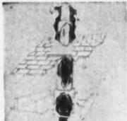
**Packaged Chimney**—Chimney Sales Co., Fredericksburg, Va. Thulman chimney is approved by Underwriters' for use in one, one-and-one-half and two-story buildings and for installation with zero clearance. Unit sent complete.
