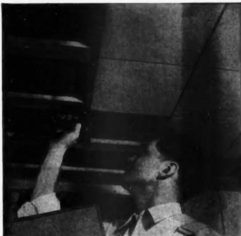
**Temlok Tile** makes old ceilings new. Units are quickly nailed or stapled in place over furring strips. The handy Lok-Bevel joint speeds the job and hides nail-heads or staples from view.
