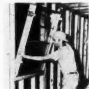
**Packaged Windows**—Fleet of America, Inc., Bladell, N. Y. Fleetlite windows are completely prefabricated, glazed and assembled, arriving on the job in corrugated containers. Extruded aluminum frame, storm sash and screen.
