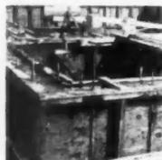
**Concrete Form Tie**—Tie, made by Gates and Sons Inc., 80 S. Galapago, Denver 9, Colo., is a twisted galvanized spreader with loop at each end. Loop goes through form, and a steel rod slides through loop to hold the form in place.
