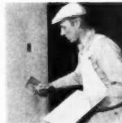
**Bonding Plaster**—Nu-Wall Mfg. Co., 923 N. 19th St., Milwaukee 3, Wis. Used over poured concrete. Applied directly on concrete; no wire lath or base coats needed. Only ¼-inch Nu-Wall coat and ½-inch finish coat required.
