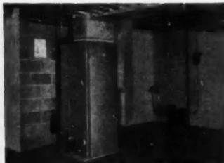
**PENNSYLVANIA** G-E Air-Wall installation in Williamsport, Pa., showing G-E Oil-Fired Unit and extended plenum.
