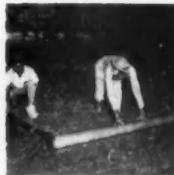
**Waterproof Paper**—Sisalcraft paper in wide rolls is lapped and sealed to serve as waterproof membrane between subfill and concrete slab in basement-less house. The Sisalcraft Co., 205 W. Wacker Dr., Chicago 6, Ill.
