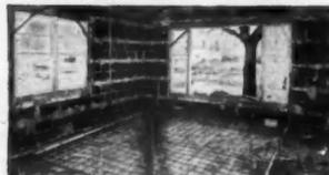
**REINFORCING MESH** in slab and over ducts adds strength to thin part of slab
