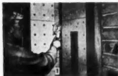
**3 TIMES FASTER THAN HAMMER AND NAILS.** New Bostitch H2B stapling hammer — shown attaching cornerite the quick, easy, low-cost way. Drives staples with  $\frac{1}{4}$ " and  $\frac{3}{8}$ " legs. H2B's drives  $\frac{1}{2}$ " staples.
