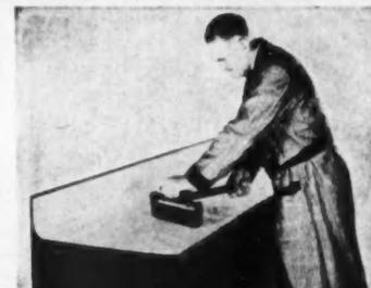
**4** Contact pressure with an ordinary hand roller assures a perfect bond. Note how VERSIBOND can be covered.
