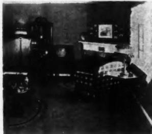
**PLUG-IN baseboard strip allows unlimited placement of furniture and electric devices** distribution panel. Installation of the baseboard electrical trim, which took the place of conventional baseboards,
