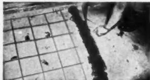
**ALL JOINTS** of waterproof membrane should be lapped and sealed with waterproof sealer
