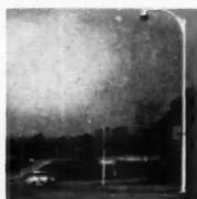
**Aluminum Poles**—Light poles, constructed of Alcoa aluminum alloys by Union Metal Mfg. Co., 1400 Maple Ave., N.E., Canton 5, Ohio, are of tapered octafute design. Bracket arms, bases and fittings are also aluminum.
