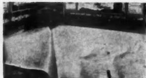
**WATERPROOF** membrane covers the area within foundations and extends on side to slab top
