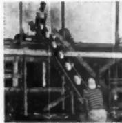
**Brick Conveyor**—Mar-Rail Conveyor Co., 560 York Ave., Pawtucket, R.I. Lightweight Brick-Toter safely handles brick, glazed tile and other materials. Two men can move. Length, 20 feet; width, 14 1/2 inches. Load capacity, over 1200 lbs.
