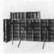
**Steel-Braced Forms**—Symons Clamp and Mfg. Co., 4261 W. Diversey Ave., Chicago 39, Ill. Panels with steel cross members every 12 inches are recommended for heavy pouring. Brace plates can also be furnished for use on 2x4-inch braces.
