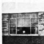
**Residence Steel Casement**—The Steelcraft Mfg. Co., Rossmoyne, Ohio. Made of heavy hot rolled solid steel sections with butt welded mitered corners. Outswinging ventilators provide maximum ventilation, and are easy to operate.
