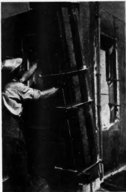
**CORNER** form developed by Pollman can be handled by one man, and adjusted to any angle from 30 to 90 degrees
