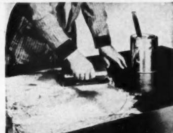
**2** A uniform coating of cement is applied to the rubber backing of a VERSIBOND sheet. Likewise, the underlying surface is also cemented.
