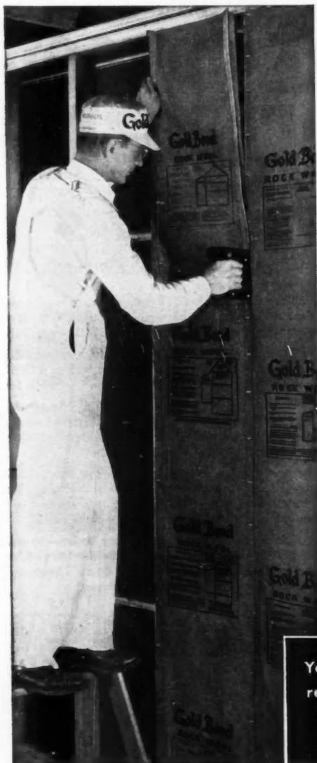
**N**OW you can put top-quality, fireproof insulation into even your lowest-priced homes! Gold Bond's new Mat-Thick Rock Wool Sealed Blankets— $1\frac{1}{2}$  inch thick—cost less than 1-inch thick competitive blankets with lower insulation value. That's about 30% more insulation for your money, and it's fireproof! It will save you \$10 or better on the average 1,000 sq. ft. house.
