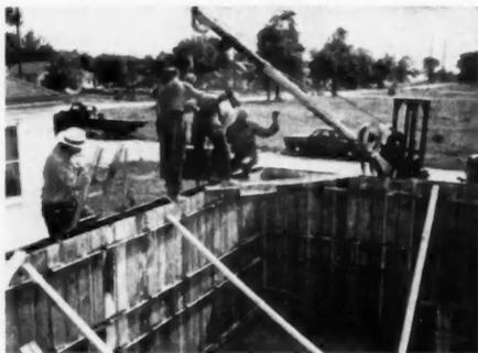
CONCRETE is placed in forms developed by Adam F. Pollman of Milwaukee. Forms are made in 34-inch-wide panels
