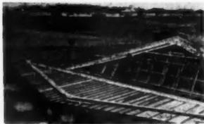
**JIG** for gable ends. Ribbons, gussets set in struts and rafters for added strength
