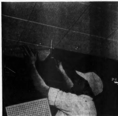
**Cushiontone** stops noise. Units can either be cemented in place or nailed to furring strips spaced 12" on centers. Short-drilled corner holes provide greater nail-holding strength.
