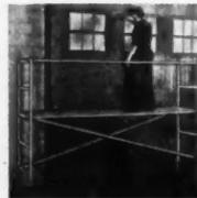
**Aluminum Scaffold**—Ten-foot ladder scaffold is erected from 6-foot, 1-inch ladder sections. Well-suited for locations where working space is limited. Patent Scaffolding Co., Inc., 38-21 12th St., Long Island City 1, N. Y. is the manufacturer.
