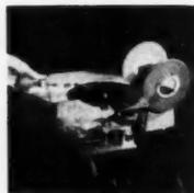
**Sharpening Fixtures** — Treycos Products, 264 Hartford Ave., Buffalo 23, N. Y. Grinder stand with Model 160 base is designed for sharpening saws from 2- to 16-inch diameters. Other available items include saw swage, all-steel saw set.
