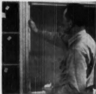
**STARTING** along the side jamb of wood frame, apply a sufficient amount of glazing compound to the perimeter of the back or permanent glazing stop. It is also important to surround the setting blocks with compound but to keep block top clean
