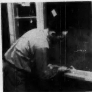
SAME procedure in regard to glazing is followed on the interior except that the application of the glazing compound on the sides of wood sash is finished flat so steel unit is not affected by condensation
