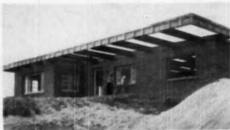
**LIGHTWEIGHT** steel beams form sunshields and porch roof for Ewing home near Corry, Pa., demonstrating design adaptability
