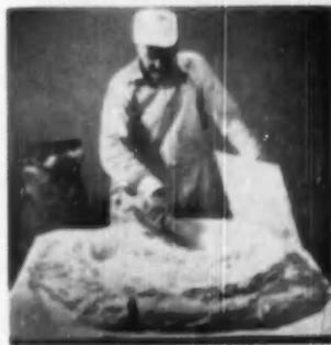
**GYPSUM** quaking plasters bleed easily with lime putty and set before putty shrinks. Ingredients are mixed thoroughly
