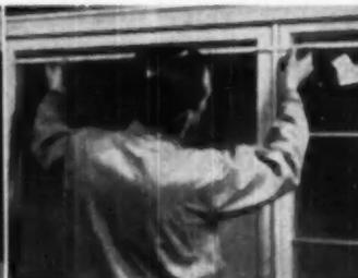
CHECK size of wood sash before installing unit. Opening should be 1/8 inch larger on all sides than the double-glazed unit.
