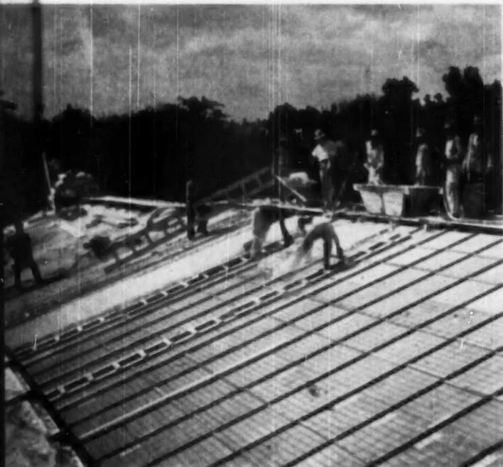
POURED-IN-PLACE gypsum roof decks are adaptable to flat, curved or pitched roofs
