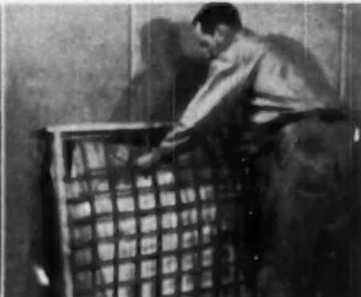
UNIT is protected on the inside by specially developed rigid cardboard web. The unit, with its stainless steel frame, is further protected by a heavy craft paper.
