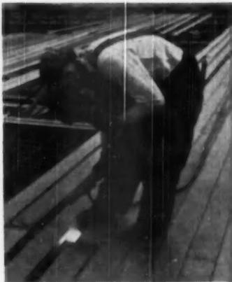
Truscon "Fireboard" Steeldeck with "Clerespan" Joists produces ideal fire-resistant roof.
