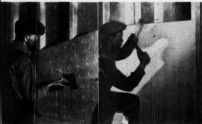
PERFORATED gypsum lath, identical otherwise in all respects to standard lath as shown above, right, allows plaster to "rivet" to lath with mechanical key
