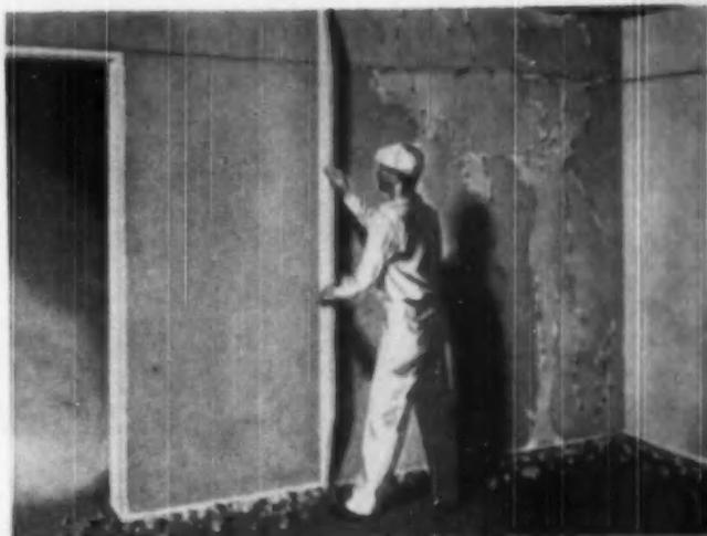
**BODDING** tool is used between grounds or screeds to develop proper thickness and plane
