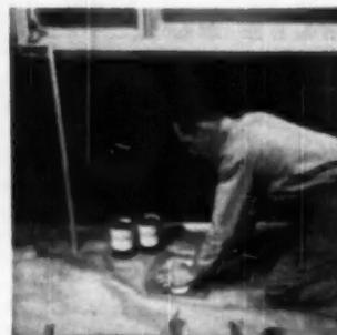
NEXT in importance to a good glazing job is a good glazing compound that has been adequately worked. Putty should never be used as it has a tendency to harden and consequently does not permit the double-glazed unit to "float" in the opening. An elastic glazing compound which retains its resilience permanently is recommended.
