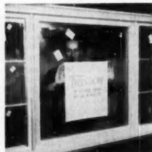
THE Pittsburgh Plate Glass Company's double-glazed unit "Twindow" is all finished. The stainless steel frame has protected it during handling and installation. It will continue to insure the insulating qualities of the unit
