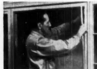
REMOVE exterior glazing stop from factory sash before installing double-glazing.
