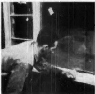
**ADHESION** of the glazing compound helps to hold double-glazing unit in place. However, as a precaution, temporary stops should be placed on top and sides. Next step in glazing is to fill in the voids between the steel frame and the wood opening which is the 1/4 inch clearance allowed for setting
