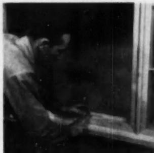
WOOD setting blocks 1/2-inch thick, one inch wide and about three inches long are placed in the position indicated by pencil mark on face of inside stop. A 26-inch sash width is used in this installation, thus the setting blocks are 9 inches in from ends.
