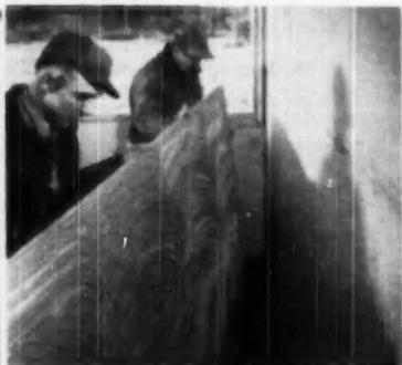
**FACE LAYER** in gypsum double wall system is "buttered" with a special cement
