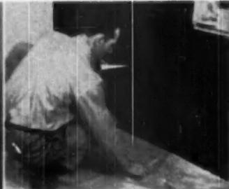
AFTER unit is removed from crate, place on wedges and against wall. This permits steel frame to rest flat against wedges with weight of unit equally distributed.
