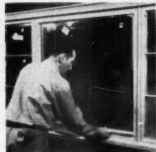
GLAZING stops should be applied carefully. Be especially particular to keep the screws headed vertically and to leave the screw head so the slot is vertical.
