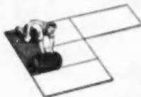
Plywood is ideal for covering old, worn floors to give a smooth new base underlay for linoleum, tile, wall-to-wall carpeting. The big panels go down fast, keep joints to a minimum. There are no humps or ridges to mar finish covering.
