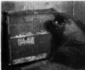
DOUBLE-glazed units are delivered to job in strong crates. First step is to tilt crate at slight angle, placing block in front. Remove one side of crate to start unpacking.
