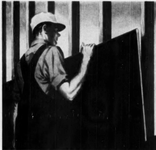
TONGUE-AND-GROOVED gypsum sheathing provides wind-tight walls. Drawing, right
