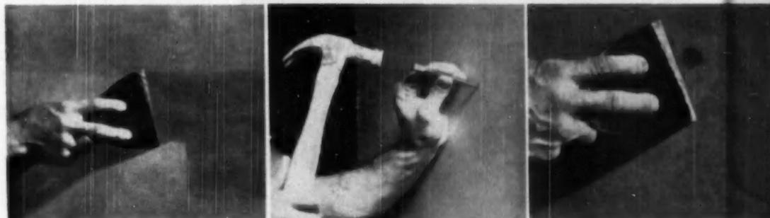
IN FOURTH stage a second coat of cement is applied over imbedded tape, and edges are feathered out, as shown, left. Center illustration shows how nails are "dimpled." Before concealing nailheads, make sure each board is tight against the framing
