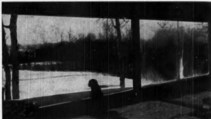
**INSTALLATION** of two types of glass in window wall shown at left was made for the purpose of comparison during period of extreme temperatures. Large unobstructed glass area at left of picture shows an installation of hermetically-sealed double-glazed window. The opening at right is glazed with two lights of single thickness plate glass.
