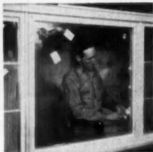
CLOSEUP view of the completed glazing job with the exterior glazing steps removed. Note how the glazing compound on the inside plate extends above the stainless steel channel. Note also how the glazing compound has been packed firmly between metal and sash completely sealing unit from elements
