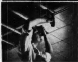
**FOR FAST application, insulating board tiles may be stapled to furring strips**
