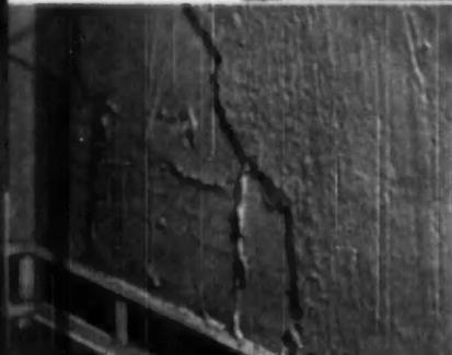
IN TWO-COAT application, cross raking of scratch coat is omitted, as shown above
