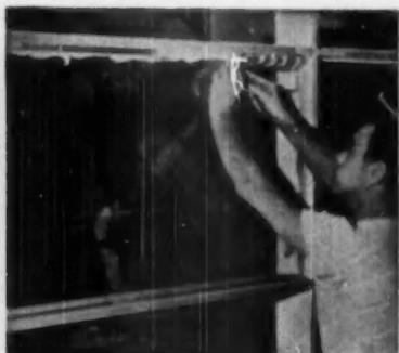
3. *Thermopane* unit in place. Frame has received a bed of glazing compound before insertion of the unit. Workman is filling voids prior to installation of wood stops.
