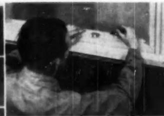
SETTING blocks on sill are placed one quarter of opening width from each end.
