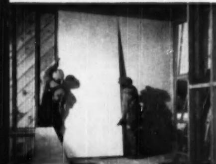
**IN DOUBLE** wallboard installations, first layer of panels is secured vertically
