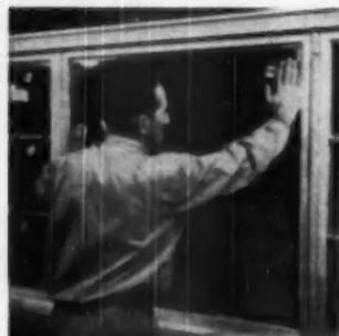
**DOUBLE**-glazed unit is put into place on the setting blocks and gently pushed into position against compound covered stops. Steel frame gives the unit added strength making the handling easier. With slow but firm pressure the steel framed unit is forced inward until all voids are filled
