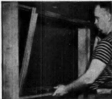
4. Aluminum ventilators of projected type are inserted into openings of wood frame in a bed of glazing compound. Wood screws hold them in place.
