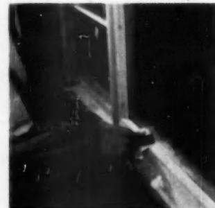
WITH the exterior glazing strips in place the next step is to force the compound and eliminate all the voids. At the bottom of each it is always good judgment to let the compound slant from the glass to the bevelled stop. Be sure that all metal edges are completely covered with compound. This improves the weatherability of glazed unit.
