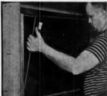
5. Thermopane (standard 42 $\frac{1}{2}$ " x 22 $\frac{1}{2}$ " unit) is installed in aluminum ventilators as in any other face-glazed metal sash. Aluminum screen is installed from inside.
