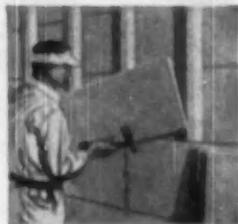
**ROCKLATH®** plaster base, with core of fireproof gypsum, saves plaster, provides a buldog bond. Perforated ROCKLATH offers a mechanical as well as a suction bond, gives greater fire protection. For all-year insulation, plus an efficient vapor barrier, insulating ROCKLATH excels. And, special Long-Length ROCKLATH is ideal in studless non-load bearing partitions and on furred masonry walls.
