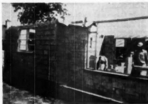
HORIZONTAL joints are accented in exterior wall of "Television House." These joints between concrete block are tooled the entrance is screened from view by a long wall. The architects were Cliff May and Chris Chase.
