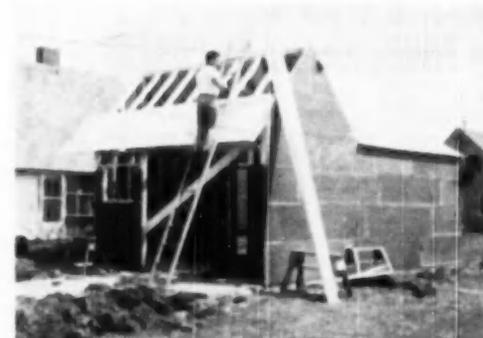
A "BOND-BILT" garage under construction. It is conventionally framed, with 2x4 studs, 16 inches O.C.
