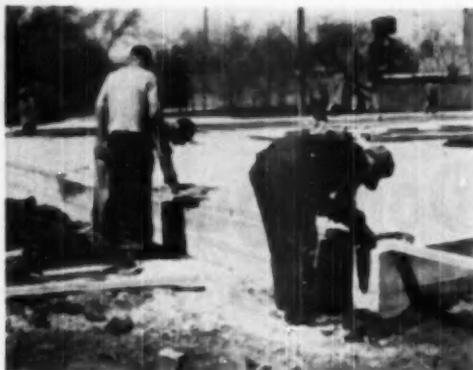
WOLMANIZED pressure-treated wood sill is installed in U. S. Gypsum company's Popular Home magazine's model house at Fair
