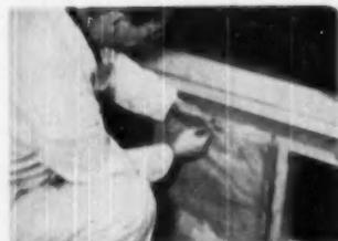
**WHENEVER** batts or blankets butt plates, headers or other framing members, they are cut slightly longer than the space they are to fill. The insulation is pushed back and paper stapled to framing members
