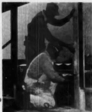
**FACTORY-drilled mullion cover is held in place on a template while electric Impactool drills 5/8-inch into the steel I-beam**
