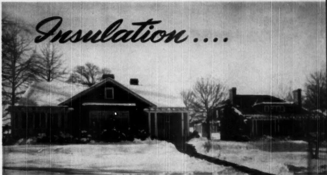
SNOW which disappears quickly from the roof of an uninsulated house is dramatic evidence of tremendous heat loss
