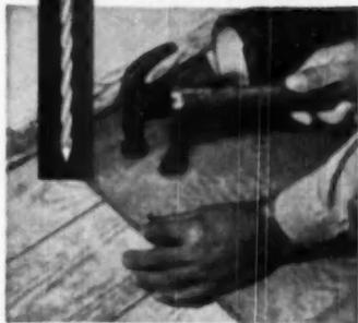
To make your linoleum underlays hold tightly and lay flat permanently, secure them with Hassall linoleum underlay drive screws. They are spiral-threaded and cement-coated for maximum holding power. Heads are flat countersunk type. Size:  $1\frac{1}{4}$ " x #3 ga. State quantity when writing for prices to:
