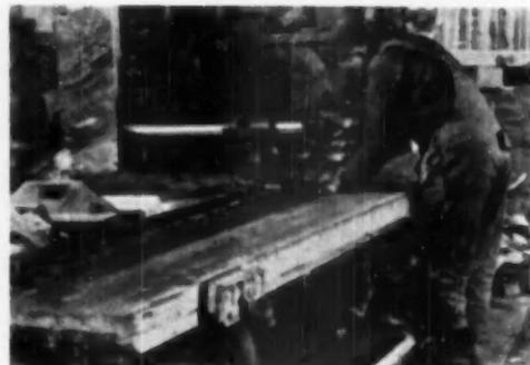
LOW platform of trailer permits use of power saw without climbing. Nuts and other supplies can be locked in trailer at night
