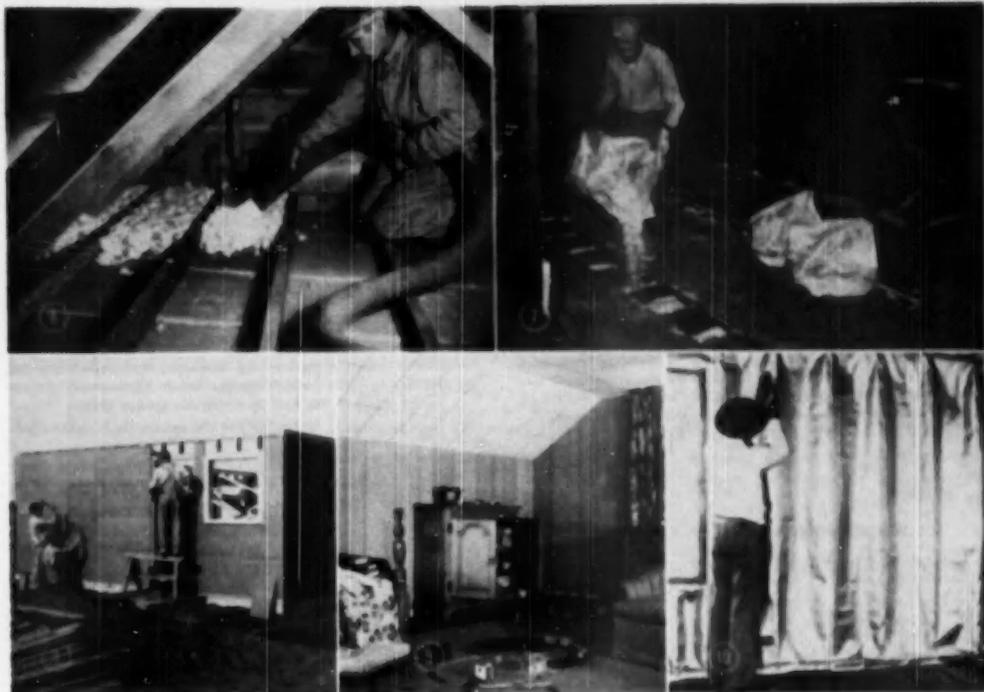
(6) LOOSE fill insulation being blown in; (7) Granular fill insulation being poured; (8) Insulating board sheathing; (9) Decorative insulating board on an interior finish; (10) Reflective insulation. Photos courtesy (6) United States Gypsum Co.; (7) Vermiculite Research Institute; (8) and (9) Insulation Board Institute; (10) The Sianikraft Co.
