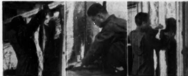
**THIS TYPE** of blanket insulation is compressed for shipment. When installed, it is cut to right length, stapled to the top plate and then stretched to floor plate and stapled there with fiber strips both top and bottom for firm attachment. It is then stapled to sides of studs to provide air space with the reflective foil on the interior, warm side
