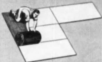
**UNDERLAY** floors for carpeting, linoleum, composition tiles and other modern wall-to-wall coverings must be smooth, firm, solid. Douglas fir plywood answers all requirements. The big panels go down fast with a minimum of sawing, cutting, fitting and nailing. They provide a smooth floor with a minimum of joints—with no ridges or "humps" to mar the beauty of the covering. For underlayment, specify Interior-type Douglas fir plywood—use either PlyPanel or PlyBase grades.
