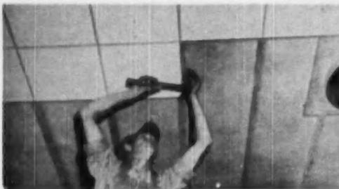
**INSULATING** board tile being applied to furring strips with concealed nailing. It is especially important that framing or furring strips for tile conform to size of units used
