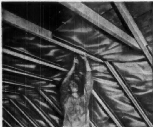
side (Type C) of tough kraft paper. Pressure-embossed in attractive design for extra solidity... clean, pliable, easy to cut and handle.
