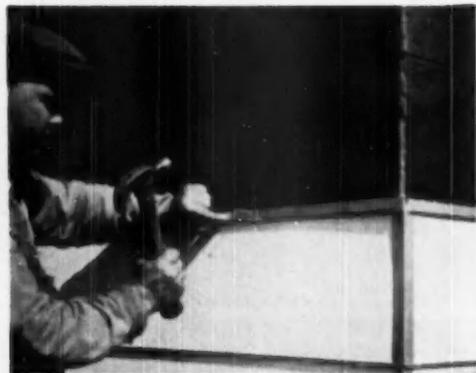
SHADOW lock system of installing shingles is used on Popular Home magazine house sponsored at Fair by United States Gypsum Co. Aluminum channeled strips, corner angles and hook nails are used to obtain deep shadow lines and distinct corners. Wall covering was Glatex, a cement siding, over 1 1/4-inch USG sheathing. Effect of the siding is a deep, attractive shadow line. Insulation was medium thick Red Top insulating wool.
