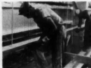
SPECIAL templates are used by members of Jamar-Olman Company's erection crews to mark locations for aluminum-steel studs
