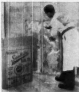
mission. Made in 14 and 24-inch widths, batts have flanged edges for easy installation. Batt is fireproof, moisture-proof, rat-proof and vermin-proof. Units are packaged in substantial cardboard cartons. Seal-Foil Insulation Manufacturing Corp., Dept. AB, Waukesha, Wis.
