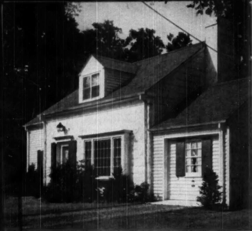
TO HAVE the garage wing conform in outward appearance to the bedroom wing on opposite side of main facade, the surface of the garage door is designed to harmonize by applying horizontal siding to the surface and cutting a window into the door to resemble a wall. Use is made of the same materials for facing the opposite end of front wall
