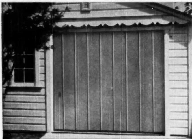
● **LIFETIME PROTECTED AGAINST RUST AND CORROSION** because Glide-Away Doors are made of paint-lock steel which is Bonderized and zinc coated . . . and for **EXTRA** protection they are covered with a prime coat of infra-red-baked paint at the factory.
