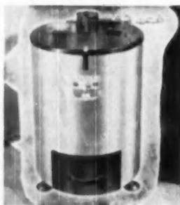
leaving only fine ash automatically swept into large ash drawer. All accessible outside surfaces are insulated with one inch of asbestos. Dimensions are: height-36 inches; diameter-24 inches; A 3/4-inch gas connection and a five-inch flue are required. Autogas Company, Dept. AB, 2153 W. Fullerton Ave., Chicago 47, Ill.
