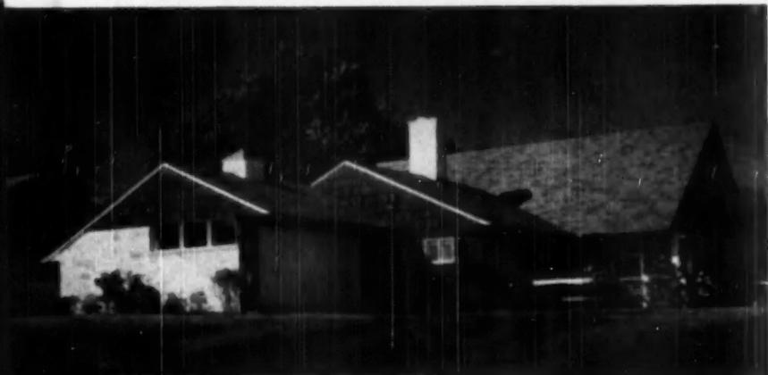
**THIS** position of the eave line in the design of the garage is flexible, as indicated in the house shown at left. It gives an informal appearance to this part of the house. Windows are effectively placed in the street wall of garage, with fieldstone and stained shingles used for the exterior
