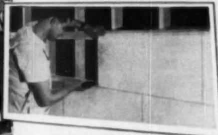
The walls are finished with 16" x 32" Temlok Tile. Tiles are nailed or stapled to furring in new work or can be cemented to old walls in remodeling. Temlok Plank is also ideal for walls, installed vertically or horizontally.
