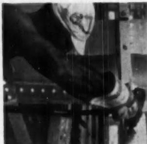
STUDS for siding material are installed before erection of corrugated aluminum
