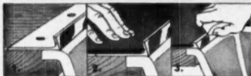
Align CHROMTRIM sink frame over opening. Embed it in Wernco waterproof adhesive and screw down permanently. Frames are pre-drilled with countersunk holes. Use screws supplied.
