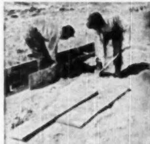
**FIBERGLAS** Slab Edge Insulation being placed around perimeter of Levitt house. 12x48-inch boards are installed vertically
