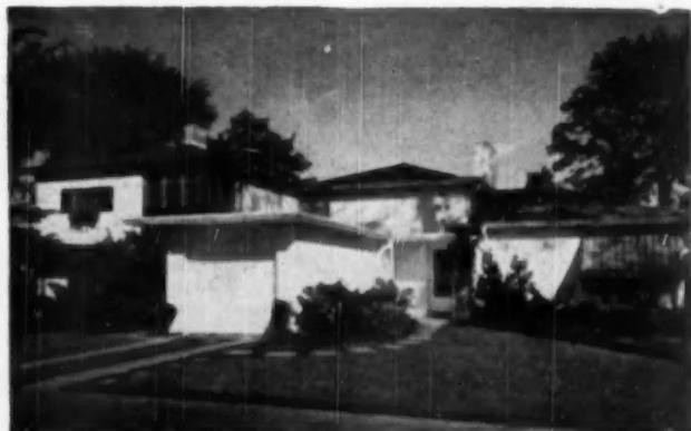
WHERE building codes permit garages are effective when allowed to project beyond the front wall of house. House and garage are of concrete block with flat deck over garage
