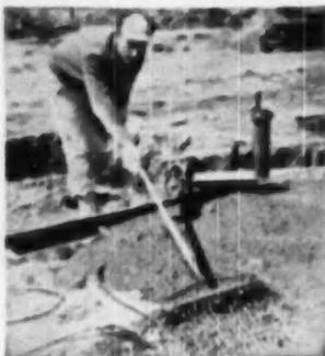
**NEXT** step is to smooth the concrete over insulation and radiant heating coils
