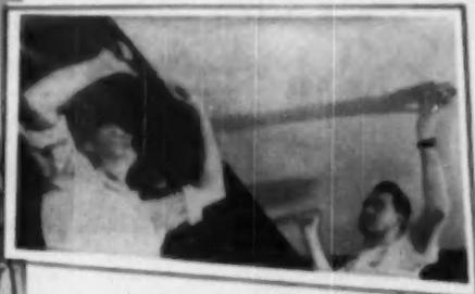
The ceiling is finished with Armstrong's Temlok Insulation Board. These big boards go up fast over furring strips. One piece will cover the entire width of most rooms. False beams hide the joints and add contrasting decoration.
