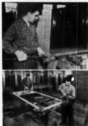
IN CONTRAST to the windows which are shipped "knocked down," combination doors are shipped set up in the large boxes shown above. Below: At dealer's shop combination windows are assembled from proper sizes. Only simple tools are needed for these operations, including the making of screen panels
