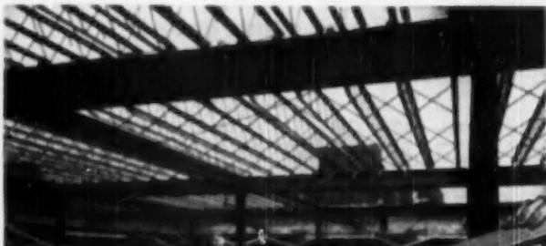
Truscon "O-T" Joists used for Roof Construction
