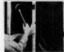
**AB2044**—Upon Roofing fastener. Upon Co., Lockport, N. Y. Fasteners, placed 12 inches O.C. on studs, are called in two pieces. Upon Strong-Bilt full-wall panel is permanently applied to wall of new house by forcing panel against sharp prongs of fastener, which penetrate panel from rear, with block and hammer. BOOTH 118.
