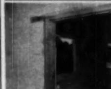
**AB25008**—Steel door frame, The Richmond Fireproof Door Co., Richmond, Ind. Furnished with one pair of steel butts welded to frame as well as a universal strike plate and dust box to receive latch bolt of tubular type lock. Shipped as unit, with proper anchors for type of wall construction to be used.
