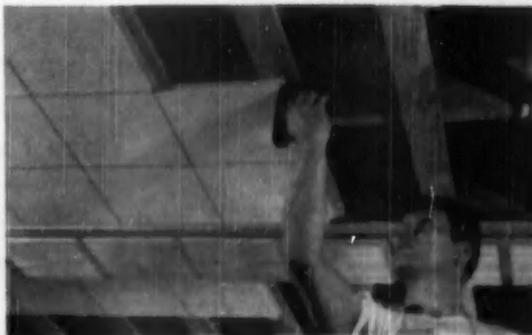
**3.** Quick, easy installation. Temlok Tile comes in three convenient sizes: 12" x 12", 16" x 16", and 16" x 32". Tiles are simply nailed or stapled along furring strips spaced 12" or 16" on centers over ceiling joists. Lok-Bevel joint provides extra-wide nailing flange which speeds nailing or stapling on the job.
