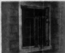
**AR2616**—Triple-Track storm window. Storm Windows of Aluminum, Inc., Marion, Ohio. Means "all-weather" triple track window has especially large glass surface. Has automatic inside lock for added safety. Combines storm cash screen and built-in permanent weatherstrip, eliminating drafts.
