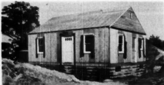
PARTIALLY completed "Fair Deal" paneled house assembled over a full basement. Note plywood sidewalls and roof decking with bevel siding on gable ends. Sidewalls will be completed with wood shingle siding.
