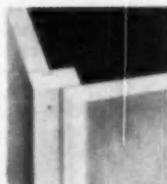
**STRONG CORNERS**—Tongue and groove construction gives extra rigidity, plus a sealed joint against warping and dust infiltration.
