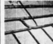
**A82015**—Shresline copper pipe and fittings, Mueller Brass Co., Fort Worth, Mich. In the installation shown above, Shresline copper headers for radiant panel heating are in place, waiting for concrete to be poured. Construction of large warehouse. Both supply and return lines are shown in this photograph. BOOTHS 198, 199.
