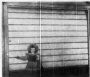
AB250410—Sectional all-steel tilt-up garage door. Morrison Steel Products, Inc., Buffalo, N.Y. Requires five inches of headroom. Factory assembled, ready for installing. Baked-on grey finish. For standard 8 x 7 foot opening. Also 8½ foot opening. Merchandising outlets now being organized.
