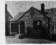
AB2999—Perma-Stone exterior wall finish. Perma-Stone Co., Columbus 11, Ohio. A material end process for casting stone-like facing directly on prepared walls by use of patented moulds. Appearance of natural stone in texture and color. Laid in random, broken, or coursed pattern design. Basic material of this product is Portland cement.
