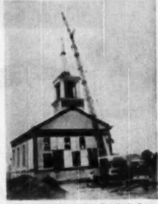
CHURCH is re-erected at Stratford, Conn., after being dismantled and moved 250 miles with the help of MC-416 Lorain crane
