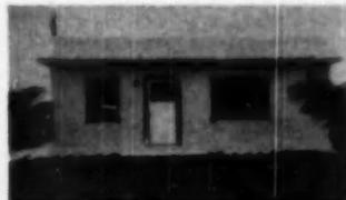
**LOW COST** Florida home rests on concrete slab, has poured concrete walls, partitions
