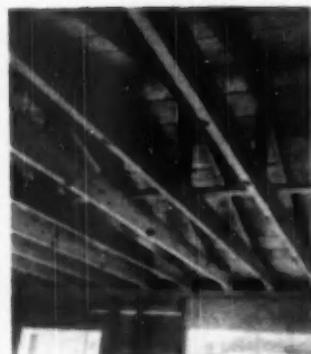
CONSTRUCTION view showing wood roof trusses on wall spaced 18 inches O.C.
