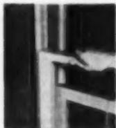
SASH MAY BE REMOVED EASY and quickly without loosening or removing weatherstripping.
