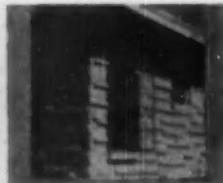
AB25015—New Texas Limestone Texas Quarries, Inc., Austin, Texas. "Roadometer" is split-face limestone in two-course height. Since this stone does not have to be faced at the job site, the firm states that it can be used of cuts comparable to stone siding. Provides attractive exterior for home.
