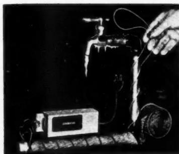
are necessary to install. Length of cable and amount of insulation and wrapping required depend upon length of pipe to be protected. Flexible cable is wrapped around pipe, about one wrap per foot. Insulation, applied, holds cable in place. Waterproof wrap is then applied, and thermostat is mounted adjacent to pipe and plugged into electric outlet. Cable is then plugged into thermostat receptacle, and unit automatically prevents freezing. Gro-Quick Co., 340 W. Huron St., Chicago 10, Ill.
