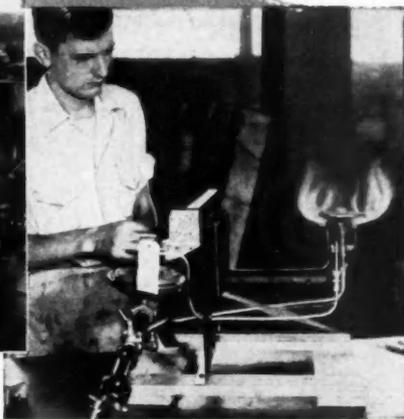
**Paul Simon** is testing the gas burner for the AS23. Each burner, oil or gas, is completely tested and thoroughly checked. They are checked for fuel leaks, electrical connections and control operation. Not until this careful test is completed and passed is a burner released for shipment with the furnace.
