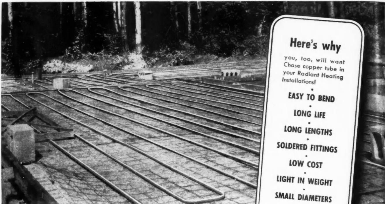
Floor installation of Chase Copper Tube for radiant heating in small home. Long 60- and 100-ft. lengths of tube eliminate many costly connections. Architect: Galloway & Henry, Westfield, N. J. Heating Contractor: T. J. De Chellis, Westfield, N. J.
