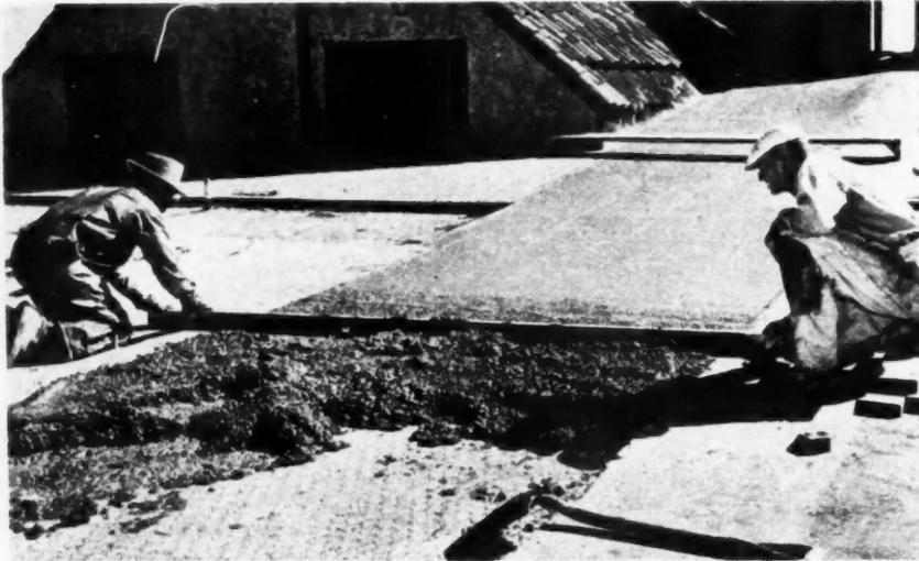
**SCREEDING** perlite-concrete roof deck to 3-inch thickness. Mix of ten parts perlite to one part Portland cement, usually ideal for roof decks, produces monolithic pour weighing about one-quarter as much as sand concrete with about 12 times the insulating value
