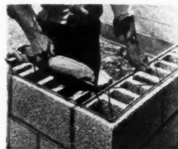
in mortar, it forms continuous lateral reinforcing to prevent cracks. Used as reinforcing to tie face brick to back up block, in double wall construction, where insulating dead-air space is formed; for brick and clay tile wall, as well as for reinforcing block walls. Dur-O-Wal Div. of Cedar Rapids Block Co., 656 12th Ave., S. W., Cedar Rapids, Ia.
