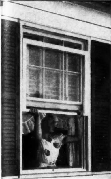
The top storm section slides into position on metal guide strips attached to sides of window frame. Positioning clips hold storm section firmly in top position.
