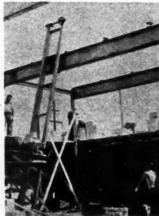
tor moves on wood track which is built by contractor on job site with standard size 2x6 lumber. Steel channel, with all joints electrically welded, provides sturdiness to elevator platform. System may be used in conjunction with any power hoist capable of exerting 400 pound effort on a single line. King Manufacturing Corp., 3146 W. Chicago Ave., Chicago 22, Ill.
