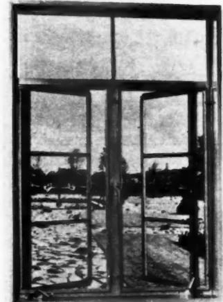
Suitable for all residential construction, frame, masonry or brick veneer. Stool, head and jamb sections formed from 18-gauge steel, bonderized and primed. Easily assembled by steel tenons, which are extensions of head and sill members inserted in slots in jambs and bent into holding position. Angle fin provided, if necessary for structural requirements. Hope's Windows, Inc., Jamestown, N. Y.
