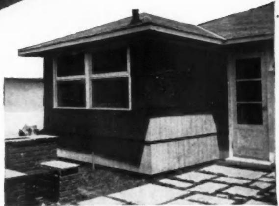
WELDTEX SIDING can be used over any type sheathing. Fits perfectly on 16" studding. Photo above shows the pleasing effect obtained by using a wood lath to create a deep shadow line. Weldtex Siding is made of 3-ply Weldtex plywood, Exterior Grade,  $\frac{3}{8}$ " thick, pre-cut in panels 48" wide, 15 $\frac{7}{8}$ " deep. Packed 20 panels per bundle (1 square).
