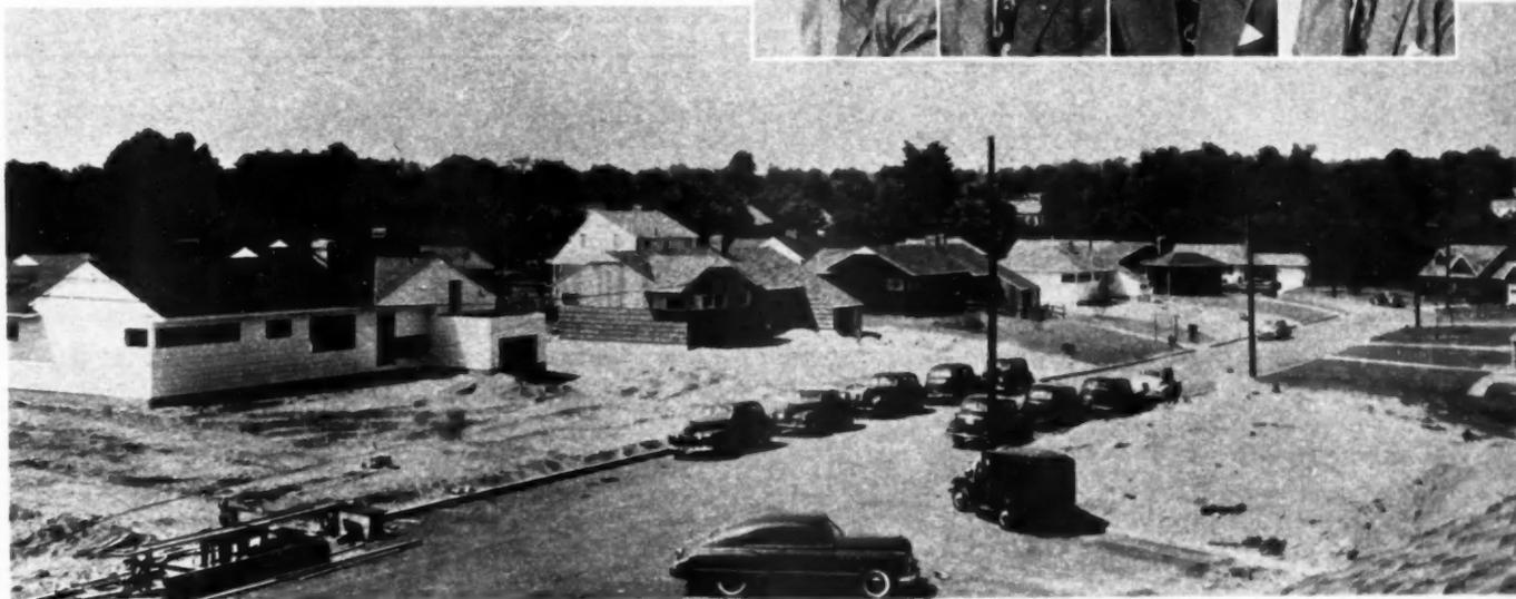
**GENERAL view of houses under construction. One of the radial arm saws used to cut lumber at the site is in left foreground**
