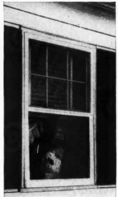
The bottom storm section and the screen section are supplied with pull handles for easy handling and are held in place by coil spring and finger pull. May be locked by hook on sill.
