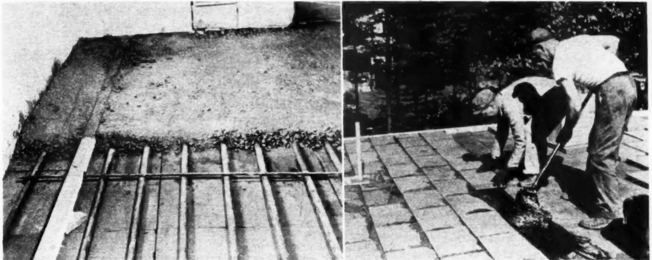
POURING concrete slab over radiant heating pipes (left) which rest on a layer of glass insulating material laid on the ground. At right, workmen mop the glass material to a flat roof deck. The insulation may be laid with the standard types of hot bitumens
