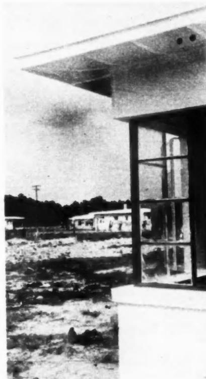
**POURED** concrete lintel supports corner of roof above this corner window of home in Burkrete subdivision. Remainder of exterior walls are of concrete blocks
