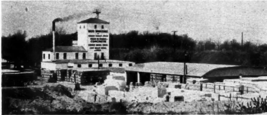
**CAPACITY** of Hass cement block and brick plant is 5,000 8x8x16 blocks per eight-hour working day. A mix-in-transit concrete service, which company operates in conjunction with plant, right, is the only one of its kind in the South Bend area.
