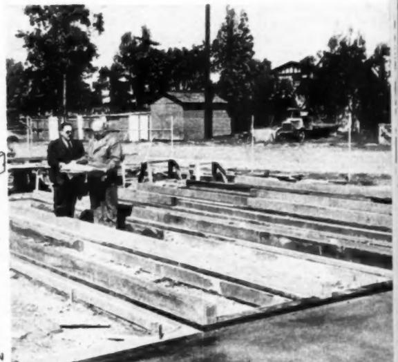
IDEAL treatment of balloon frame and California-type structures is shown in drawings, left. The 4x6 girders in illustration are treated with a moisture resistant preservative that, in addition to repelling termites and fungi, offers dimensional stability
