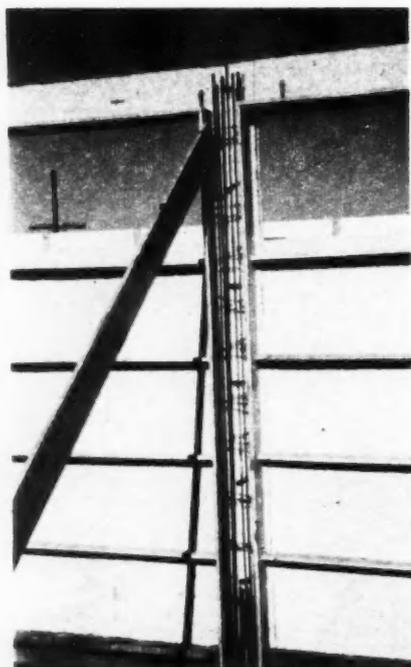
**EXTERIOR** view of present gypsum wall set up ready for application of exterior precast reinforced concrete slabs. Note steel set up in column ready for pour
