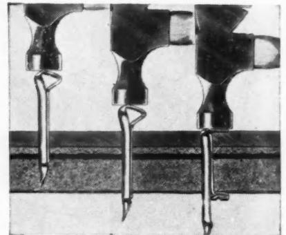
CROSS section illustrating the locking action of ES-nails. Maximum holding power is obtained when locking foot opens immediately behind gypsum sheathing or deep within insulating sheathing board
