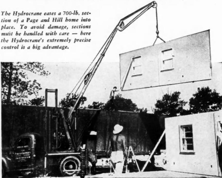
A TRUCK-MOUNTED Bucyrus-Erie Hydrocrane has cut the time for unloading and erecting pre-fabricated homes from 6 or 7 hrs. down to only 2½ hrs. — that is the experience of Petroleum Equipment Co., Milwaukee, Wis., sub-contractor erecting Page and Hill homes. Previously, a motor transport tractor equipped with chain hoist hauled sections from trailer to foundation. The tractor couldn't operate on uneven ground, and much of the heavy work still had to be done by hand.
