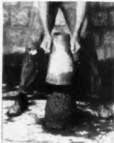
Lifting the slump cone in a typical test for the consistency of concrete.
