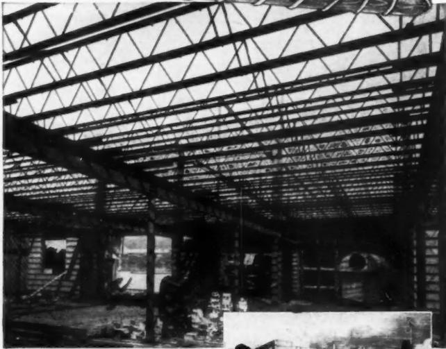
Ritenour High School in St. Louis County, Mo., shown under construction using Laclede Steel Joists. Architect: Wm. B. Ittner, Inc. Contractor: Lecoutour Const. Co. Architect's sketch at right.
