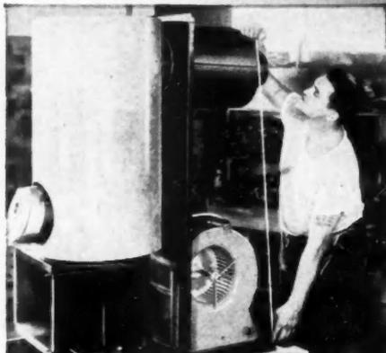
**Robert Kleiman**, a line inspector, supervises the assembly of the various parts of the heating unit. He makes sure each element is in its proper position and thoroughly secured in place. For years Kleiman has been on the line—checking his assemblies—and passing them on for enamel jackets.
