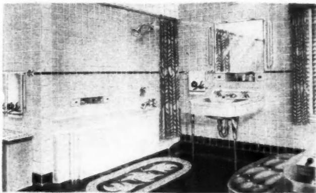
*the new featherweight wall tile, fabricated of sturdy aircraft aluminum, finished in lustrous enamel permanently bonded to the metal.*
