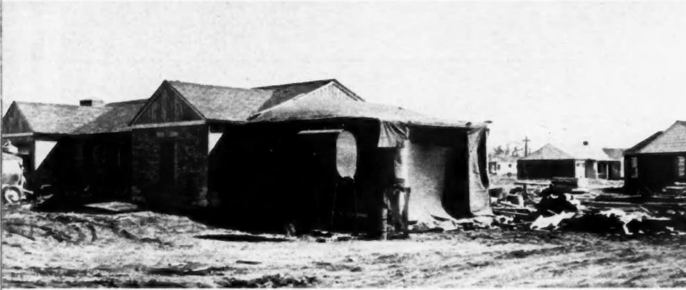
**PARTIALLY** finished house centrally located on site provides space for precutting equipment and storage. Lumber is stored under temporary tarpaulin roof until cut
