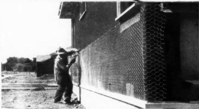
The use of Keymesh Reinforcing speeds up construction because of its ease of application.
