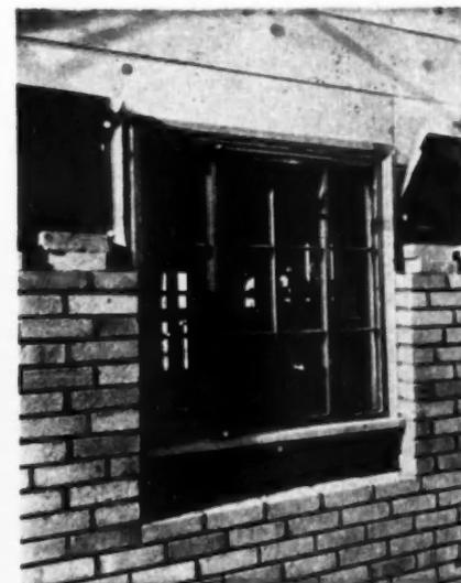
**TYPICAL** brick veneer wall under construction. This type wall is preferred by many builders because of its flexibility and the variation in design that is offered
