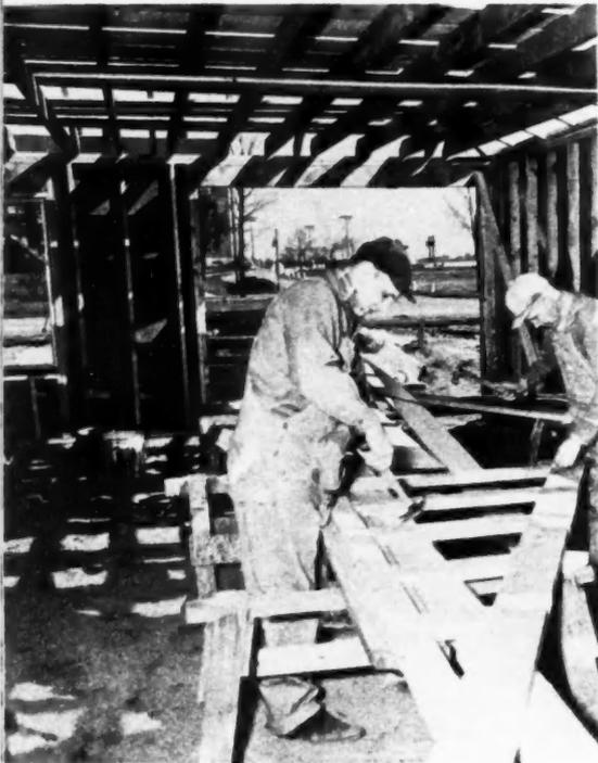
**GABLE** ends are assembled on horses before being hoisted and put into place
