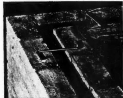
**CAVITY** brick wall in process of being built. Two rows of brick are separated by a wide air space. Metal anchors placed in joint at every sixth course bond the two walls. Care must be used in building
