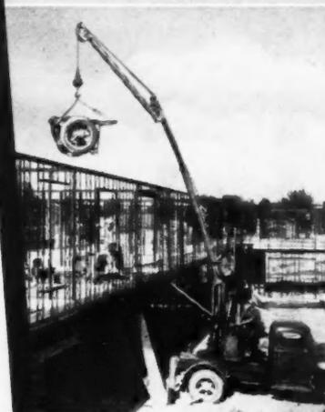
Hoisting concrete buggies is another quick, easy job for the Hydrocrane. Operation is simple — hand levers only, no foot controls.
