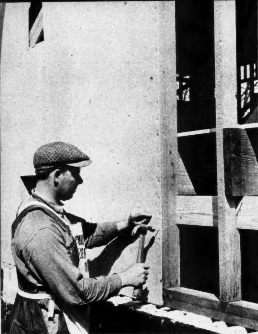
METHOD of applying insulating board sheathing to exterior wall
