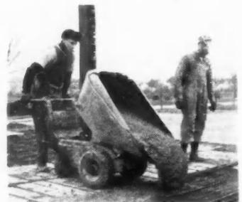
foot pedal. Equipped with a 9 square-foot steel platform, it hauls half-ton loads. Powered by enclosed engine, climbs 20 per cent grade fully loaded. Three gallons of fuel provide 8 hours' continuous service Bell Aircraft Corp., P.O. Box 1AB3, Buffalo 5, N.Y.
