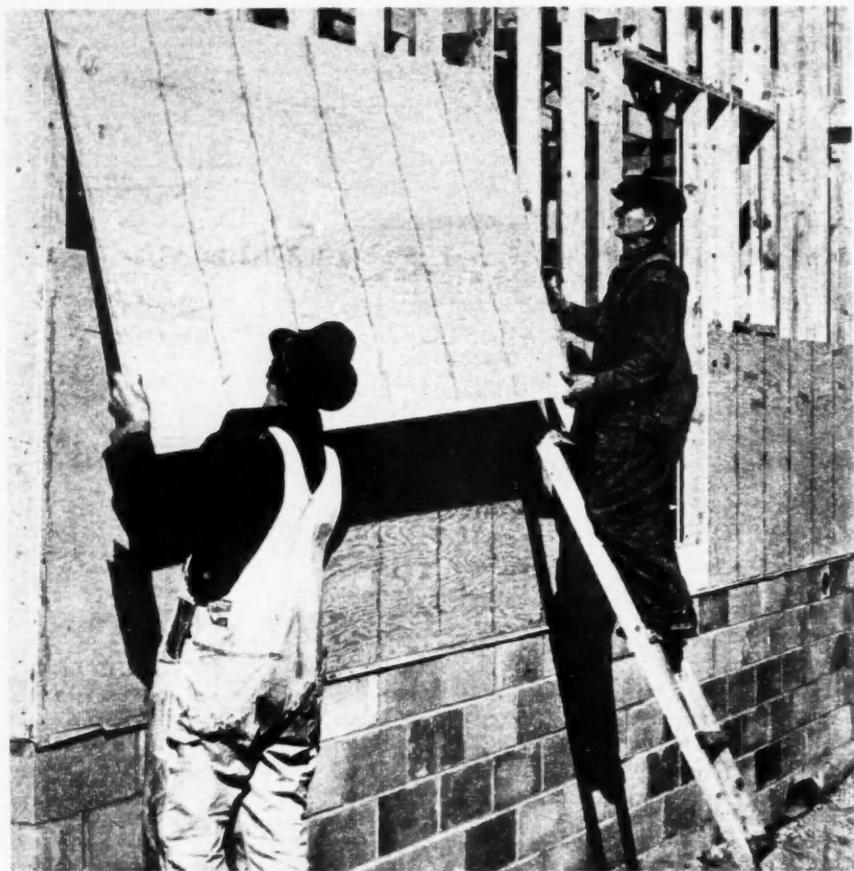
SCORED plywood veneer applied to outside face of studs provides rigidity to walls
