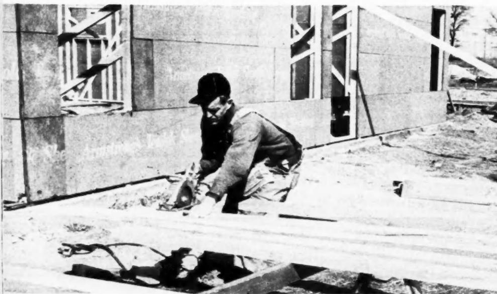
**EIGHT**-inch blade Skilsaw is used to make angle cuts on rafters at site
