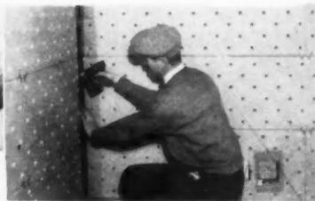
**How to Speed up Tacking.** This Bostitch T5 Gun Tacker shoots staples in . . . within 1/16" of corners, closer than any other tacker. A time-saver for applying insulation, metal lath over joints and corners . . . a cost cutter on dozens of jobs.
