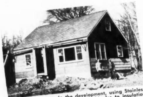
One of the houses in the development, using Stainless Steel ES-nails to apply asbestos shingles to insulation sheathing.
