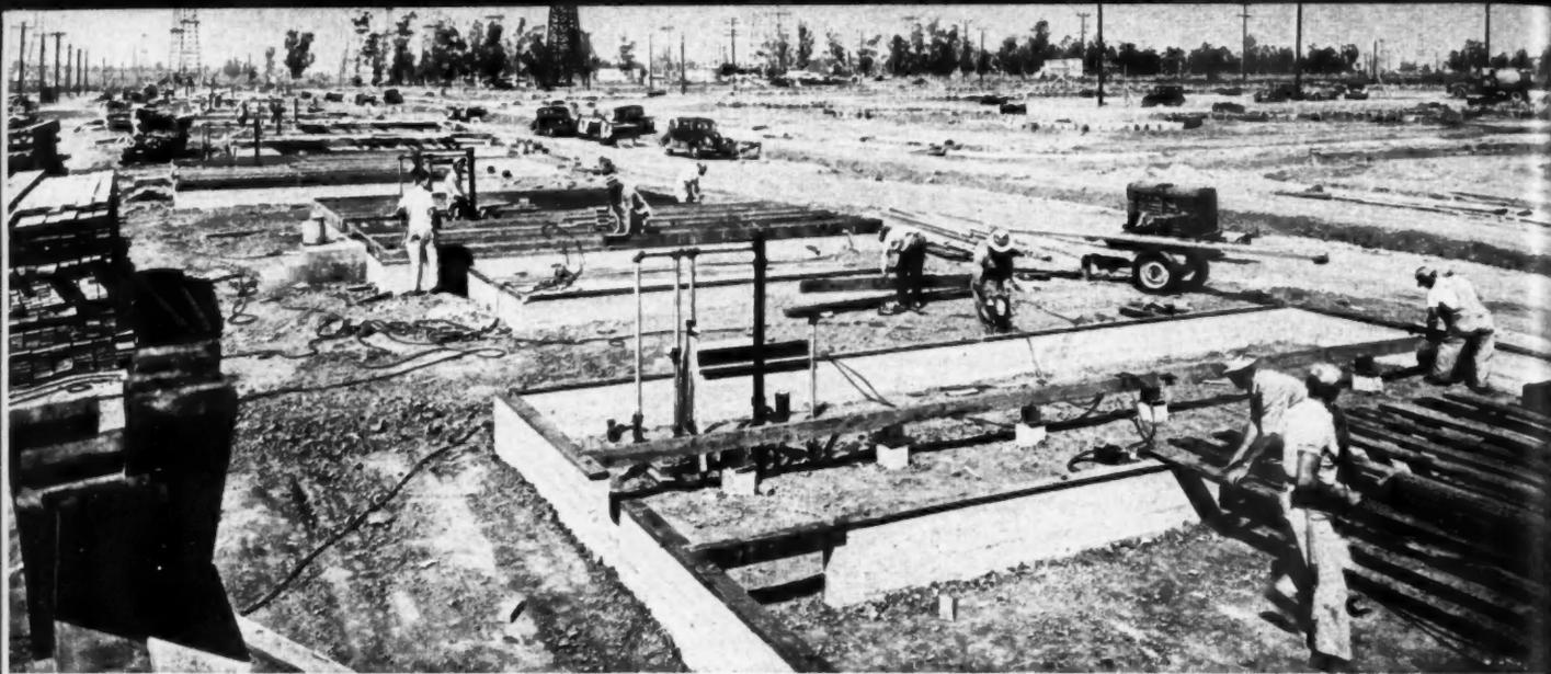
**HOLES** in mudsills are bored with a Skil-Drill by men in mudsill and girder crew. Left, a Cleveland trencher digs foundation footings. By careful stripping, oiling and handling, foundation forms have been used more than a hundred times
