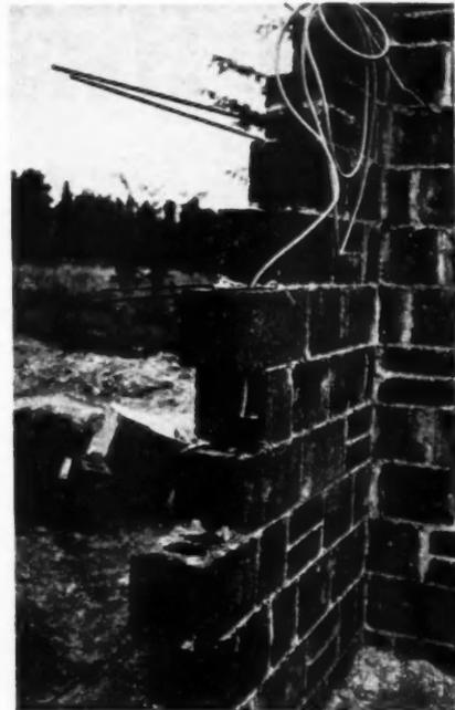
**PORITION** of cinder-block wall under construction. For additional rigidity reinforcing rods are placed in blocks. Voids in blocks are used for extending conduit
