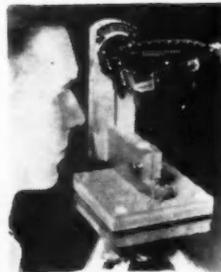
Aside from the fact that it has a tripod and plumb-bob the BURT QUADRANT-TRANSIT bears little resemblance to regular transits. It has two view finders, of the gun-sight type, at right angles, one being adjustable horizontally and vertically. A compass may be used. Weight complete with tripod 5 lbs.
