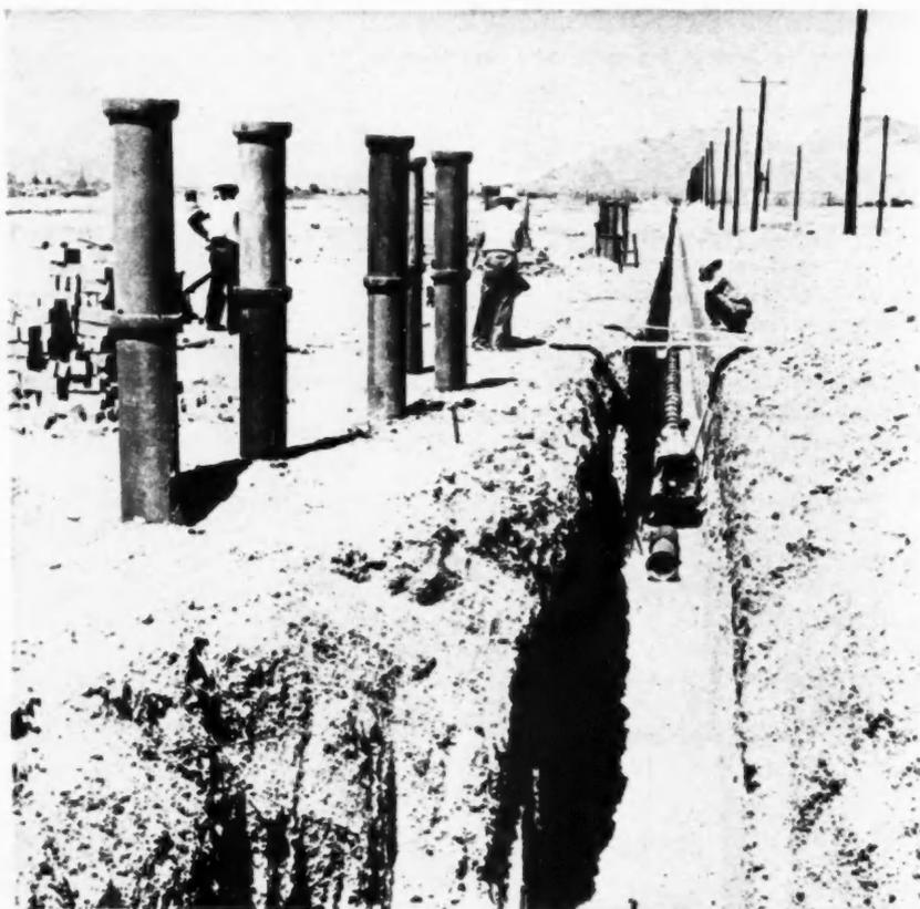
MORE than 11,000 feet of 8 and 10-inch vitrified clay pipe go to provide sewerage facilities for the first 700 homes. Over 50 miles of pipe will be installed
