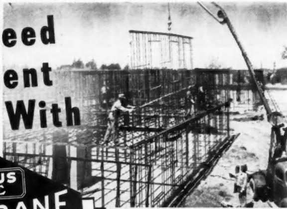
Here the Hydrocrane places steel wall frames. Full hydraulic control permits moving frames a fraction of an inch at a time if necessary—an important safety factor.
