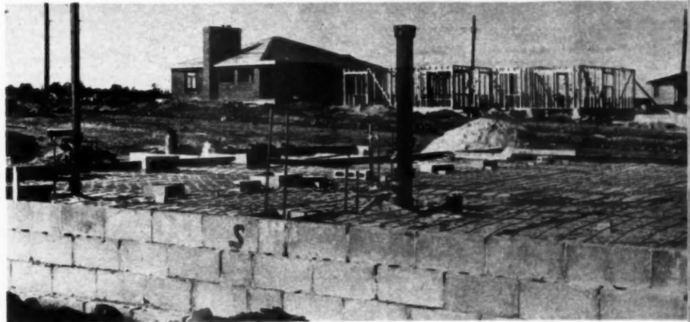
TYPICAL foundation of a Diamond Bar home. Moisture barrier has been laid over which steel reinforcing has been placed ready for concrete floor slab to be poured
