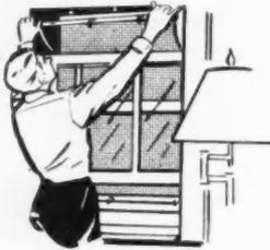
blind stop and drawn taut at sill with thumb screw. Tension is maintained on sides by five strand salvage edge, and "free floating" sill bar at bottom corrects out-of-square sills. Keystone Wire Cloth Co., Hanover, Pa.
