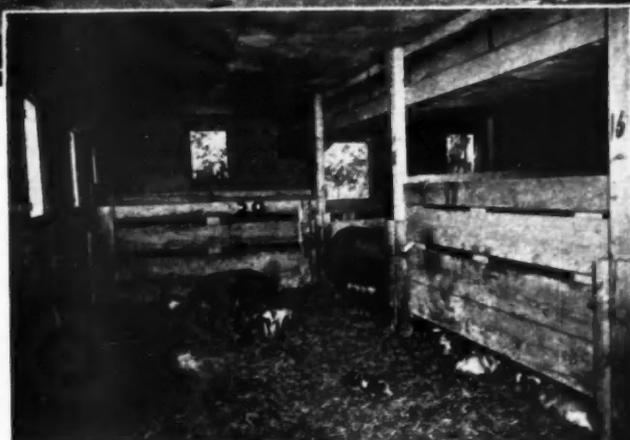
HERE is the interior of the old hog house after remodeling. Note dry condition of floor, ventilating duct and adequate insulation
