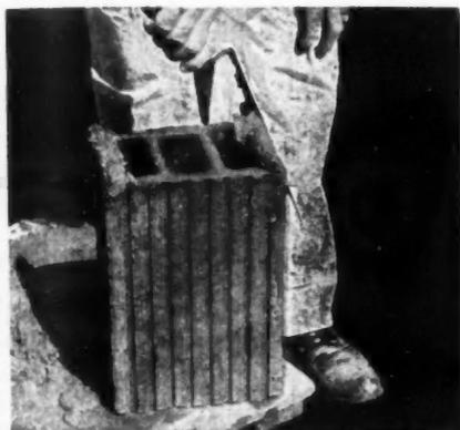
Method 1. Full head joints should be thrown onto both edges of the tile to be placed, or—
