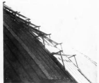
VIEW of vapor seal before application of aluminum sheets on the roof of the University of Minnesota fieldhouse. Eighty-five thousand pounds of sheets, cross seams and extruded battens were used to re-roof this 22-year-old structure.
