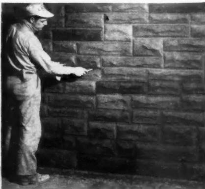
AFTER the student has created a stone-like pattern, he is taught to blend it with natural stone granules of various colors, using a special blowing device. The margin of each stone block is then tooled to create the true mortar joint
