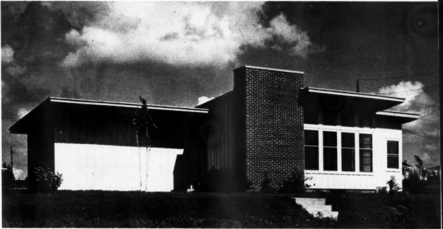
THIS modern design by McEnary & Kraft, project architects, offers a compact two-bedroom arrangement with attached garage. Exposed rafters on overhang adds a note of interest to shed roof. Plan of first floor at the right
