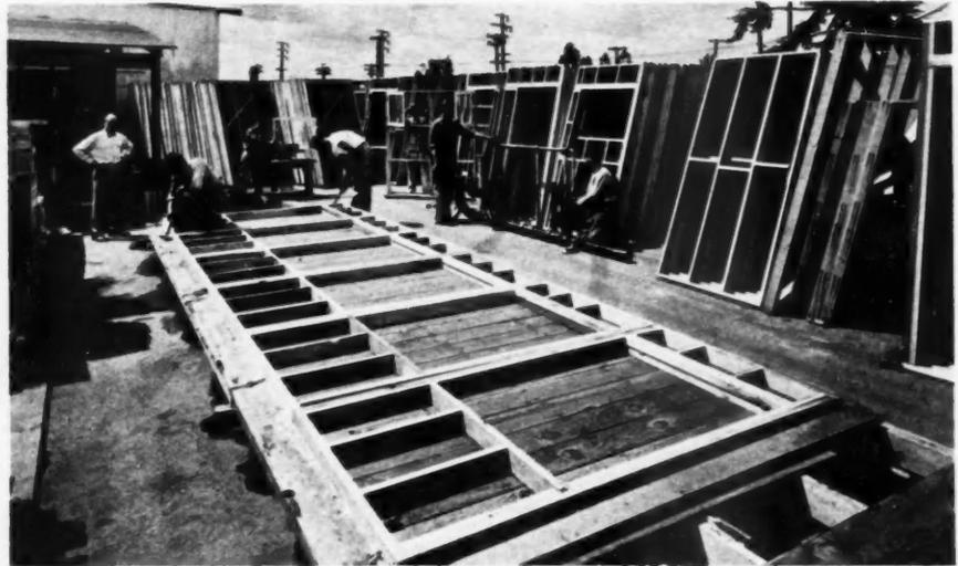
ALLIED Building Supply Co. yard, showing jig table and stock of completed wall panels
