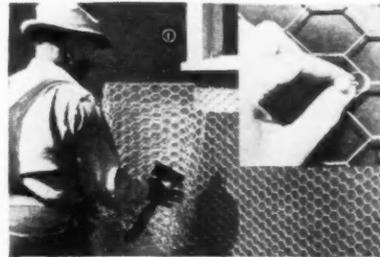
force stucco. It is available in two weights, woven of 17-gauge galvanized wire into a 1 1/2-inch hexagonal mesh, and 18-gauge galvanized wire in 1-inch mesh.
