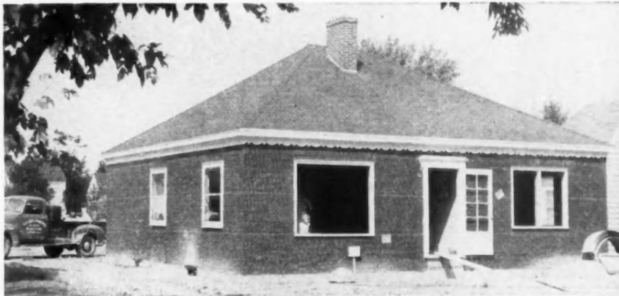
KEYMESH REINFORCEMENT applied on five-room house ready for first coat of stucco
