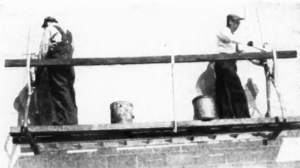
Faster, easier, safer operation of suspended scaffolds is provided by this new SAF-T-SWING winch and stirrup unit. A complete SAF-T-SWING Stage includes two winches—each with attached stirrup and 150 ft. of steel cable—guard rail and center post. The stirrup can also be replaced by a bosun's chair.
