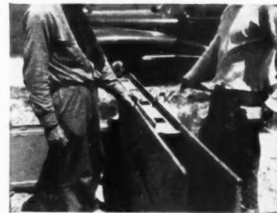
LIGHTWEIGHT interlocking metal members, with clips, holds side board panels
