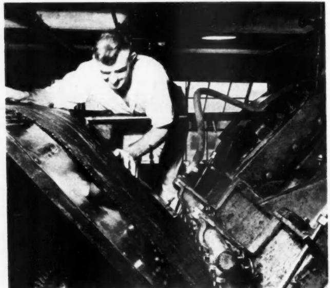
**7.** HERE the material is carefully fed into a punch press where it is die-cut into tile with square edges
