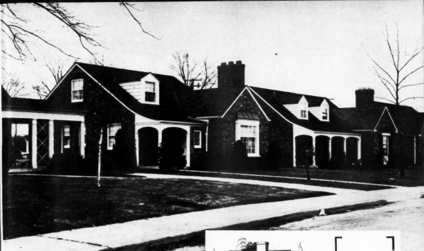
busy all the time. Most of the houses are brick or stone veneer, and many of them have fireplaces. Foundations are concrete blocks. Interior walls are plastered over gypsum lath. All ceilings are insulated with cotton insulation, and in some houses, the sidewalls are also insulated with the same material. Heat is supplied by Lennox oil-fired forced warm air furnaces.
