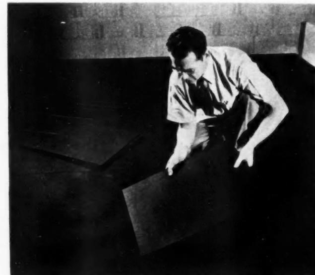
**8.** INDUSTRIAL tile is hand set, block by block in fast-setting cement. Floors are ready for immediate use
