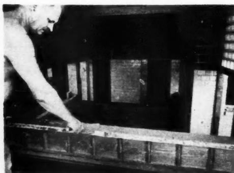
**TROWELING** becomes a simple operation of leveling off the mortar bed. Fixture permits a relatively dry mortar mix
