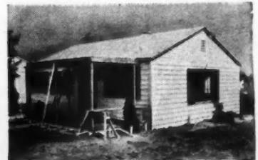
Porch being applied to the completed house, showing Reynolds Lifetime Aluminum Clapboard Siding with its final (second) coat of paint.
