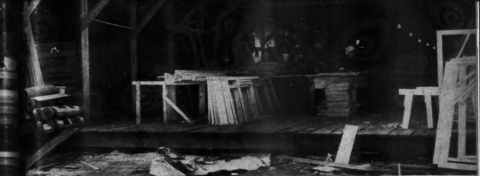
OTHER end of Kelly-Generes temporary job site shop. Wall panels are produced here, and doors and sash fitted in shop-made frames.
