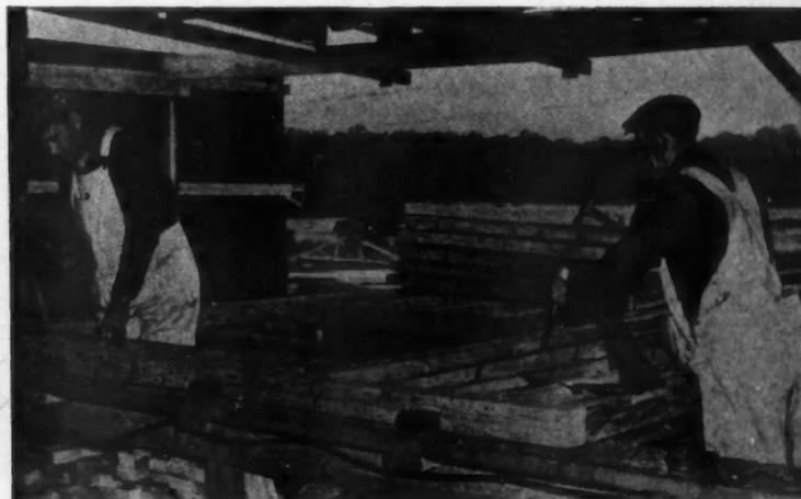
WALL and roof sections are site fabricated, ready for assembly.
