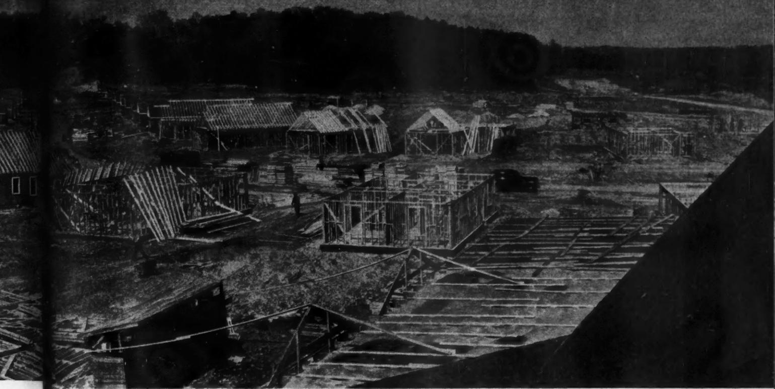
Md., showing all stages of field work, from site development to framing, trimming and landscaping, being performed simultaneously.
