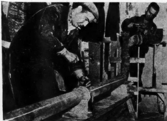
PLUMBING and heating assemblies are shop fabricated and tested.
