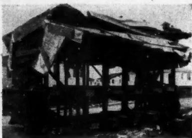
TO make short lengths of dimension lumber that is often wasted, available for use, Kelly-Generes, New Orleans, La., builders rigged up this portable storage shed that moves on skids with the aid of a cable to different points of operations. It is divided up into sections where pieces may be stored according to their lengths. Marker is placed in front indicating their sizes.
