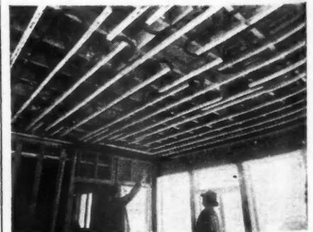
**HEATING** coils installed in ceiling ready for installation of metal lath and plaster.
