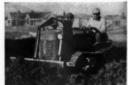
to operate close to the walls of houses and make close turns around trees, thereby accomplishing work which formerly required hand labor. The dozer is hydraulically operated with raise, lower, floating and hold positions, and is easily transported.
