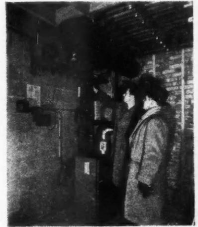
**BOILER**, pump, electrical controls, expansion tank and pipes to coils in ceilings.
