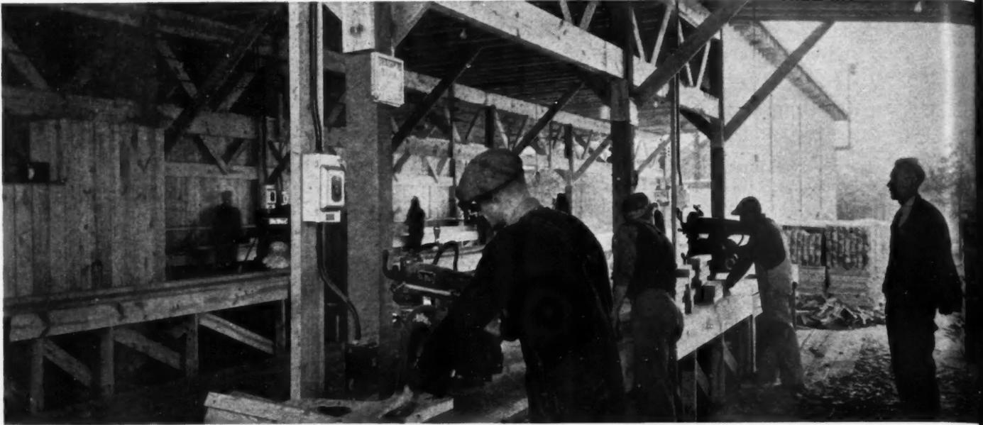
**SITE prefabrication is profitable on multiple housing jobs. Here power saws play an important part in precutting.**
