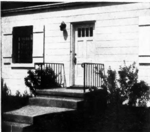
Horizontal joints were emphasized in this house in Joliet, Ill., by making them concave with a jointing tool. Vertical joints were cut flush and tight. The walls were finished with portland cement paint.
