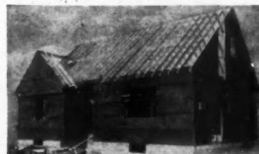
**CUTS SHEATHING COSTS 1/3 to 1/2.** One man can handle the 1/2"x2'x8' panels, cutting and nailing right on the studs. You can use brick, wood, asbestos, stucco or stone exteriors.
