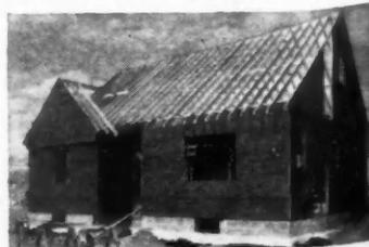
**CUTS SHEATHING COSTS** ½ to ⅓. One man can handle the ½'x8'x2' panels, cutting and nailing right on the studs. You can use brick, wood, asbestos, stucco or stone siding.
