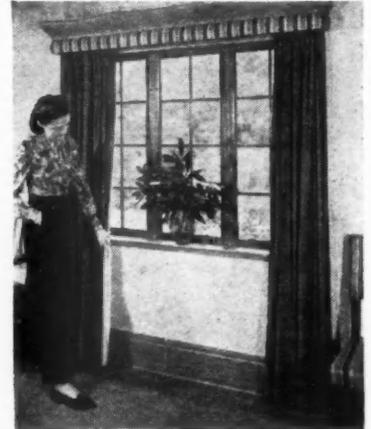
Replacing the conventional wooden baseboard, the new heat panel delivers radiant heat rays into the room at ankle height. In appearance it is a hollow cast iron unit 7 in. high and 1¾ in. wide, connected with the usual heating boiler. The panels are installed on the outside walls in place of the regular baseboard and painted to match the woodwork of the room.
