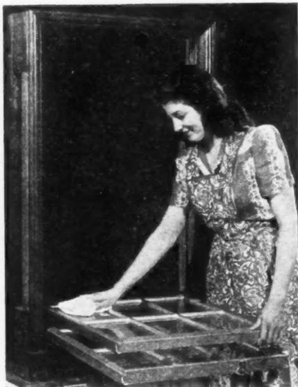
The weights, chains and pulleys have been replaced with a new patented device which provides smooth, noiseless and non-rattling up and down movement.
