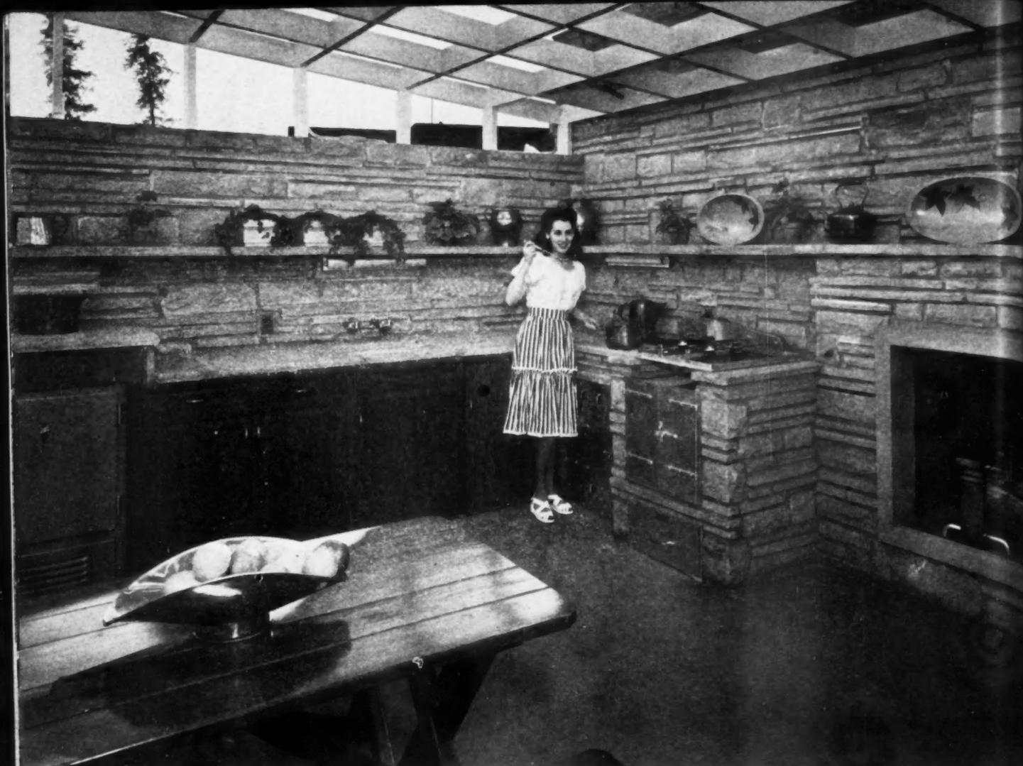
**WITH HEARTH** and background of flagstone and wall stone, barbeque is an attractive and completely equipped outdoor kitchen. Note refrigerator at left, and work top, cabinets, shelves and broiler. Barbeque has hot and cold running water and radio connections.
