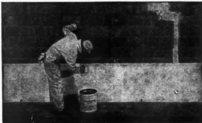
B. THOROSEAL, a slow-set hydraulic compound, gives the applicator 2 to 4 hours, before set begins, to brush THOROSEAL into the masonry surface. (Scrubbing not necessary, as THOROSEAL is prepared especially to flow easily and quickly into every crack, void and defect in the surface, where it becomes structurally stronger than the surface to which applied.)
