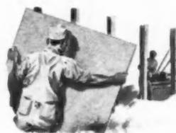
**TEMLOK\*\*** . . . the efficient, easy handling, Armstrong fiberboard insulation, available in sheathing, lath, and de luxe interior finish panels, planks, and boards.
