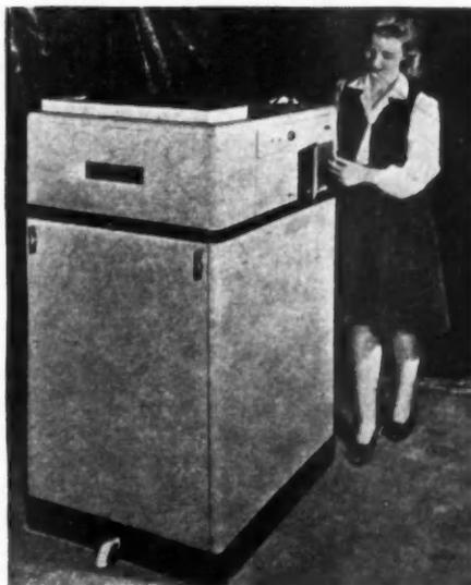
**COMPACT** and wholly enclosed, the Precipitron home unit is no larger than a refrigerator.
