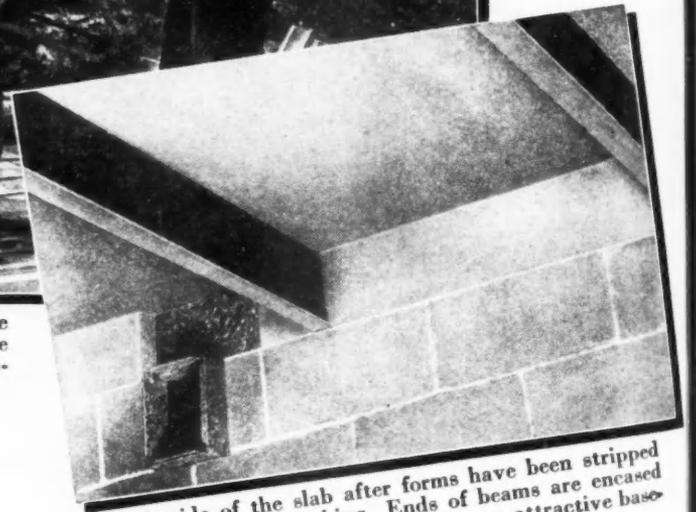
Underside of the slab after forms have been stripped for use as roof sheathing. Ends of beams are encased in concrete fire stop. After painting an attractive basement will catch the eye of prospects.
