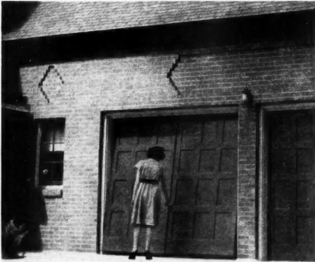
● Architects and builders have been quick to use "Over-the-Top" Door Equipment because of its versatility. It can be installed on standard or mill-made doors, weighing up to 720 lbs. and having openings from 6' 6" high and 7' wide up to 12' high and 18' wide. "Over-the-Top" Door Equipment requires only from 2 1/4" to 6" headroom, depending on size of door. It is simply made, easy to install, and costs less than most overhead door devices. Write for new brochure containing complete details.
