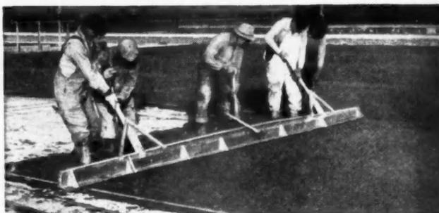
• Screeding Zonolite Insulating Concrete roof fill over concrete slab. Easily formed into saddles and cants for proper drainage.
