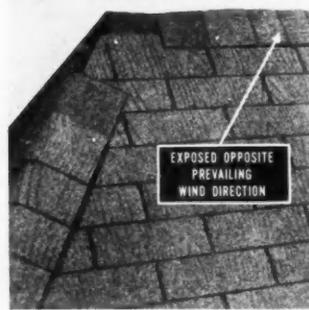
Plan courses so nails at ridge are covered by at least 1" of overlying ridge shingle. Last course of roof shingles may be turned over or trimmed even with ridge. Shingles at hips should be trimmed even with hip line. For cover shingles on ridges and hips, use Master-Bilts cut in thirds and trimmed to edges of "cut-outs". Lay with butts exposed 5" to weather. Place nails 1 1/2" from each side, not over 6" from butts. On ridges always expose opposite prevailing wind direction.
