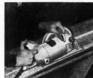
Cutting Rabbets ten times as fast as by hand with Grooving Blade.
