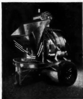
Loads and measures while you mix, then shakes waiting batch into drum. Fastest, huskiest half-bagger built; machined steel drum tracks, other 1945 features. Get Catalog JM-5.
