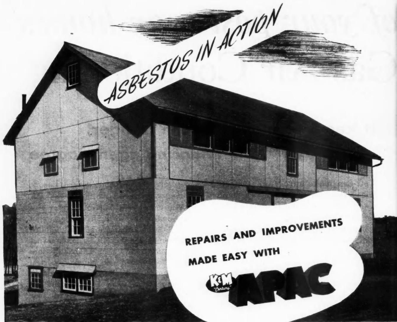
No matter how old the barn, house or shop, you can quickly repair or improve it with this all-purpose asbestos sheet material. It is easy to handle . . . easy to apply . . . amazingly adaptable. "Century" APAC is cut by scoring one side with any sharp pointed tool—then simply snapping it. It is easily fastened too—with nails or screws.
