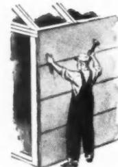
Celo-Rok Weather-Proof Siding is a fire-resistant gypsum board for use in place of both sheathing and siding. Treated with weather-proofing compound. Green-finished exterior requires no painting.
