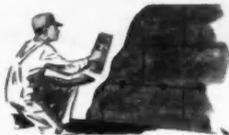
• Insulite Sealed Lok-Joint Lath, with asphalt barrier against the studs, retards vapor travel. Bildrite Insulating Sheathing, being permeable to vapor, permits what little vapor escapes the barrier to pass towards the outside.
