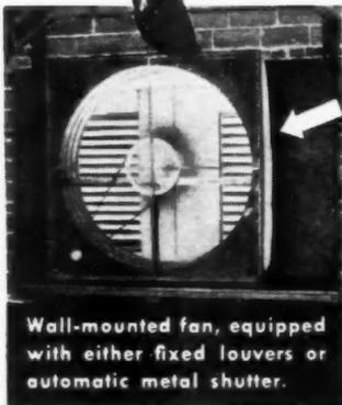
Wall-mounted fan, equipped with either fixed louvers or automatic metal shutter.
