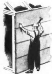
Celo-Rok Weather Proof Siding is a fire-resistant gypsum board—a single structural material which will serve in place of both sheathing and siding. Both surfaces and all edges are treated with a weather-proofing compound. Exterior side is finished in green and requires no painting. Available in 1" thickness with ship-lapped long edges and 1/2" thickness with T&G long edges—24 inches wide, in 6, 8, 9, and 10 foot lengths.
