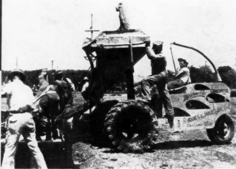
**2 CONCRETE LOADED AT CENTRAL MIXER** is carried in a Mixermobile buggy for pouring into foundation forms; 48 hours later forms are stripped, walls sprayed with a seal cure.
