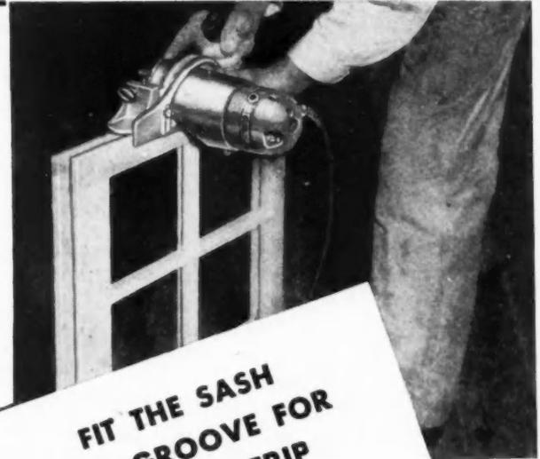
**FIT THE SASH AND GROOVE FOR WEATHERSTRIP WITH THIS ONE CARTER TOOL**
