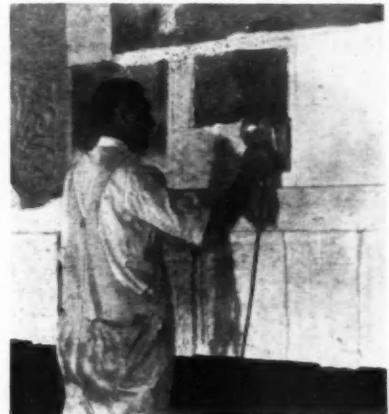
**How To Apply Cement to Acoustical Tiles**
