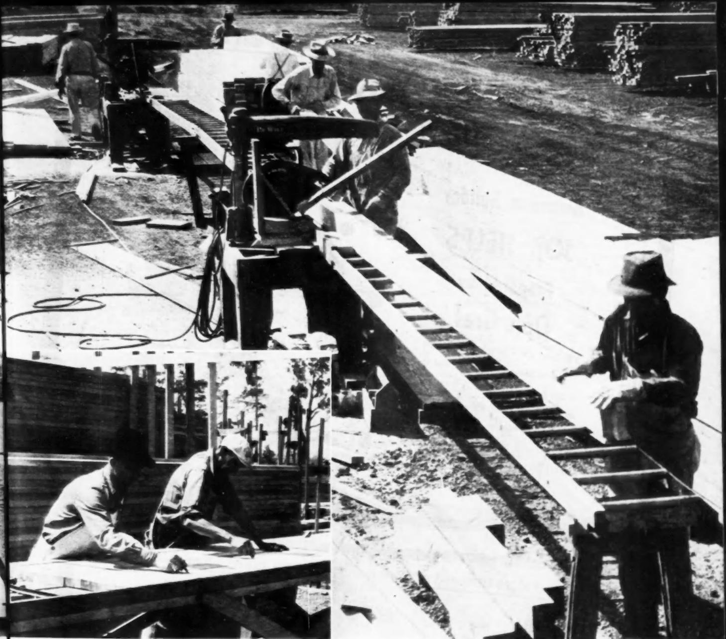
**4** PRECUTTING AN IMPORTANT STEP as shown above. In insert two workmen near stock pile are multiple marking studs for window, door openings, partitions, etc. From there framing is passed along to the cutting line where two cuts can be made without lifting off roller table as shown in larger view of cutting yard. Seven men cut 700 rafters in an hour with a setup such as this.
