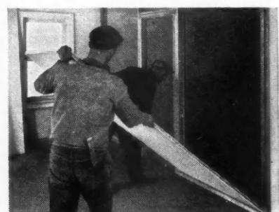
**For Inside Walls and Partitions**—Gold Bond Solid Partition Panels are fastened between the studs by mouldings. Their large size means speed on the job. Their strength insures solid, rigid walls. Permanent or demountable and completely salvageable.
