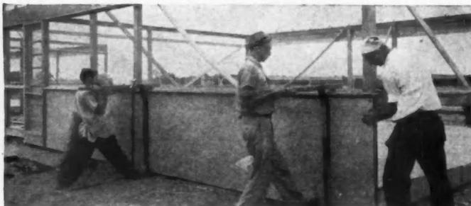
**2** A sheet of 1½" Cemesto is being applied to the lower section of wall. Panel is 12' long, 4' wide.
