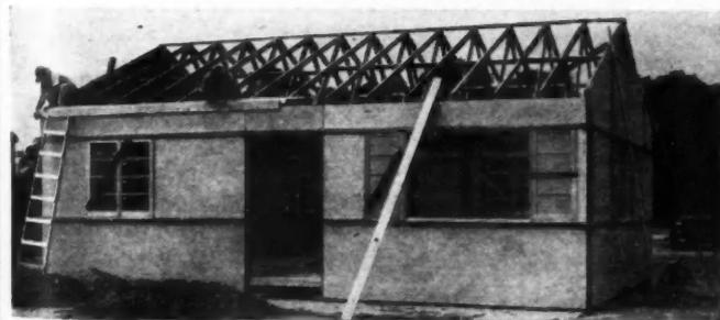
**5** All roof trusses have now been installed. These are put up at the rate of about one per minute.
