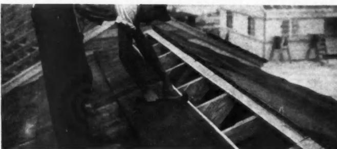
**6** Celotex Celo-Roof combines insulation and roofing and is applied direct to roof trusses.
