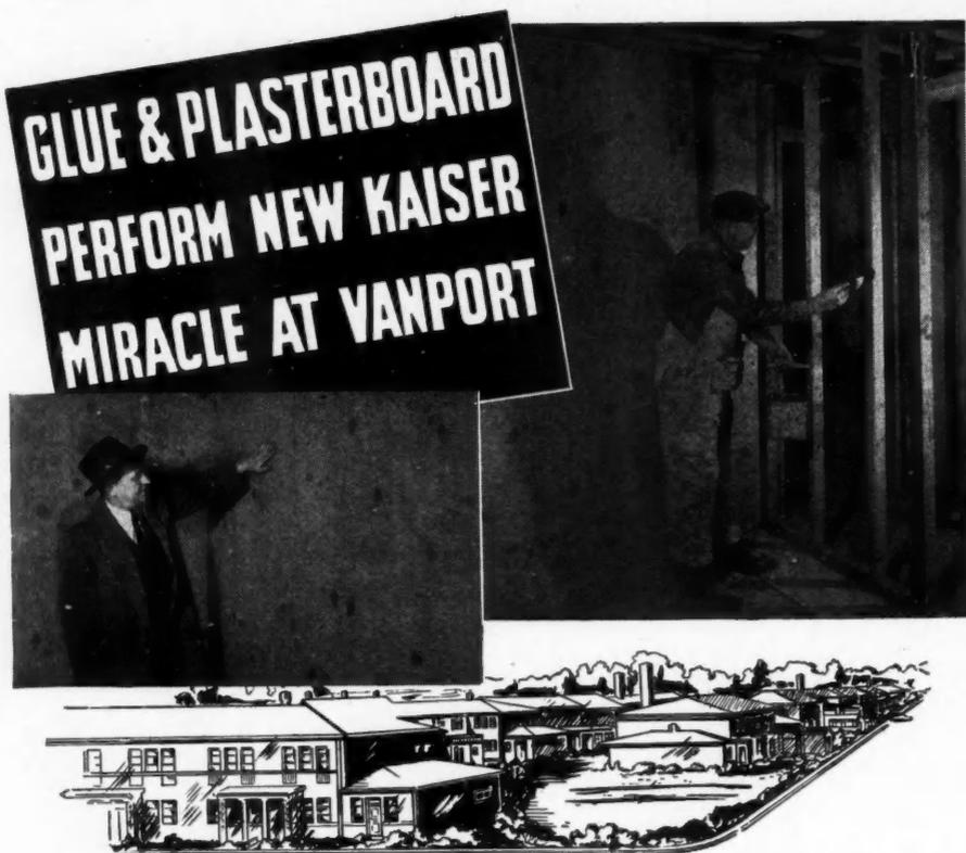
RIGHT: Brushing Laucks Construction Glue on studding before applying Wallboard. LEFT: Frank Stepanek, "expediter" of glue and plasterboard walls, for world's largest housing project.
