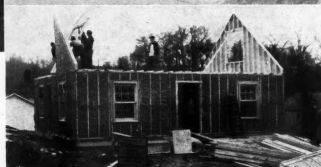
**ABOVE:** All sections for a house loaded on truck; at site they are quickly assembled, ready for exterior finish.
