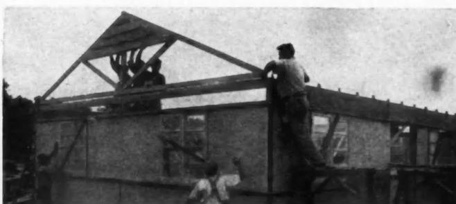
**4** An end roof truss, equipped with ventilating louvres, is fitted into position in a matter of minutes.
