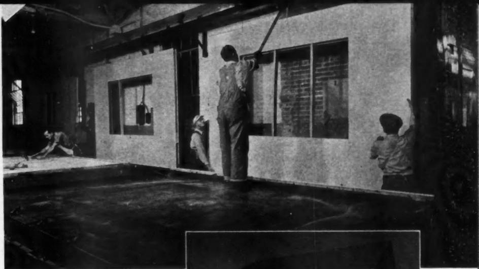
OVERHEAD conveyor transports these large panels after fabrication on jig table in foreground. House at right is typical unit built by Libbey-Owens-Ford Glass Co., using the National Homes System.
