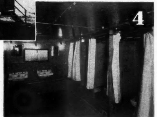
*Two laundry units (as shown at left) and four toilet units (as shown at right) are sufficient for every 100 dwelling units.*
