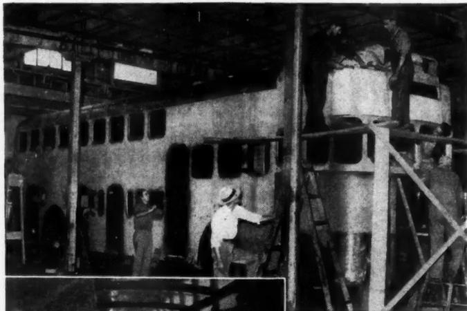
(At top of page) One of Santa Fe Trailways' smart new 117-passenger Victory Liners. The exterior, interior, partitions and floors are built of Douglas Fir Plywood. Now under construction is a 150-passenger all plywood Victory Liner.
