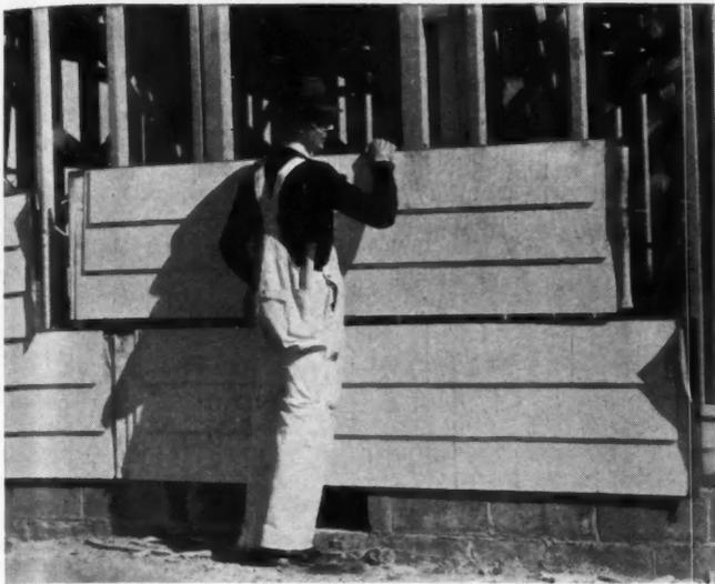
THE Weatherseal panel comes 2 x 8 feet and cuts erection time.
