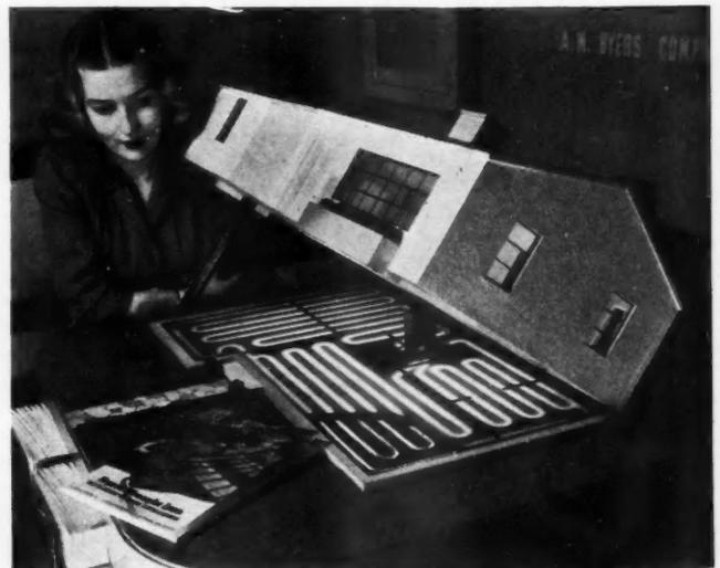
MODEL house tips up to show heating pipes in floor.
