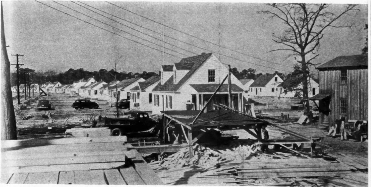
FOUR HUNDRED houses are scheduled by Contractor V. T. Myers in his Monticello-home job in Norfolk. Lumber stored in foreground is pre-cut on power saw, trucked to each foundation site. BELOW: Red cedar shingle exteriors being applied. Plans on next page.
