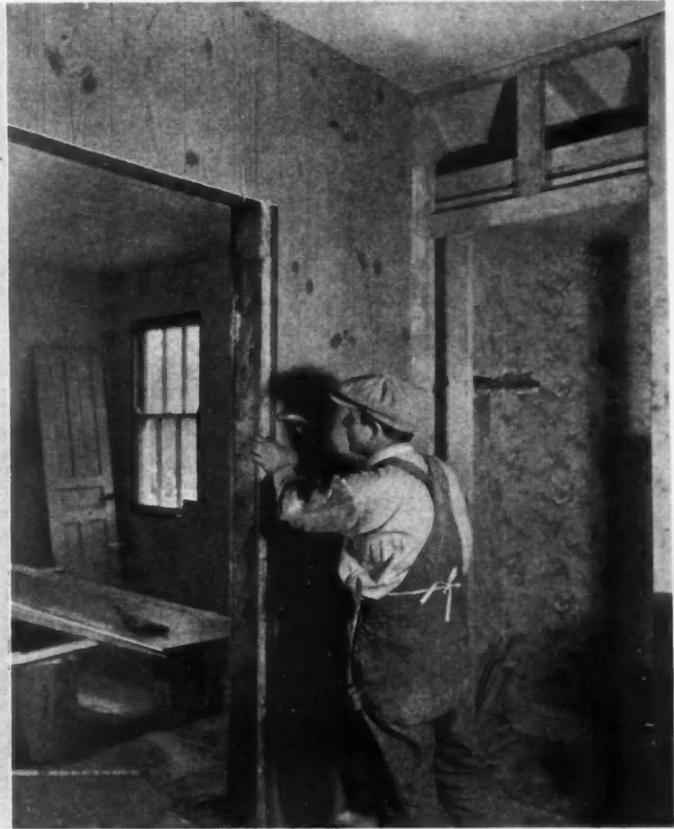
**AIR DUCTS** are run between joists and are of gypsum board, thereby saving on sheet metal; front hall is finished in Knotty Pine Sheetrock, square edge boards butted tight to make an invisible joint.
