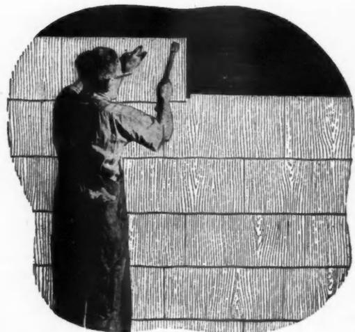
STAINLESS steel face nails are always used with "Vitramic" siding. These nails are of super rust-proof quality . . . the strongest rust-proof siding nails made.
