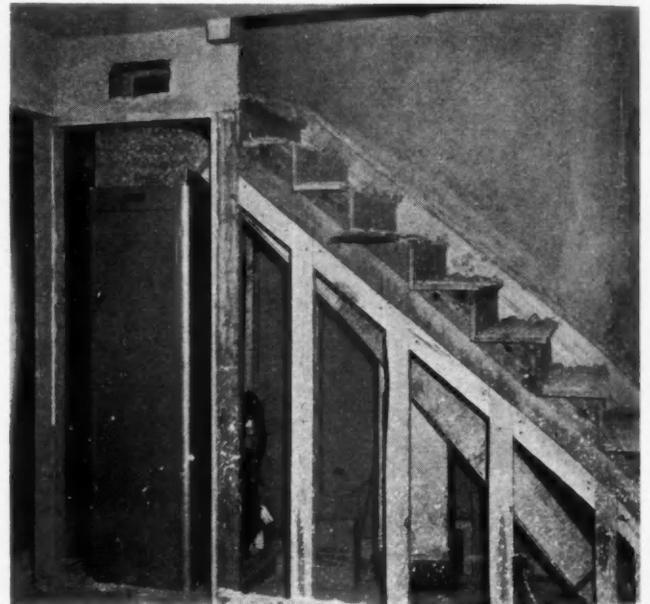
HEATING PLANT under stairs. In 2-story model illustrated on opposite page Myers installs a compact unit under the stairs with short runs of ducts carried in a furred down ceiling to rooms.
