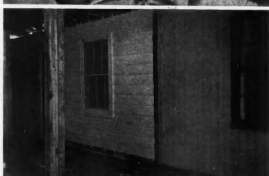
**EVEN** gable ends are finished complete with windows in place and screens hung. Sections here are ready to move on to loading platform where they will be shipped to site and erected as shown at far right.
