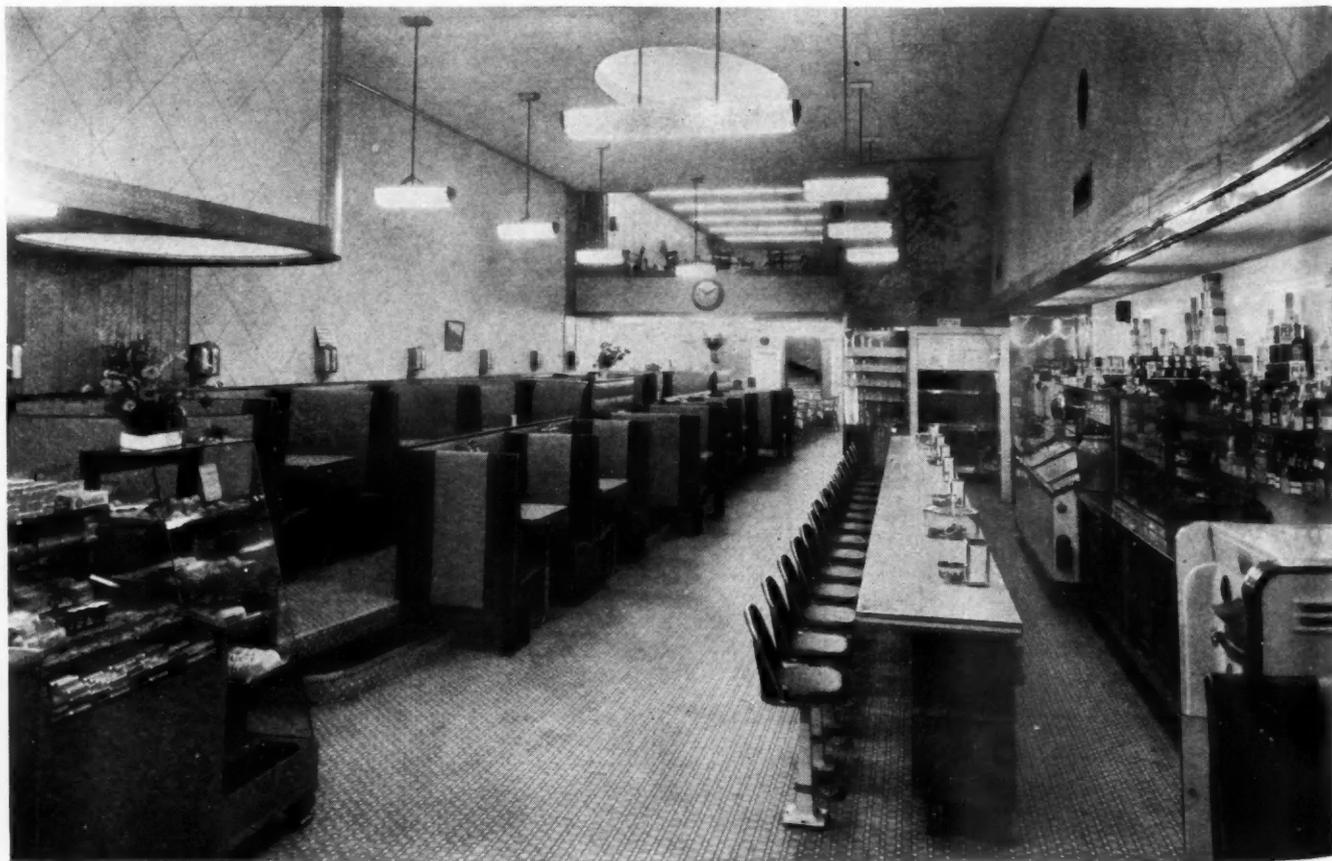
INTERIOR WALLS are finished in insulating board; balcony can be seen at far end of restaurant.
