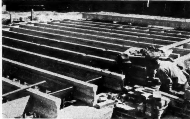
Top, attractive new home of Fred Lang, of Cunard-Lang Concrete Co., Columbus, Ohio, concrete blocks in foundation and cinder blocks, painted, above grade. Center, residence built with units produced by Cinder Block Co., St. Joseph, Mo., which also produced the concrete joists, lower photo. 'Incor' and Lone Star used throughout.
