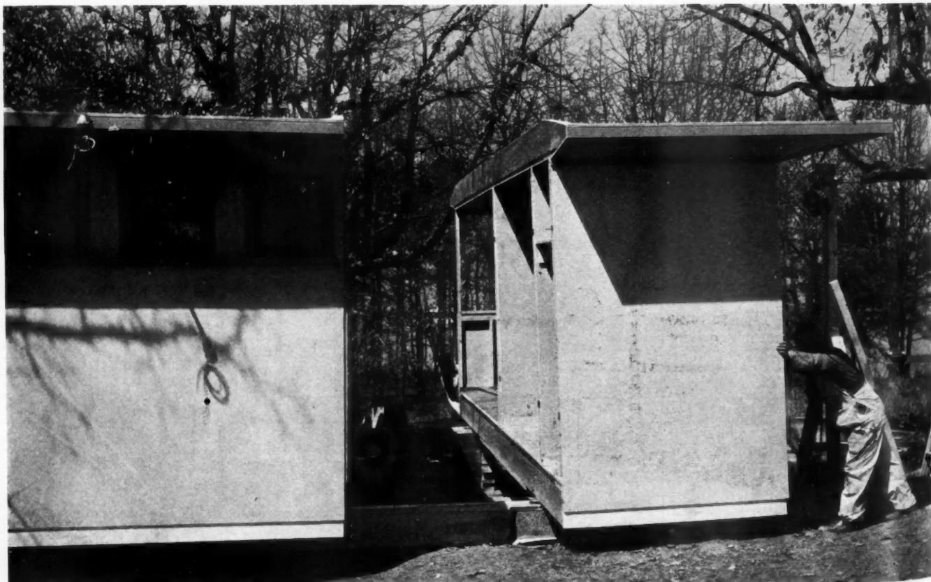
SECTION, lowered off truck onto prepared foundation, rides easily along prepared rail—1" pipe and small pulley wheels. Section is fully equipped and wired and has plumbing and heating installed.
