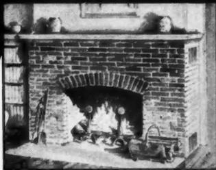
... With the double-walled steel Heatilator serving as a form for the masonry, you can build any style of fireplace and be sure that it will work properly . . . **WILL NOT SMOKE** . . . and that it will *Circulate Heat*.
