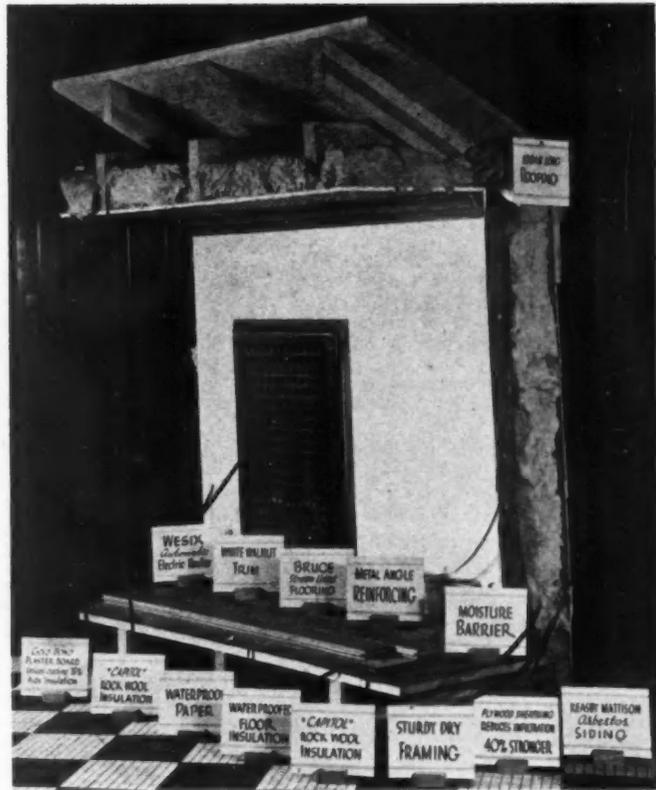
THIS sectional model of Fonde construction is displayed in the window of the City Power Board. It shows electric heater, thorough insulation, quality building in this "first smokeless community."
