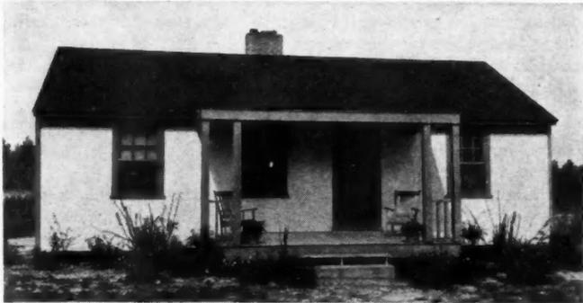
According to W. V. Albright, district engineer for the FSA, the "cotton house" (four-room structure as shown in the picture) can be built for about \$1,350, which is about the cost of an ordinary frame dwelling with wood siding and shingle roof. The house is ceiled with plywood.
