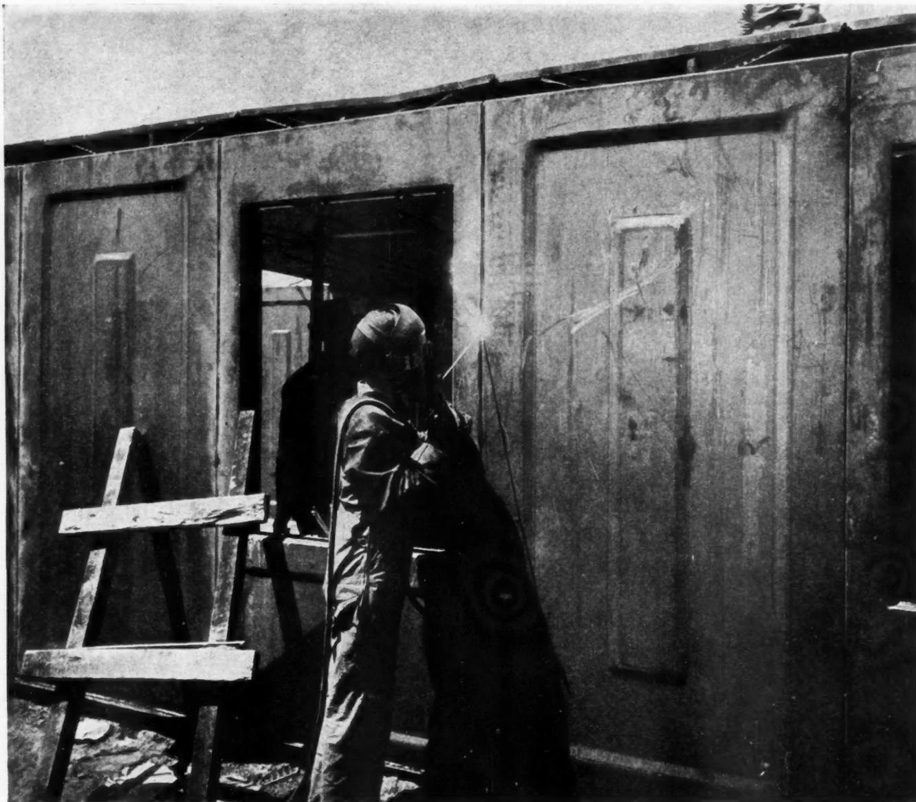
FIELD ERECTION of welded steel structural panels in Georgia industrial project.
