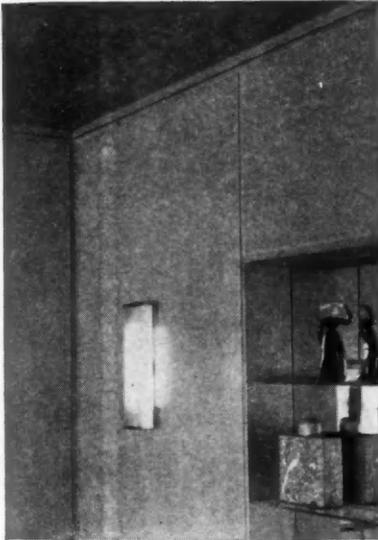
OPEN joint paneling, as in close-up at left, is detailed in diagram. Panel edges are quickly rabbeted with power router shown in operation below.
