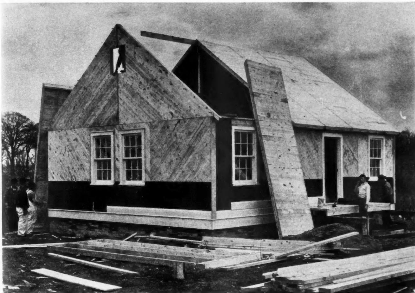
FIVE by 14 ft. roof section about to be set into place, on low-cost house of Richmond Housing Corp.; forty-two sections are used.
