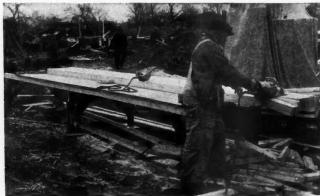
CONSTRUCTION views show, top, 2 by 6 subflooring being laid over 4 by 8 joists; center, looking down the trench excavation, workmen laying out studding in foreground; bottom, power saws are used to cut wall studs and notch for ribbons.
