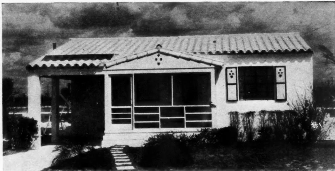
THIS Miami, Fla., home in new Lester F. Preu Corp. development features concrete block construction; as in other Preu houses, it has a solar water heater built into the roof over the porte cochere. The sun's rays furnish hot water.
