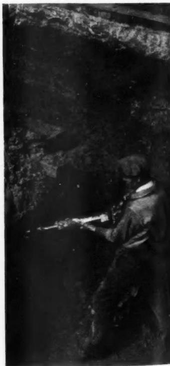
CONCRETE SURFACER (at left) operated by compressed air used on Indiana school. AT RIGHT, pneumatic clay digger speeds difficult digging.
