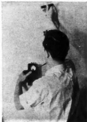
SIMPLE method of testing a plaster wall for moisture content with new detector to determine condition for decorating, finishing, etc.
