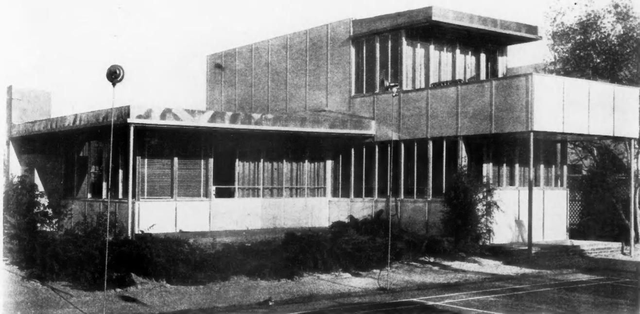
MODEL home in California. Outside walls of outdoor plywood; joints covered with aluminum batten strips. With waterproof joints architects are finding many new designs entirely practical.
