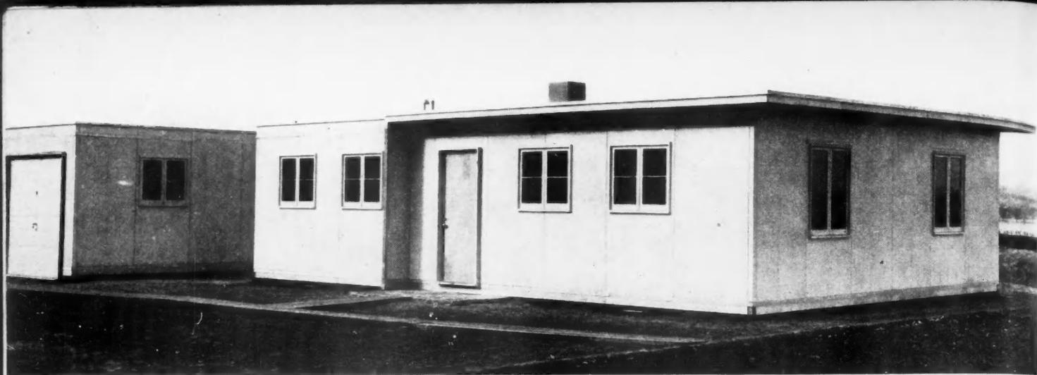
THE new prefabricated plywood panel house at Madison, Wis., designed and built by the engineers of the Forest Products Laboratory. Photo shows all panels in place and house completed.
