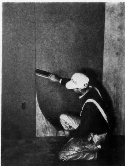
**UNIFORM** adhesion of the felt to the plywood is assured by going over it carefully with the smoothing brush.
