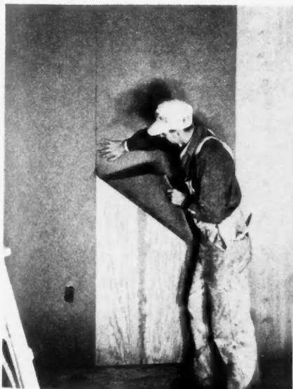
**THE** straight-edge felt is tightly butt-jointed, thereby providing an absolutely smooth surface for the paper.
