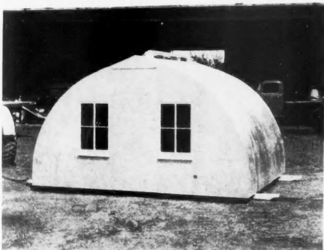
POULTRY brooder house using laminated bent rafters and plywood panels weigh less and are stronger than when built of natural lumber.
