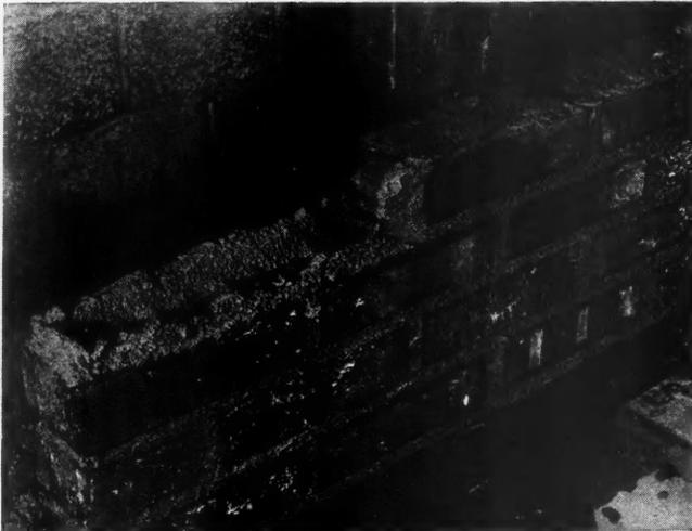
Figure 3—Workmanship B, showing furrowed bed joints and butting of bricks for head joints
