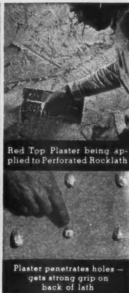
Red Top Plaster being applied to Perforated Rocklath
