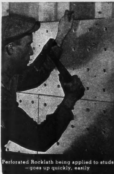
Perforated Rocklath being applied to studs — goes up quickly, easily
