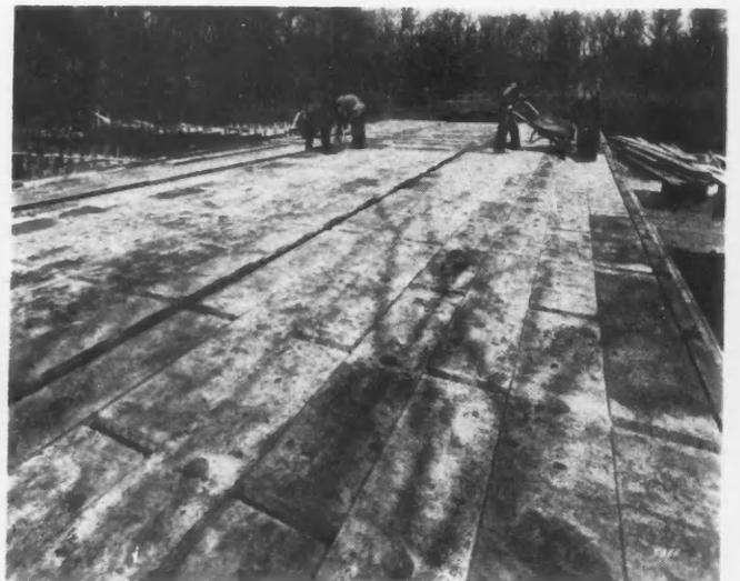
LIGHT WEIGHT concrete slabs in position and workmen pouring beams of Park house in Glen Ellyn.
