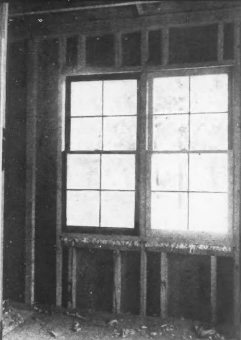
LEFT: View of framing around opening which has a lining of weatherstrip and serves as jamb and head. Note sash balances and narrow mullion; "Furstix" glue strips have been applied to joists and the stud at far left.
