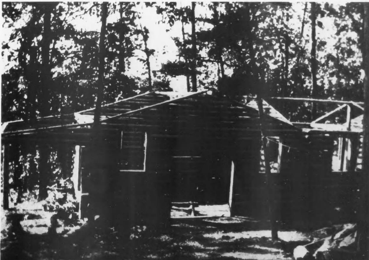
CABIN ready for roof and fireplace. Note how logs are graduated from the bottom up to top.
