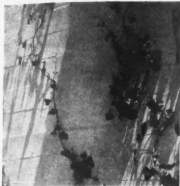
Monolithic concrete wall, board marked, painted. One of many textures possible at low cost when walls are cast in place.
