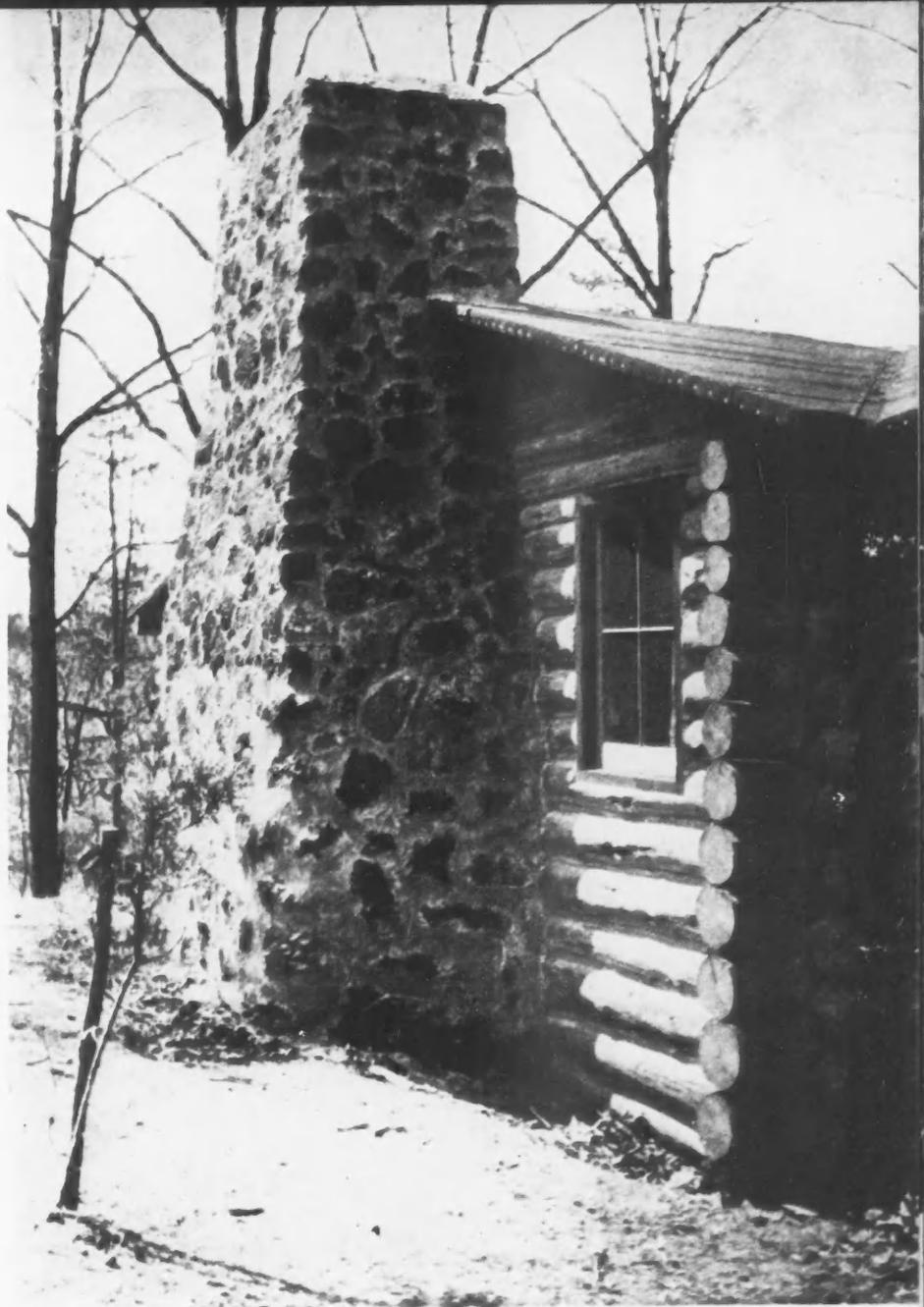
**GOOD** example of saddle and notch corner construction. Also note how second wall ties in behind first one avoiding use of too long logs.
