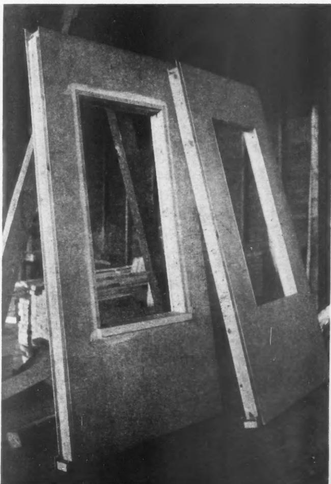
**SHOP-FABRICATED** plywood wall units; the one in foreground shows the exterior surface, the other displays the inside of a unit.
