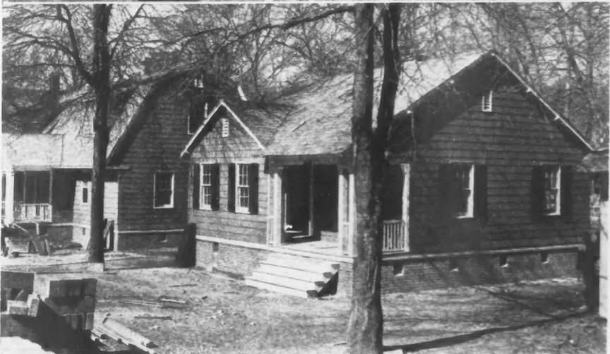
MUSCLE SHOALS house (above) being raised above ground level to overcome dampness and further attacks by termites. Note removal of shingles at corners to permit termite eradication and repair. Below, the same house after raising and termite eradication.
