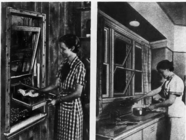
LEFT: Washing Jiffy-Kleen windows is done safely from inside. Right: Sash tilted for ventilation keep out rain and snow in bad weather.
