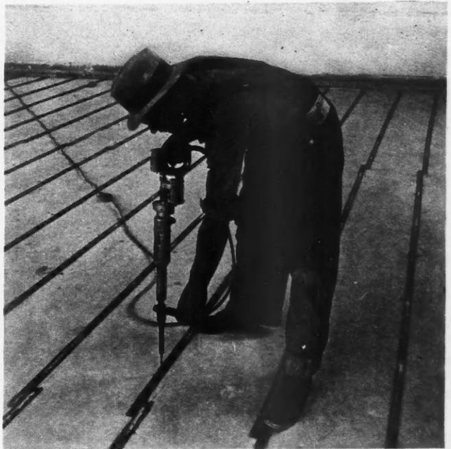
**SPEEDING** up the job. Combination hammer and drill used by F. & H. Construction Co., Chicago, for rapid installation of floor sleepers.
