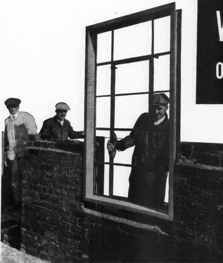
Method of installing in solid brick or block construction.
