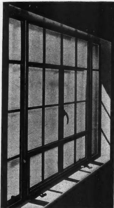
LEFT: Air-Conditioning Window as installation appears from interior with both casement and Tiltin sill ventilator closed; casement handle protrudes through circular aperture, fitted with rubber seal.
