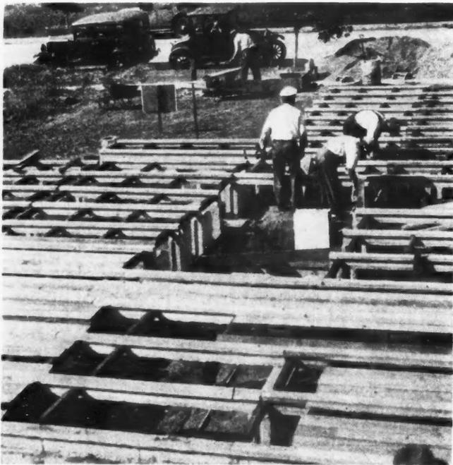
Construction view showing Joist being set and in place. Spreaders and Slab Forms in Place. To right are shown details of Girder, Joist and Slab construction.
