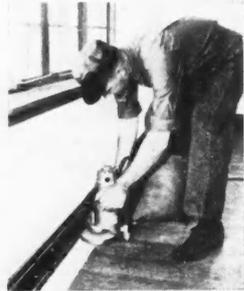
For floor sander operators. Sands and matches up the edges of floor of an ordinary sized room in 12 minutes—Write quick for information—also on floor sanding machines.
