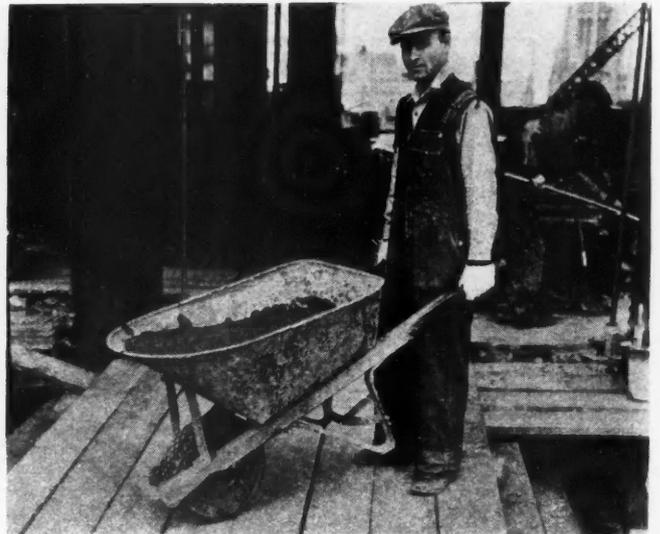
Pneumatic tired wheel barrows are being used for the first time in construction of the Field building, Chicago. Eastholm-Melwin, concrete contractors, says they eliminate laying planking over tile floors.
