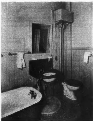
**BEFORE AND AFTER** views of a model modernizing job. The old roll rim tub, high tank closet combination, exposed lead piping, wooden wainscoting and other items are replaced in the model new bathroom by the latest matched fittings in modern design. Washable wallpaper, black rubber tile floor, rectangular mirror, two-way electric sockets, interesting modern details are effective.
