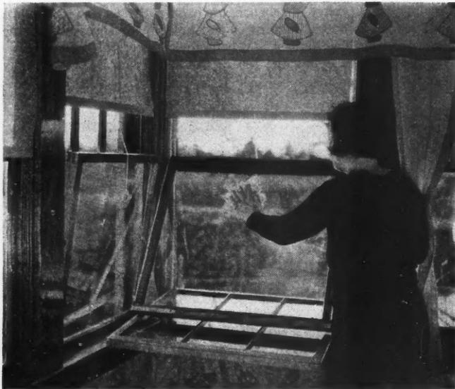
Bottom sash of new window pulls clear into room, reverses and slides up again. Top sash likewise pulls down, reverses.
