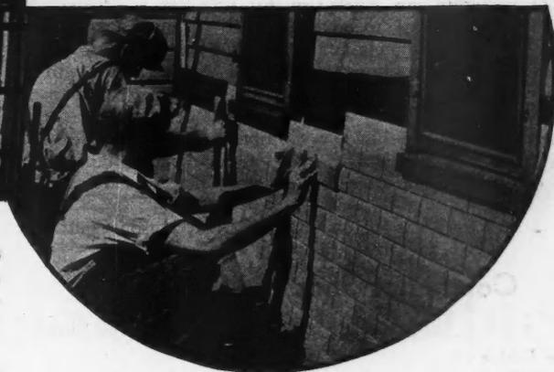
**R**UBEROID'S recent announcement of its ingenious Asbestos Cement Brick-Type Siding, textured like rough natural brick, has been enthusiastically received by carpenters and contractors.
