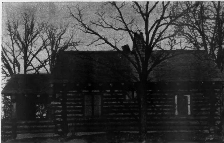
Sunset Lodge, built by C. B. Wilcox, illustrates several important points of log cabin building. Logs fit well together, have permanent, tight joints.
