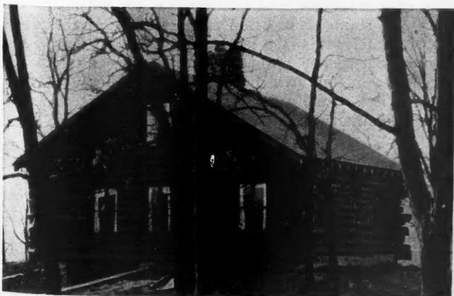
Rear view of Sunset Lodge showing entrance to garage in basement. Although inexpensive, this cabin is built to last many years and is warm and weathertight.
