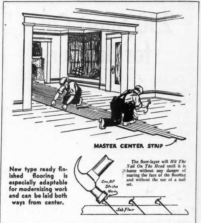
New type ready finished flooring is especially adaptable for modernizing work and can be laid both ways from center.
