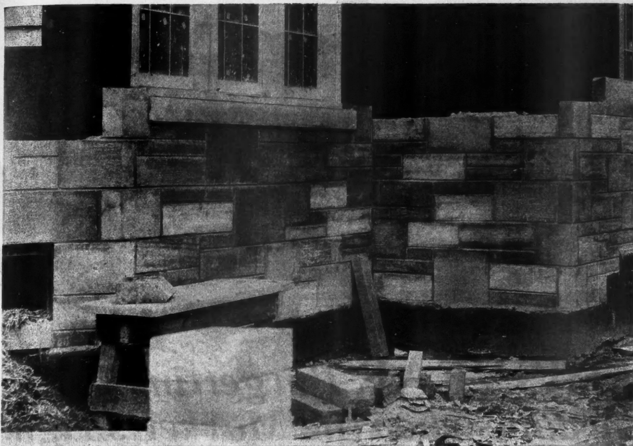
This view shows method of construction. Note stacked slabs of stone.
