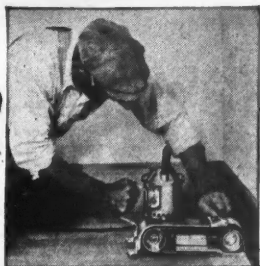
Finishing butt ends of floors with the edging attachment
