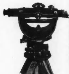
Level and Transit Are Combined in This One Instrument for the Use of the Builder.
