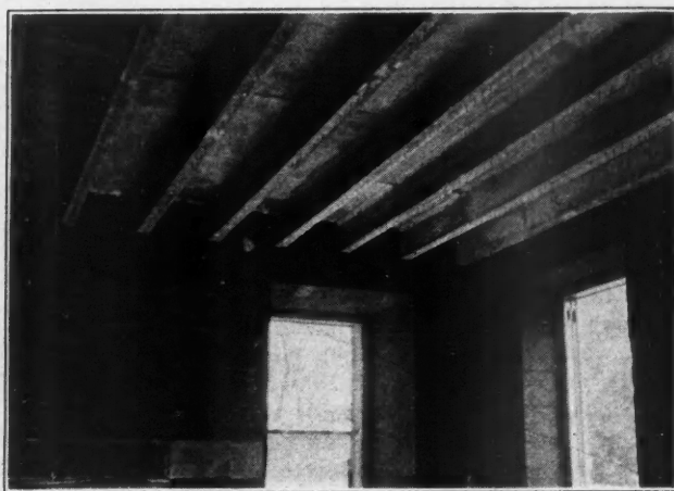
Hangers Imbedded in the Concrete Joists Provide a Means of Attaching Metal Lath to Which Plaster for Ceiling Is Applied.
