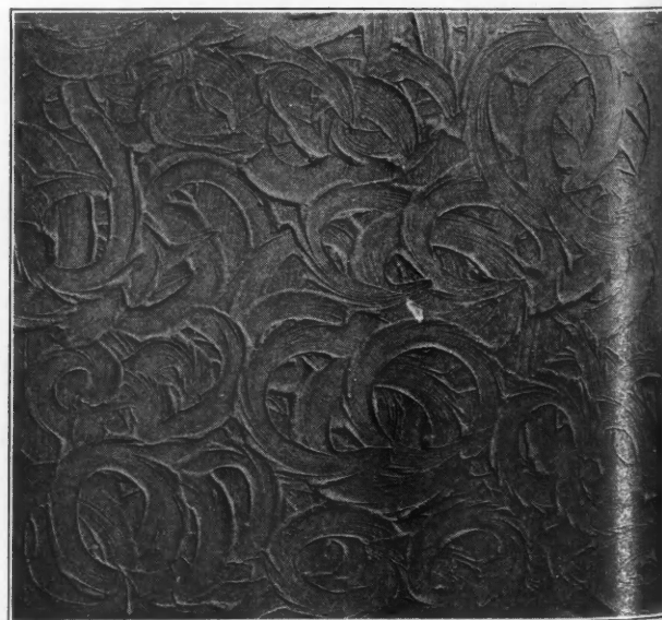
Figure 4—An Unusual Effect but Very Simple to Produce with the Curved Back of a Serving Spoon.
