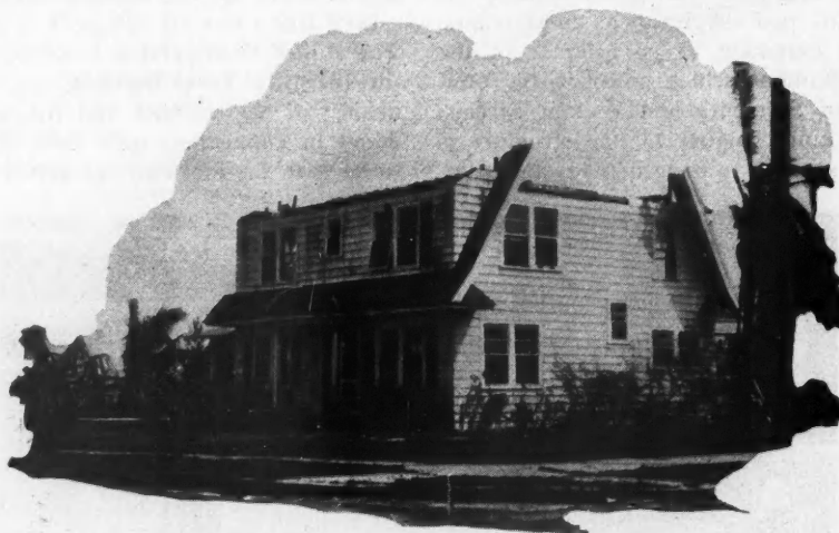
Lack of Anchorage of Roof to Side Walls Accounts for This Typical Roof Loss in the Recent Florida Storm. Good construction would have prevented this damage.
