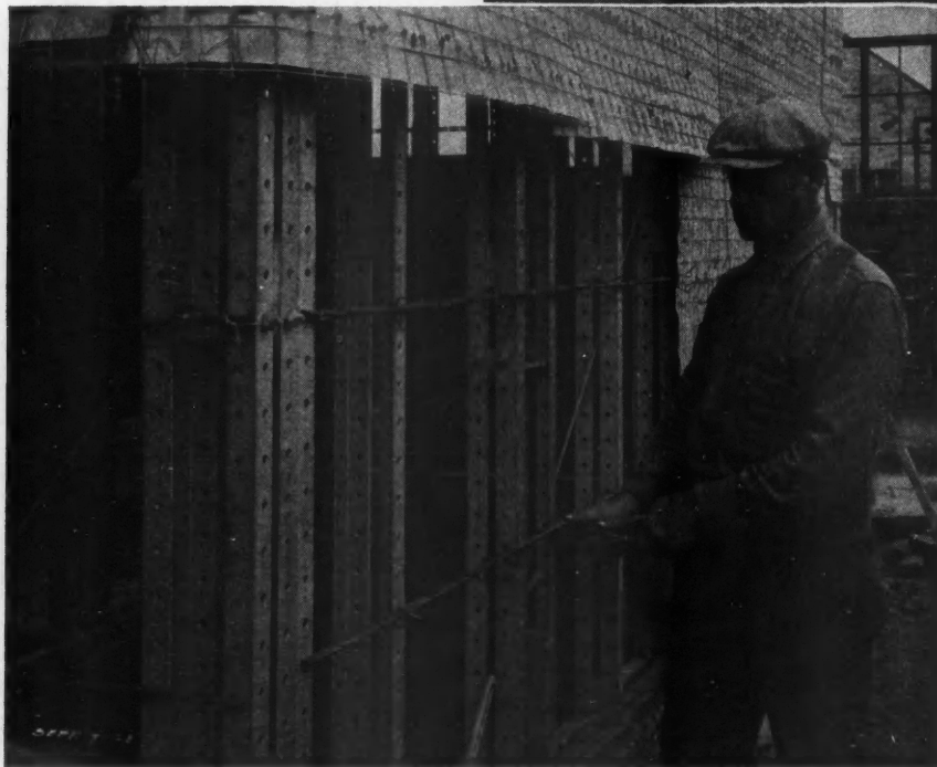
A Corner Detail of the Pittsburgh Steel Frame House, Showing Many Features of Construction. Note the corner post and typical studs; the perforation of all steel members, including the sill formed of two channels; also note the wind bracing wires and turn buckles. Illustration shows how attachment clips for plaster base (welded mesh reinforcing fabric with waterproof backing) is fastened to the studs at regular intervals.
