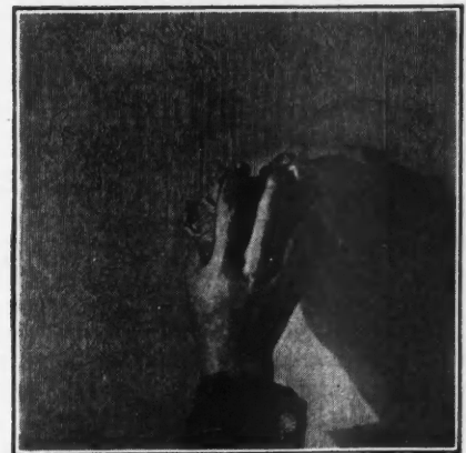
Producing the Crumpled Roll Effect Shown Above, Figure 2, in Plastic Paint with a Wad of Crumpled Newspaper.
