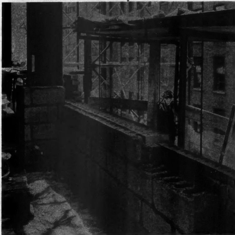
Exterior Wall of the 25-Story Integrity Trust Building Under Construction, Showing How Concrete Masonry Is Being Used for the First Time in Skyscraper Construction.
