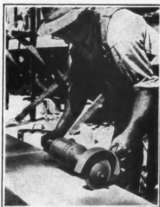
An electric carborundum saw, or an ordinary hand- or buck-saw, is used for breaking Indiana Limestone. One man keeps a number of stonemasons or bricklayers busy laying up stone.
