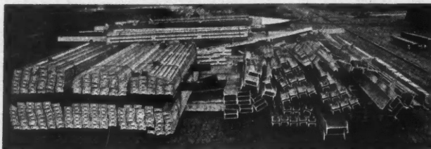
Here Is the Steel Frame for the Pittsburgh Demonstration House at the Mill, Bundled Ready for Shipment. Everything is complete, ready to bolt together on the job.
