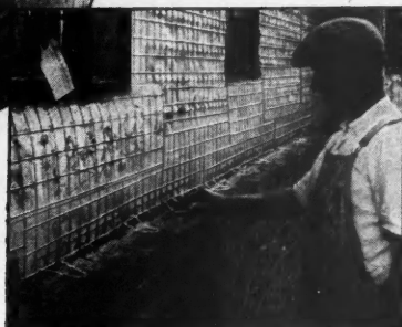
STEELTEX for Brick Facing provides a 1-inch reinforced cement slab, cast in place as the bricks are laid, forming a monolithic, moisture-proof wall of brick, steel and cement. Wall ties, hooked to the STEELTEX, are embedded in mortar.
