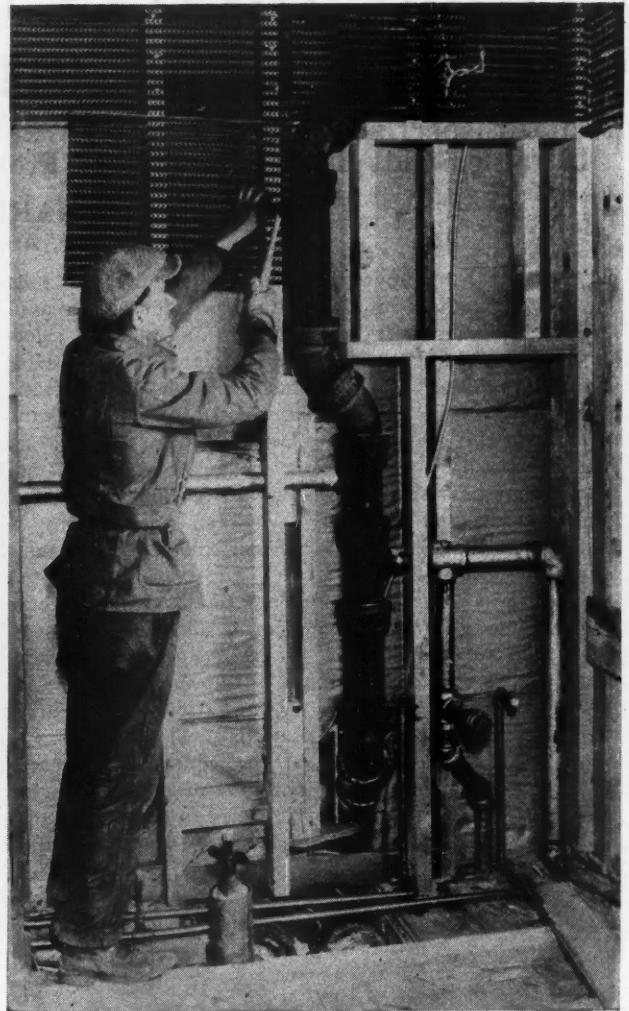
Quilt Insulation, the Proper Use of Brass Pipe and Metal Lath with Strong Framing Combined to Make the Concealed Portions of the Master Model Homes an "Honest Deal" on the Part of the Builder.
