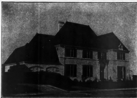
House at Stockton, California, John Upton Cloudsley, Architect. Roof of Cabot's Creosote Stained Shingles. Stucco walls finished with Cabot's DOUBLE WHITE. Insulated with Cabot's Quilt.
