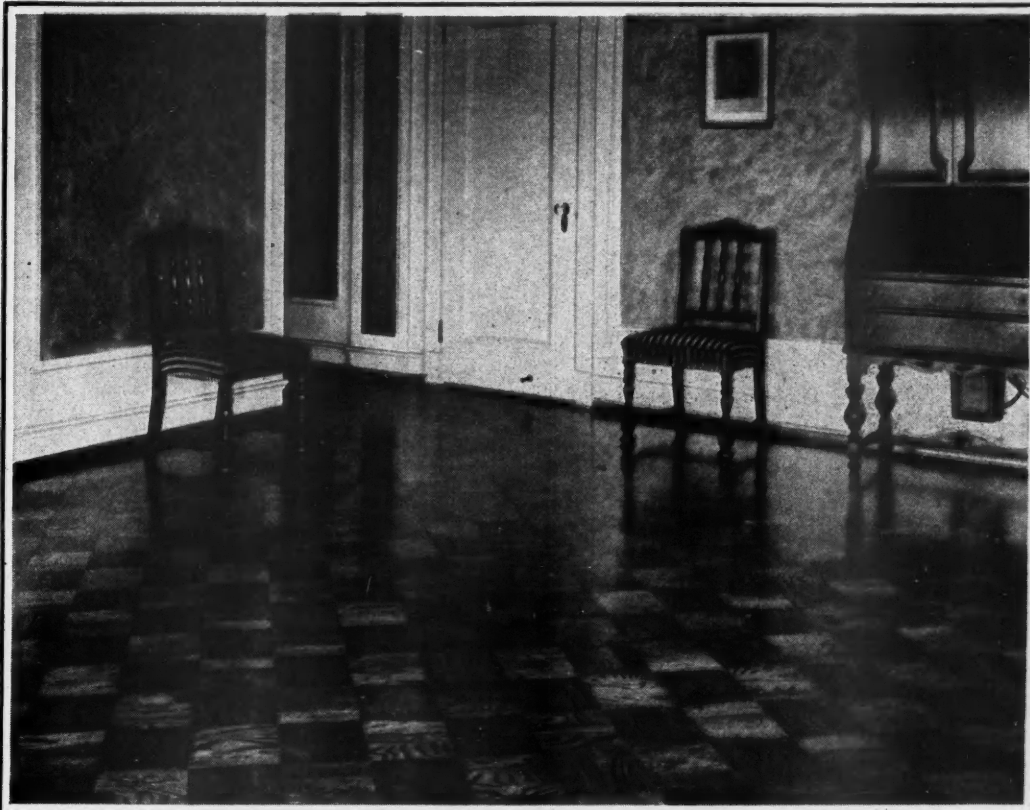
A complete unit of four flooring strips, splined together
