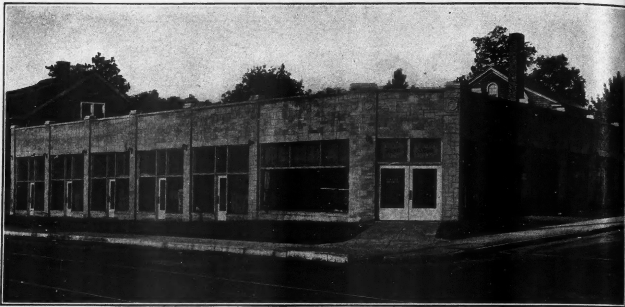
Carter Block, Indianapolis. E. H. Dalby, Designer and Contractor. An example of a moderate-priced store building built of Variegated Indiana Limestone Random Ashlar.
