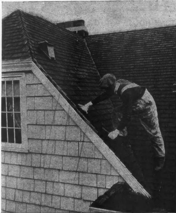
In Order That Old Shingles Shall Not Show at the Gables, Cut a Bare Strip Along the Edges and Nail on a One by Two-Inch Batten Which Will Look Like Part of the Trim.
