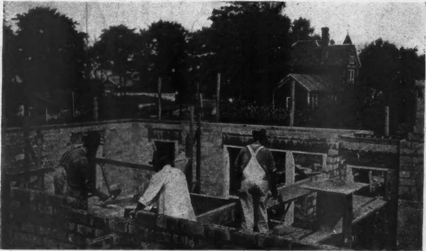
Concrete Tile Build Up Swiftly and Accurately Into All Types of Walls, Bearing or Otherwise. Both partition and main walls of the house under way here are being built of the small, strong and easily handled concrete tile.
