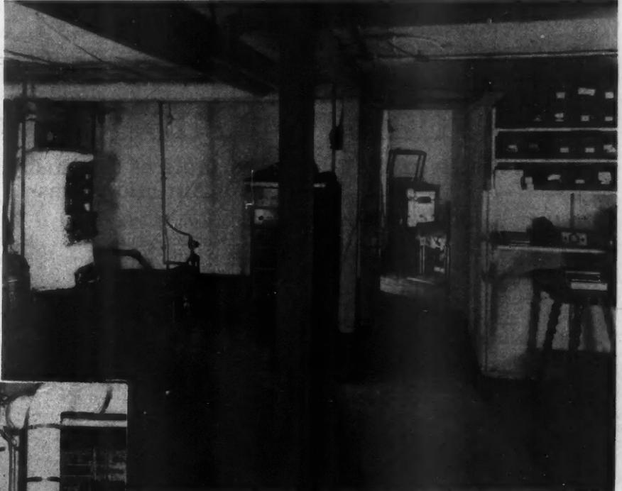
A Clean, Comfortable Basement Fitted Up for Living and Bed Rooms. The heating plant with automatic oil burner and the hot water heater show at the left of the picture.
