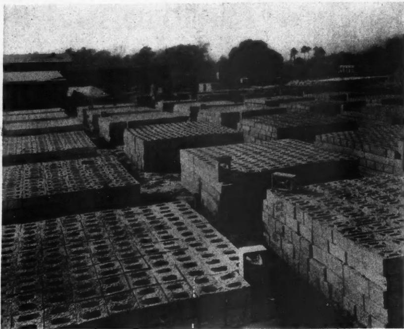
Thousands of Concrete Tile Were Manufactured, Cured in Steaming Curing Chambers, and Stacked on the Grounds in Advance of Their Use so That Well Cured Tile Were Assured for All Portions of the Structure.
