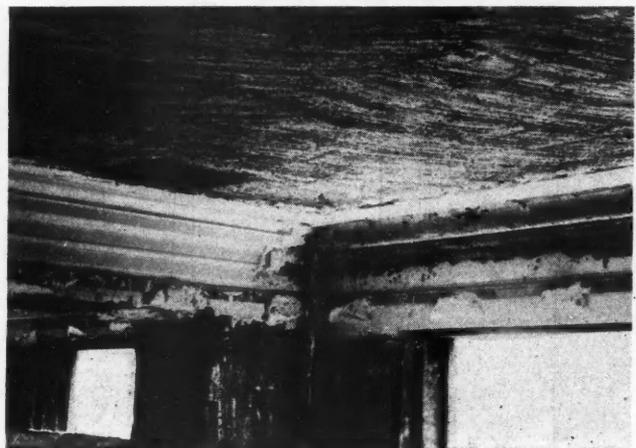
Fig. 3. The Portion of the Cornice at the Right Is Seen as Produced by the Rough Template While That at Left Is Finished.
