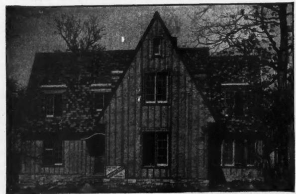
House near Chicago, showing its "underclothing" of Cabot's Quilt, with jarring strips over the Quilt, on which the outside finish is laid. Roof also insulated. Leon E. Stanhope, Architect, Chicago.
