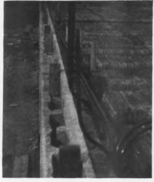
End Board and Floor Forms in Position for Casting the Beam and Arch Floor.
