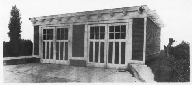
THE SEALY GARAGE—Here is a design with a nearly flat roof, the slope being only sufficient for draining, which has been given an added degree of individuality by projecting rafters which are suggestive of the pergola.
