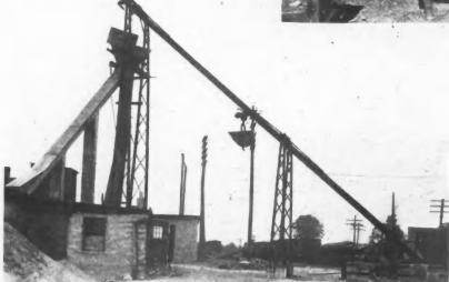
Bucket Conveyor and Gravity Chute Handling Aggregate at the Plant of the Steward-Silver Company, Columbus, Ohio. This method shows efficiency in some plants.
