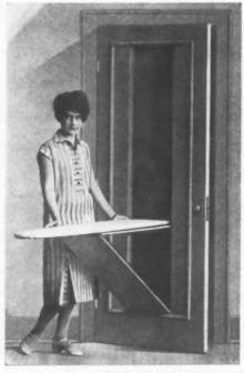
This Ironing Board, Built Into a Door of Standard Size, Is Absolutely Out of the Way and Out of Sight When not in Use and Among Other Uses Makes an Ironing Board Available in Any Bed Room.
