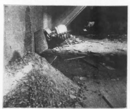
Not All Fire Hazards Are the Result of Faulty Construction. This loft over a theater auditorium, with ashes, rags, paper and rubbish littered over the floor is a serious fire hazard.
