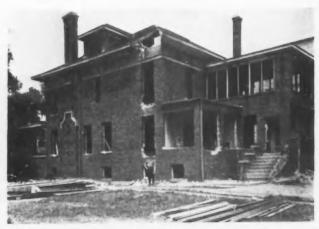
The Start of the Job, Showing the Building "Gutted Out," All Sash Frames and Interior Finish Removed and the Roof Ready to Be Taken Off.
