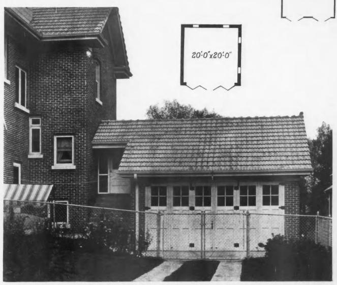
THE SECOR GARAGE—Not only does this garage follow the style of its house, but is attached to it with the appearance of being an actual part of the structure. It is, however, separated from the house structure by a solid wall, which is a requirement under the fire regulations of certain communities.
