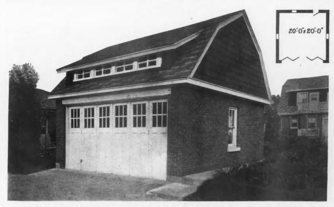
THE SAINT CLAIR GARAGE—Another attractive design, for the larger brick residence, is of brick and shingle construction with a composition shingle used on the roof. It is of a size to provide for housing of two cars and its plentiful lighting will be found a great convenience.
