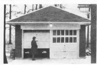
Doors Which Slide Up Into an Overhead Position Are Always Out of the Way, Are Never Damaged by Being Banged by the Wind and Are Not Injured by Rain, Snow or Ice.
