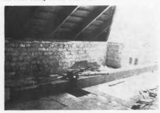
This Is Probably the Most Satisfactory Method of Holding the Timber for Supporting the Hoisting Pulley.
