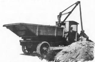
A Derrick Which Can Be Mounted on Any Truck Chassis Is Made in Two Sizes, 1,000 and 1,500 Pounds Capacity, and Is Adapted to Hoisting, Loading and Digging.
