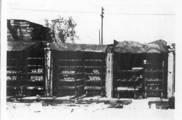
The Elimination of Waste Space in Curing Tunnels Makes a Direct Saving in the Amount of Steam Heat Required. These tunnels at the tile plant of the Superior Sand & Gravel Company, Detroit, Mich., are just long enough and high nough to admit the loaded cars.
