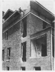
Pulleys Suspended from a Beam to Lower Steam Radiators, and Plumbing Pixtures to the Salvage Truck.
