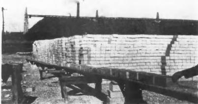
View at the Delta Brick & Tile Company's Plant, Detroit, Mich., Showing Belt Conveyor in Use Bringing Concrete Blocks to the Storage Yard.
