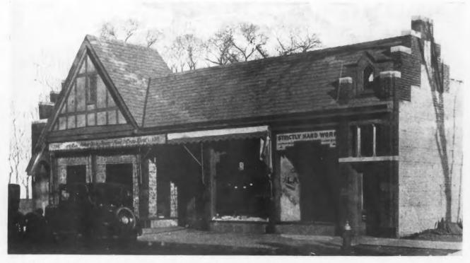
Small Store Buildings of This Type Usually Require No Basements and Small Cabinet or Hot Water Heaters in Each Store Will Supply Adequate and Economical Heating.
