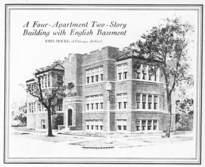
Here is a high-grade, side entrance apartment building for a 50-foot lot, with two four-room apartments on each floor. All rooms are exceptionally well lighted. The heating plant is placed at the rear of the basement space, leaving the front apartment for very desirable living quarters.
