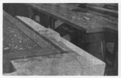
A Concrete Floor Built Up to Give It a Thickness Equal to That of the Water Table Course on the Outside. Notice the air space between the concrete floor and the masonry wall.
