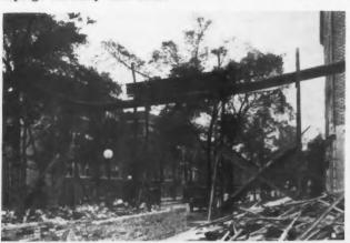
A Runway from the Second Floor Is Provided for Depositing the Bricks, Which Have Been Cleaned, in Piles.
