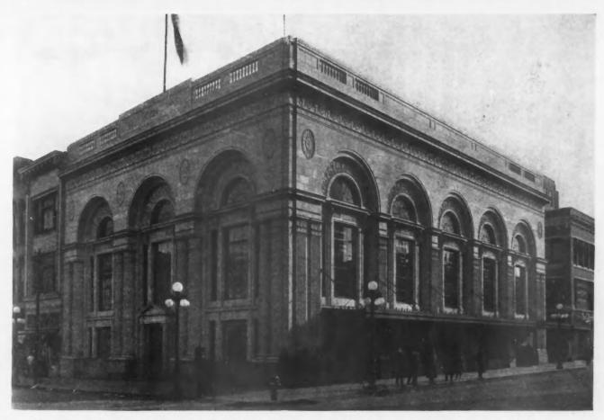
Kalamazoo Trust and Savings Bank Building, Kalamazoo, Mich., Weary and Alford, Chicago, Architects. The building is of reinforced concrete and has two large steel girders which span the banking room. An economic feature of this building is that space has been provided for a number of high class shops, and revenue from these leases is said to be sufficient to carry the investment in the entire building.
