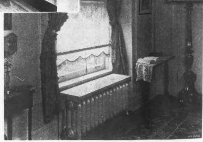
Radiator Furniture Not Only Improves the Appearance of the Room but Also Improves the Heating Efficiency as Well. A large quantity of water can be evaporated from the pan under the ornamental seat assuring healthful moisture in the home.
