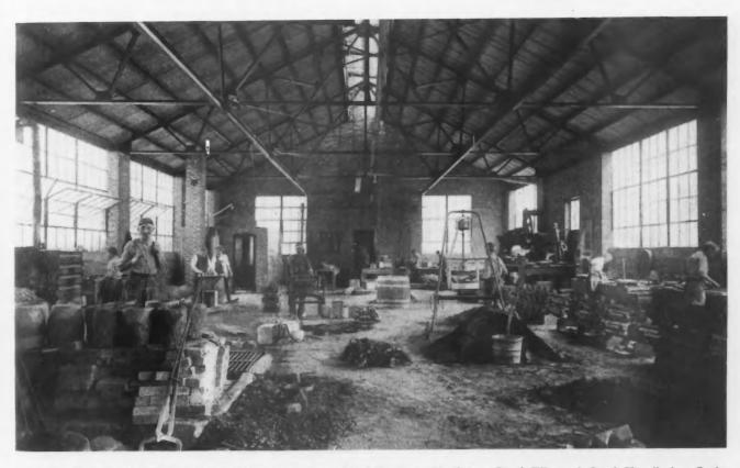
This Is a Typical Industrial Building with Steel Roof Trusses, Skylights, Roof Tile and Steel Ventilating Sash. All weights suspended from roof trusses, such as the conveyors shown, must be added to the roof load and stated to the truss designer.
