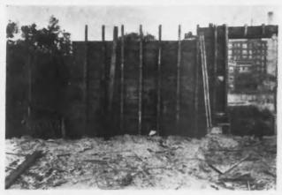
Sheathing Can Be Stripped from the Studs Without Damage by Knocking It Off with the Front of a Pick.
