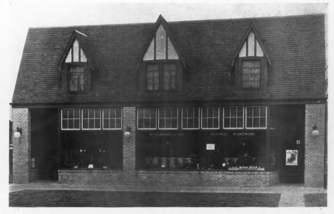
This Lot Being but Fifty Feet in Depth, Small Stock Rooms Are Provided on the Attic Floor Above. Reference to the plan shows that disappearing stairways conserve profitable space in the stores at a minimum cost.
