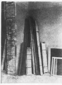
The Casing, Jamb and Head Moulding for Each Door Should Be Carefully Removed and Tied in One Bundle.
