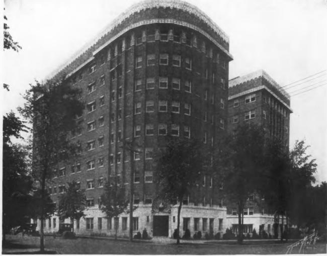
The Two Wings of This Fine Apartment Hotel Are Connected Only on the Ground Foor and This Liberal Light Court Allows Full Daylight to Each Room. Full use is made of the disappearing bed feature and beds of this type only are used throughout the building.
