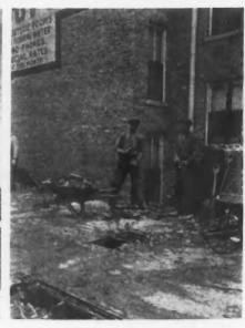
A Small Double Bladed Ax Is Used to Clean Bricks and the Rubbish Drops to the Floor Below Through the Hole in Front of the Men.
