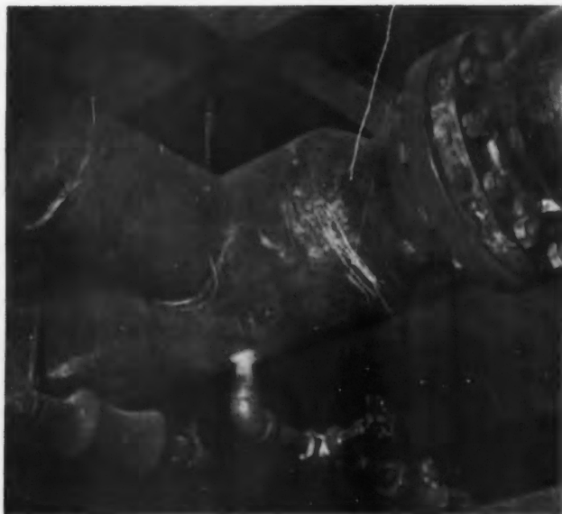
It Is When Making Connections Like This That the Advantages of Welded Plumbing Installation Are Most Apparent. These three joints would be both difficult and expensive if screw connections were used.
