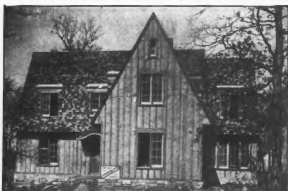
House near Chicago, showing its "underclothing" of Cabot's Quilt, with "urring strips over the Quilt, on which the outside finish is laid. Roof also insulated. Leon E. Stanhope, Architect, Chicago
