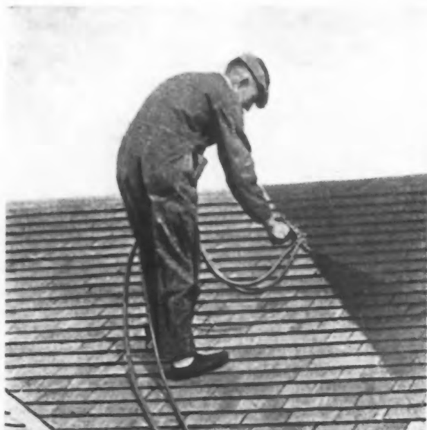
Large Roof Areas Can Be Quickly, Economically and Thoroughly Painted with Mechanical Equipment and Their Life Is Greatly Increased by Paint.
