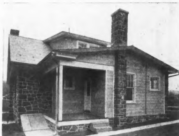
Showing Application of Linabestos Clapboard
