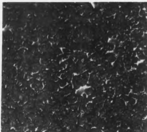
Interesting Wall Finishes Produced with a Spray Gun and Plastic Paint. A wide range of textures from a light sandpaper finish to a heavy stucco effect can be secured by this method.
