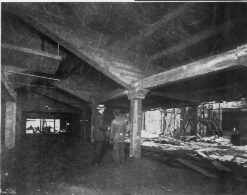
Another Detail of Construction Showing How the Balcony Is Supported by Reinforced Concrete Cantilever Beams, with an Overhang of 18 Feet Which Obviates the Necessity of Supporting Columns Beneath.
