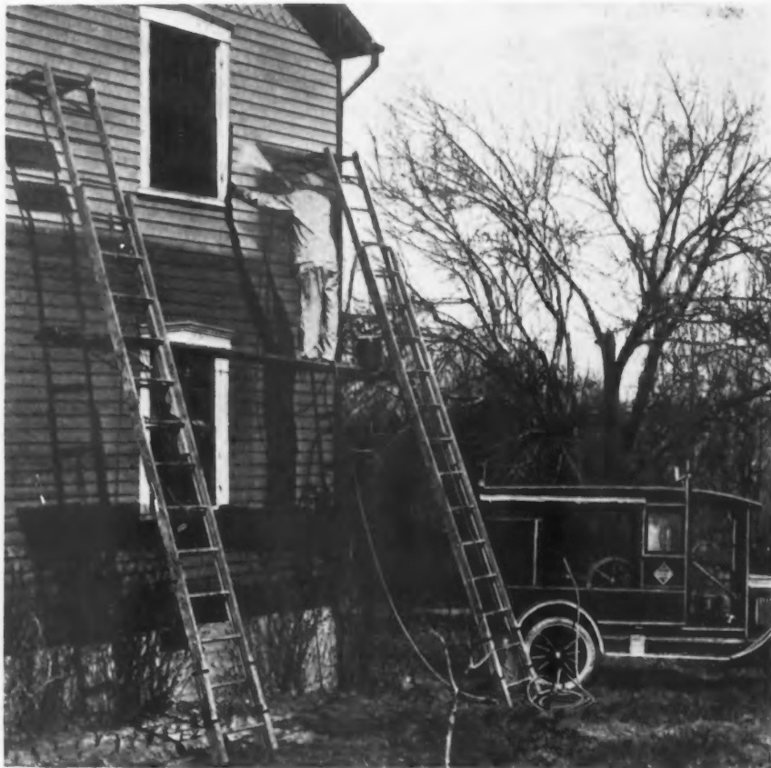
By the Mechanical Method, It Is a Matter of Minutes to Paint the Side of a House and There Is a Big Saving in Cost.
