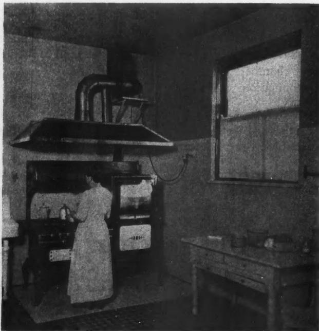
This Ventilator Is Built Into the Range Flue. Power is taken from a light socket or especial wiring can be provided.
