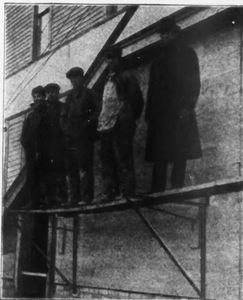
The "Safety First" Possibilities of the Steel Scaffold Bracket Are Evident from This Illustration.
