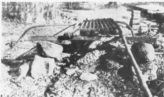
Simple and Inexpensive Device for Heating Mixing Water Recommended Where Steam Boiler or Other Source of Hot Water Is Not Available.
