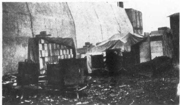
Tarpaulins and Salamanders Used in Heating Concrete Block to Be Laid During Cold Weather. Warm block lay easily and rapidly and protect the mortar against freezing.
