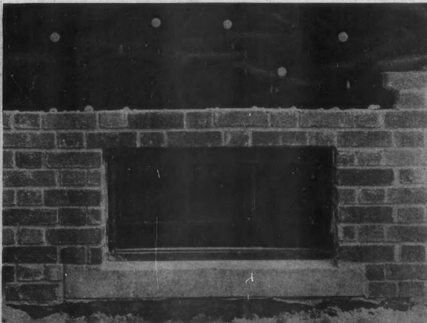
Detail of Good Brick Veneer Construction. Note tar paper fastened with big headed tacks to sheathing boards. A 4-inch face brick wall is tied to the wood frame.
