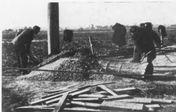
Stove for Heating Sand and Gravel Made of Several Sections of Discarded Smokestack.
