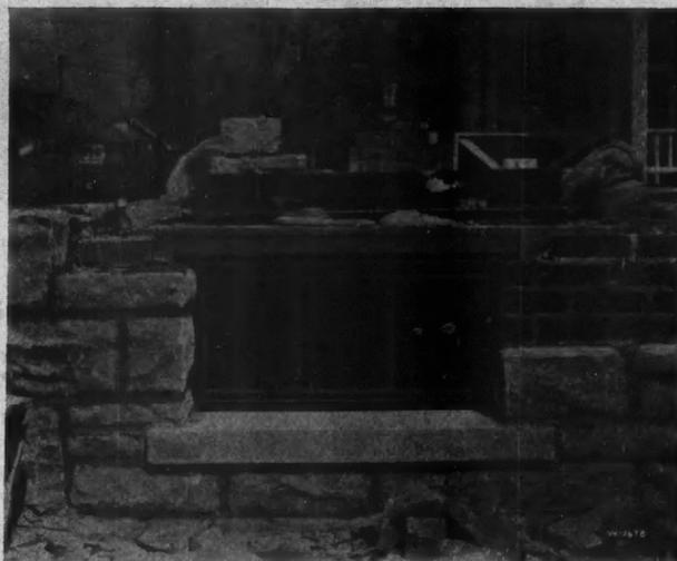
Closeup of Steel Cellar Sash in Stone and Brick Wall.
