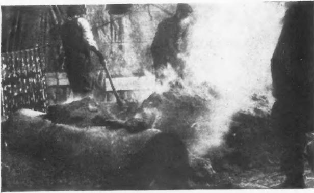
Iron Pipe Sections Being Used as Heaters for Sand and Gravel on the Work of the New Chicago Union Station.
