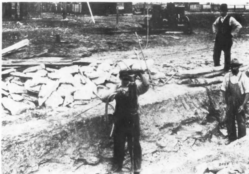
Power Operated Air Compressor Rig Successfully Drilling in Hard Rock at St. Paul, Minn.
