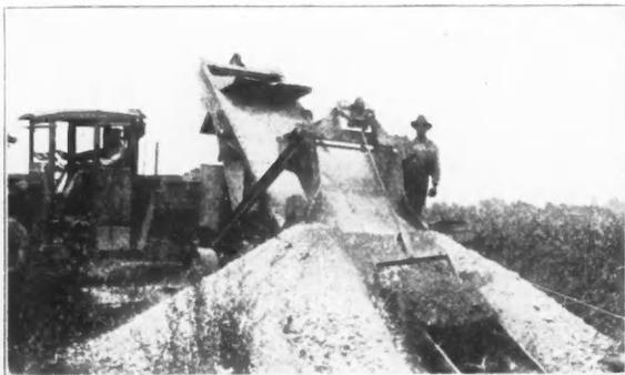
Fig. 2. Excavator and Loader on Gravel Pit Work.
