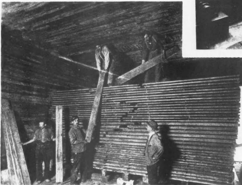
This Is How the Freshly Cut Lumber Is Piled for Treatment by Super-Oxygen in a French Kiln-Drying Plant.
