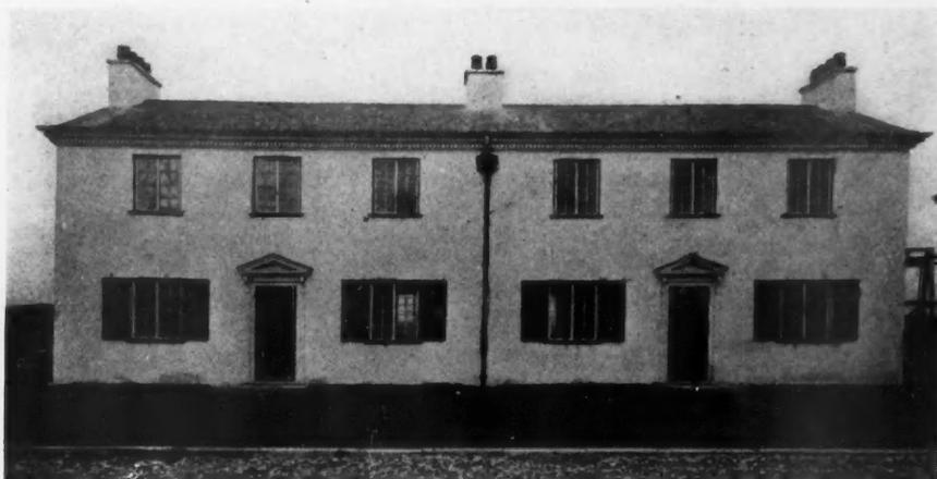
Steel Framed House Finished and Ready for Occupancy. This Is the So-called Semi-Detached House, Containing Four Apartments. The Floors Are Concrete with Oak Covering.
