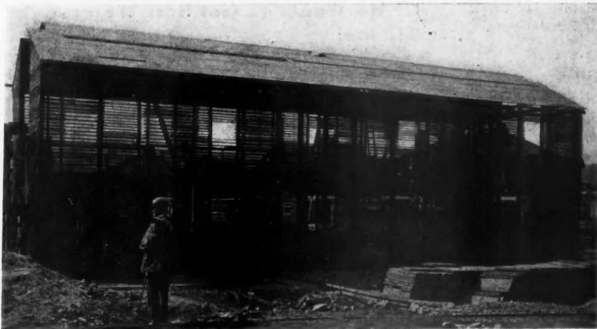
Steel Framing Covered with Metal Lath and Ready to Receive Stucco Covering. The Roof Is Boarded with Sheathing. The Partitions in This House Are Made of Cement Slabs.
