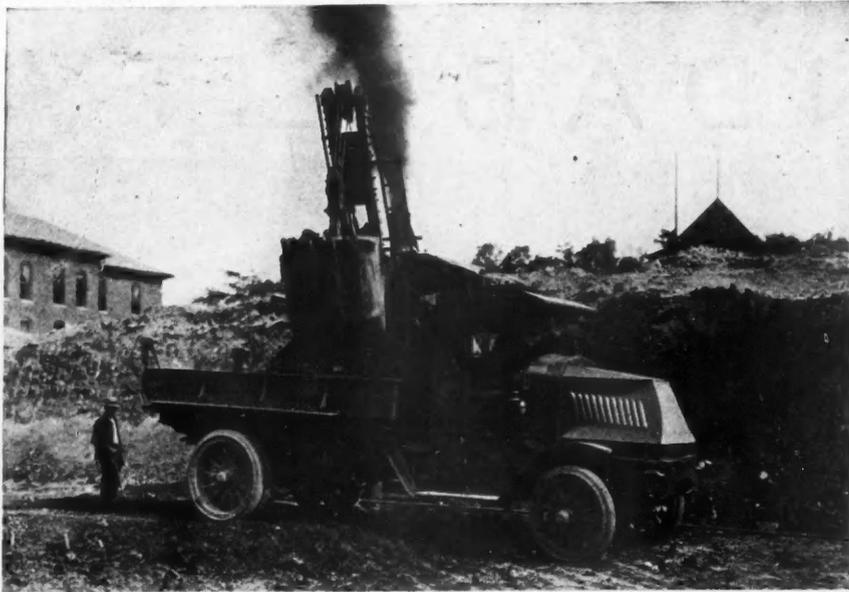
Dempster Construction Company Found This 3 1/2-Ton "Mack" Truck Could Keep Up with a Steam Shovel Despite the Heavy Grade. It Also Used a Short Cut Which Was Impassable for Horses.
