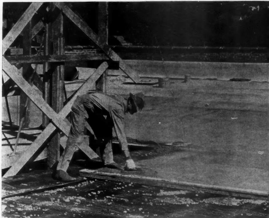
Troweling Concrete Slab in Steel Lumber Flat Roof Construction.
