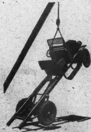
Duplex Limited lifted clear of ground by wire around windshield frame. Strength of cowl means safety and less vibration.
