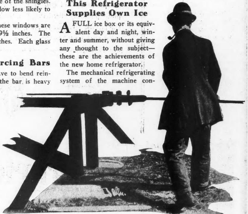
Bar Bending Machine for Bending Reinforcing Rods on the Job. It Is Light and Can Be Carried Around from Place to Place Without Trouble.
