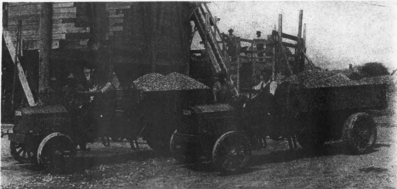
The Rowe Contracting Co., Boston, Mass., is a busy firm and for that reason maintain a fleet of 5-Ton "Packards" like the pair shown above. These trucks have just been filled up from hoppers and are starting out to the job which is quite a distance away. The dump bodies make unloading a matter of minutes.
