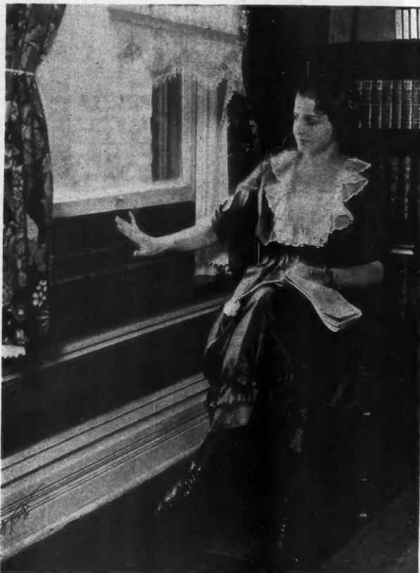
The Fresh Air Enters the Room But Is Deflected Upward so There Is no Trace of Draft When a Person Sits Next to the Window. The Arrangement Also Prevents Rain from Coming Thru.
