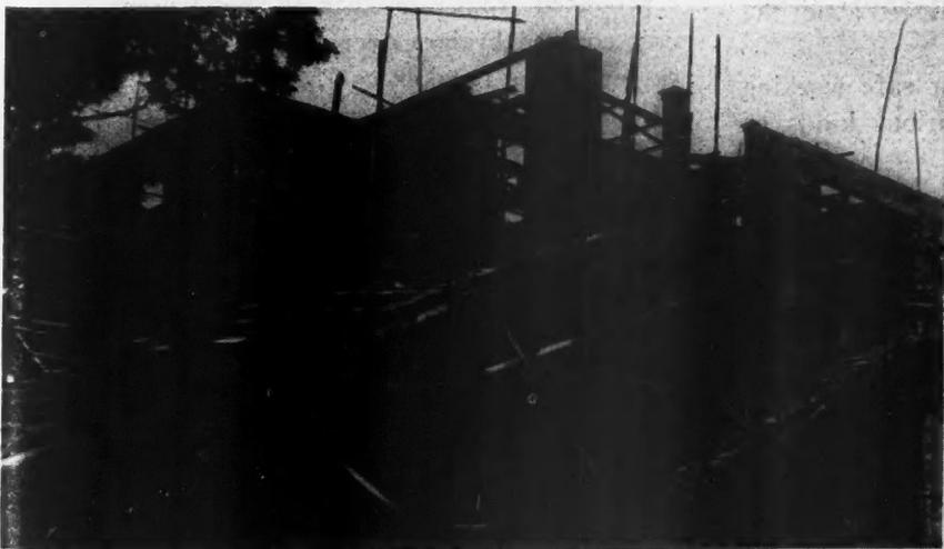
Home of M. A. Cheek, Also of the Firestone Rubber Co., Under Construction Near Singapore. Note the Scaffolding and Runway of Bamboo. The Runway Replaces the Ladders and Hoists Commonly Used in the United States.
