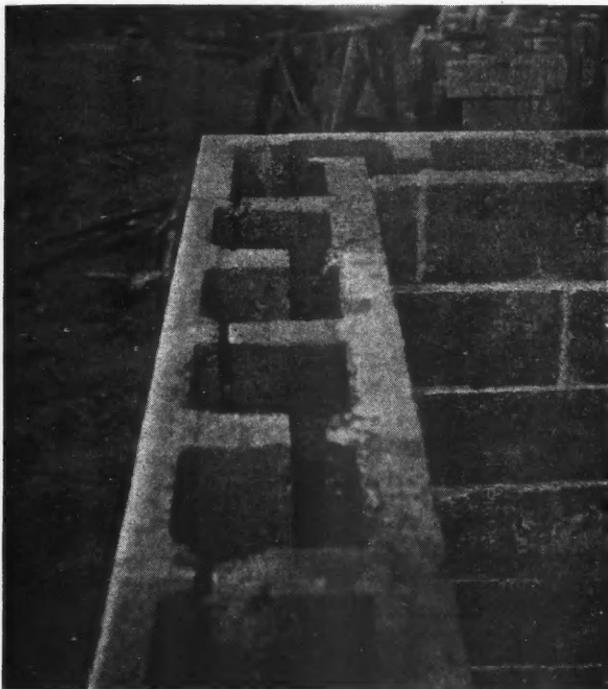
Figure 8. System Illustrating Use of Special Length Corner Block.
