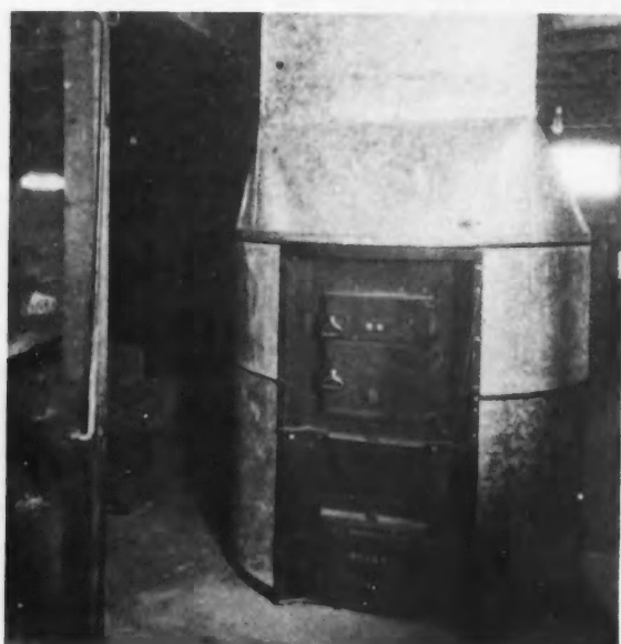
Composite Photograph, Showing the Pipeless Furnace in the Basement and the Double-Faced Register Above It. Note the Location of the Register in the Opening Between Living and Dining Rooms. The Single Register Supplies Heat to Both Lower and Upper Floors of a Medium-Sized Home, but It Does Not Heat the Cellar.
