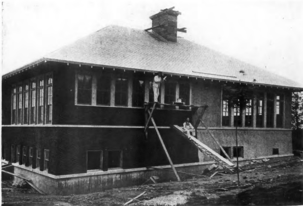
Reinforced Plastering Fabric on a Small School Building, Part of Which Has Been Covered by Stucco. The Backing Gives as the Stucco Is Forced Against It, the Plaster Sinking in and Keying on the Reinforcing Wires.
