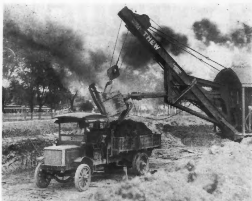
A "Federal" Truck Receiving Dirt from a Steam Shovel Excavating for a Big Building. Trucks Take Heavy Loads and Carry Them Up the Grade from the Excavation Easily.
