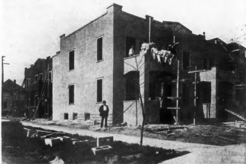
Workmen Finishing the Stucco Walls of an Apartment Building. The Base Is Reinforced Fabric. The Picture Shows the Excellent Surface Secured.
