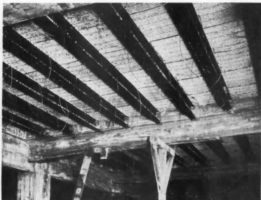
Metal Lumber and Metal Lath Floor Construction, Ready for the Suspended Ceiling.
