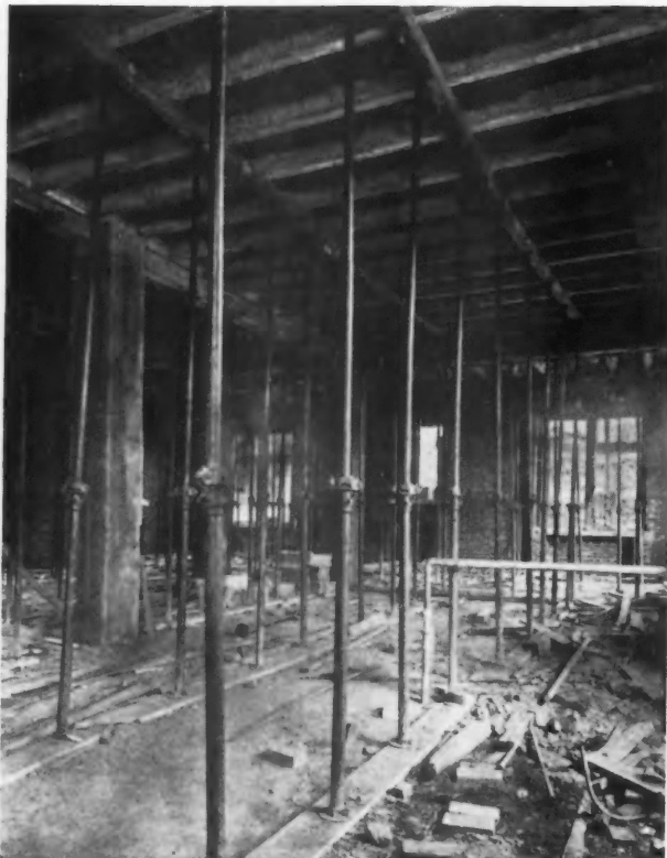
Floors Held Up by Joint Panel Jacks That Take a 4-Inch Timber. The Jacks Make the Job of Shoring an Easy One and Save Much Time and Labor.
