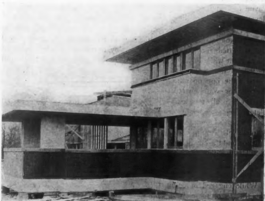
Sun Parlor of Residence, Showing How Square Mesh Fabric Was Applied Over Furring Strips 16 Inches on Centers.
