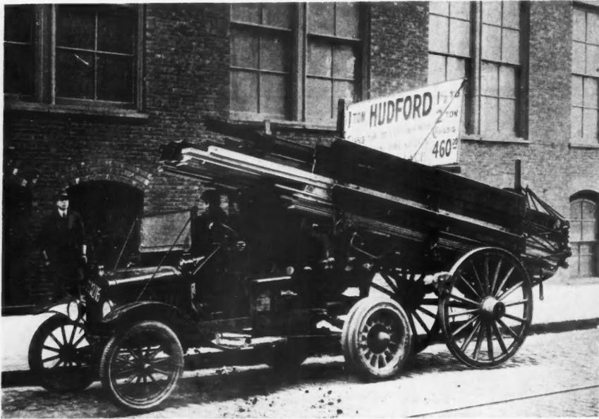
A Philadelphia Contractor Has a "Martin" Trailer, Specially Constructed to Haul Materials to the Job.
