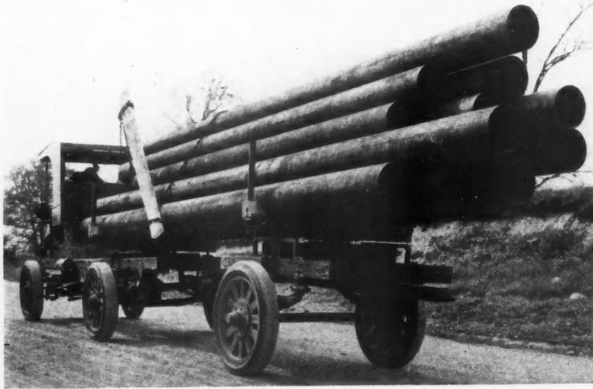
How Long Pipe May Be Hauled by the Use of Semi-Trailer in Connection with a Motor Truck Is Here Shown. The Rear Wheels of This "Miami" Trailer Are Supporting the Bulk of the Load, and Extending the Wheel Base of the Vehicle, so That There Is No Danger in Turning Street Corners.
