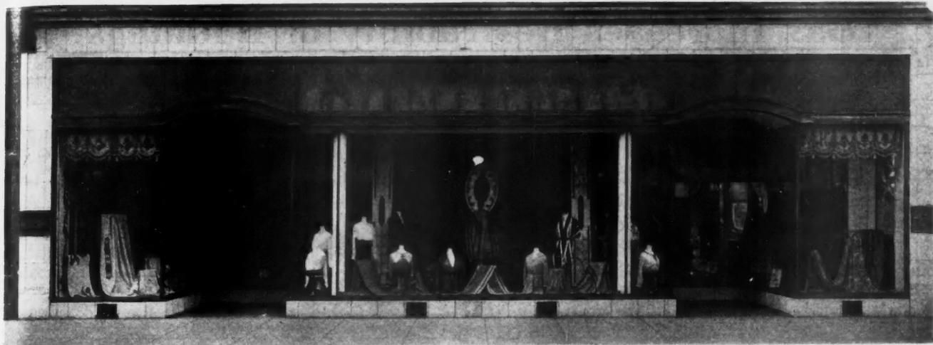
Another Type of Modern Store Front Construction. Entrances at Each Side Give Patrons of the Store a Front and Rear View of the Central Window, and Also Allow for Good Displays of Merchandise on Either Side. The Terra Cotta Trim Adds to the Attractiveness of This Front.
