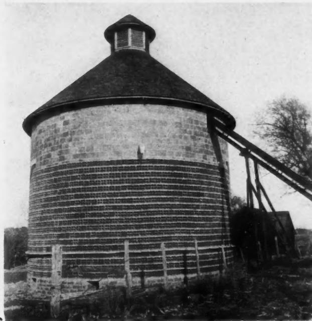
Circular Corn Crib and Granary of Vitrified Clay Tile. The Tile for the Lower, or Crib, Section Have Pierced Holes for Ventilator.
