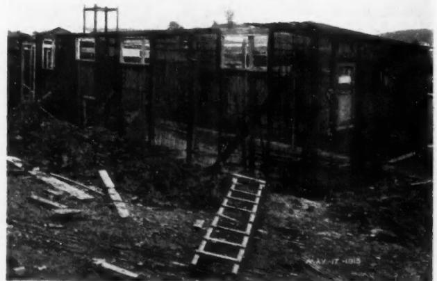
Hog House Under Construction, Showing No. 27 Gauge Trussed Metal Lath in Place for the 3-Inch Side Walls.
