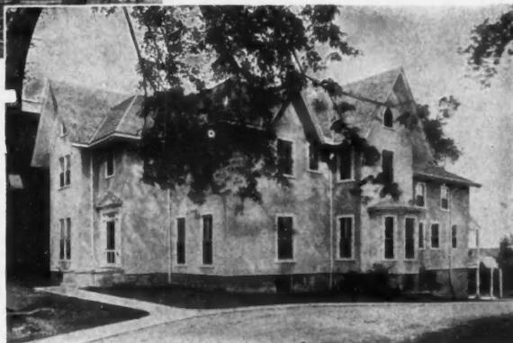
The Same House Improved with Metal Lath and Stucco Exterior Put on Over the Old Boards.
