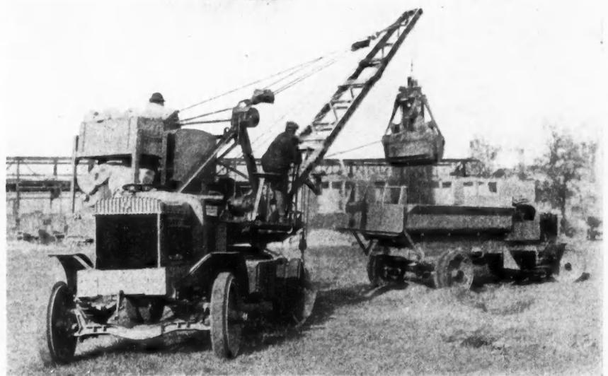
The "Winther" Truck and Mounted Hoist Delivering the Clam-Shell's Load to Another Truck.
